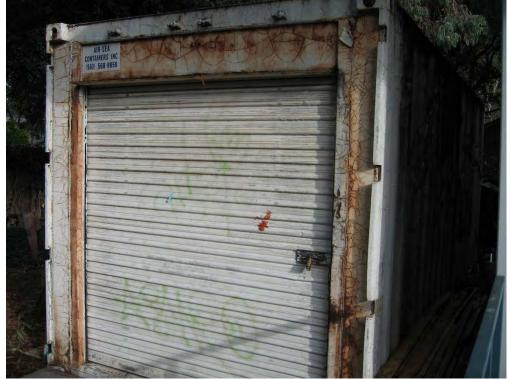
Photograph 21: Paint cracking on the outside of a storage container behind the gym
