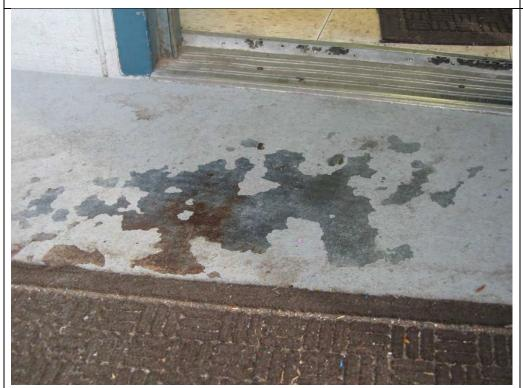
Photograph 19: Peeling paint on the metal walkway going into the gym
