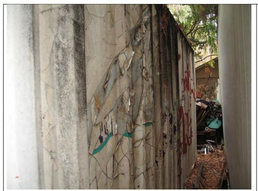
Photograph 22: Paint peeling on the outside of a storage container behind the gym
