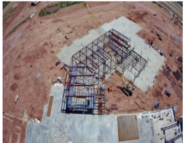
Area A & E Steel Erection Ongoing
