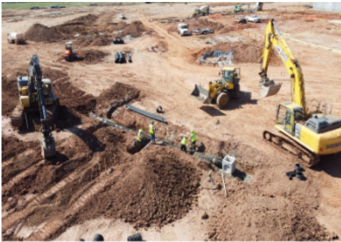
Storm Sewer ongoing East Side
