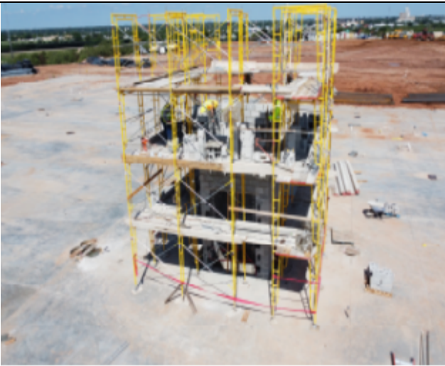
CMU Elevator Shaft Area F
