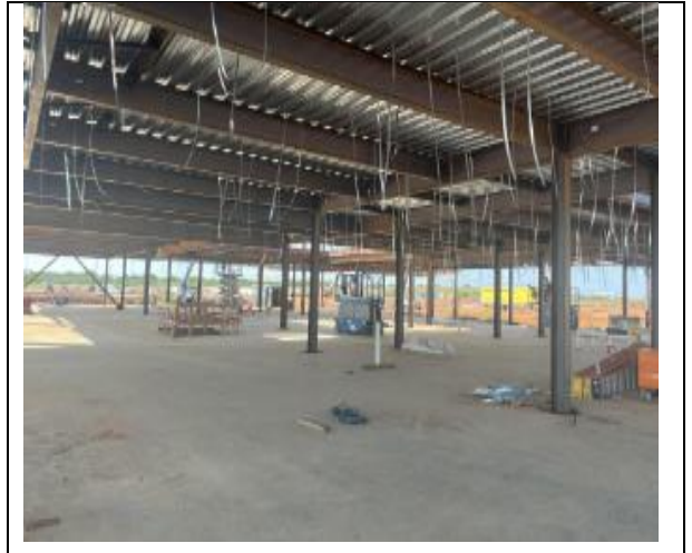
Area A & E Overhead Hangers and Straps
