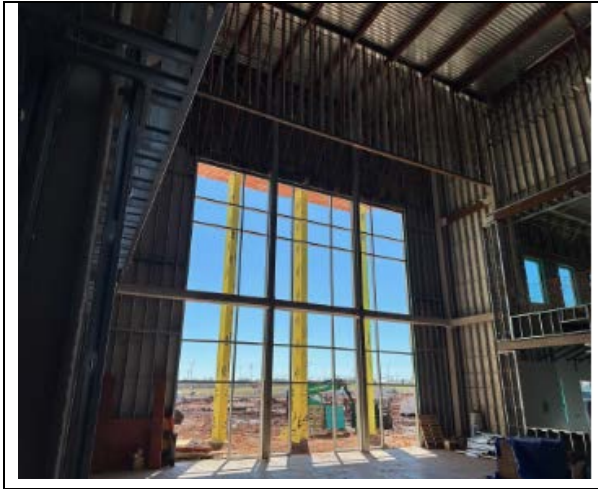
Area B Curtainwall
