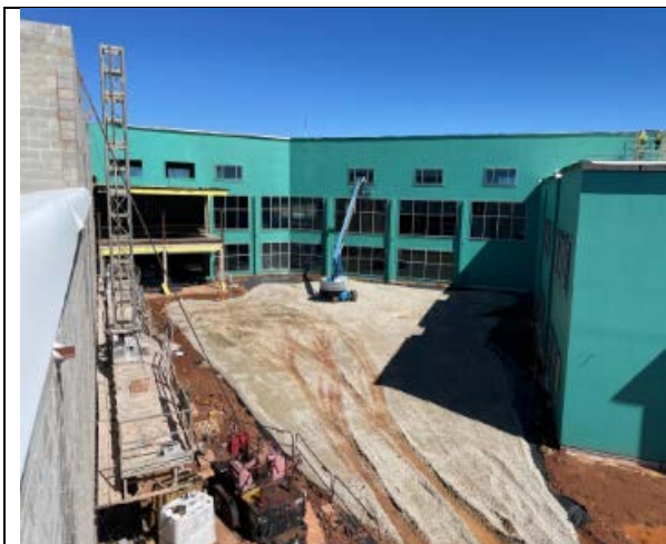
Courtyard Stone subbase
