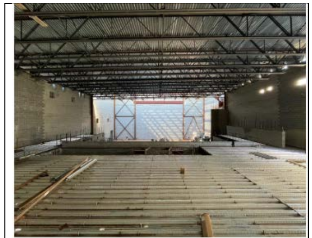
Area V Floor and roof deck
