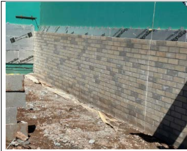
Area A Brick Veneer started
