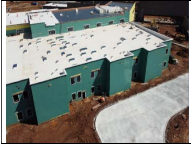
Exterior Sheathing/Windows Areas C & D
