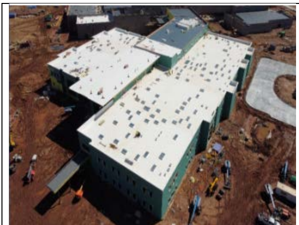
Roofing Areas B & E
