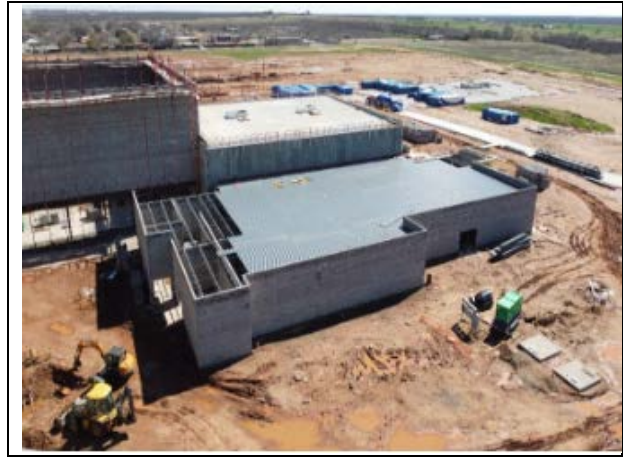
Area K Steel Erection
