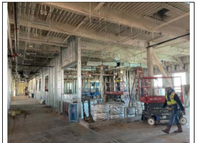
Area S MEP Overhead and Wall Framing
