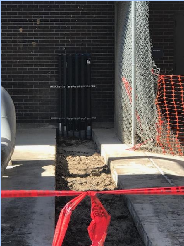
CTE electrical infrastructure connection to the main school plant.
