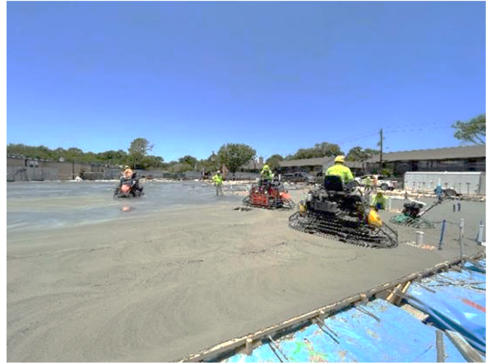
Power trowlers stabilizing and smoothing slab
