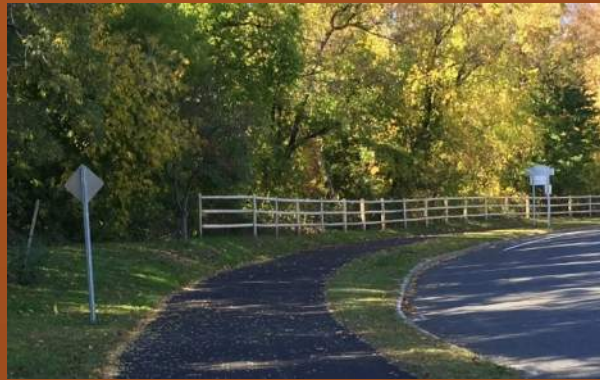
Phase 2 – Near Quaker Lane South
