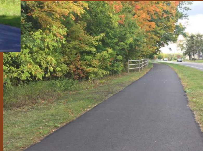
Phase 2 – Along Trout Brook Drive
