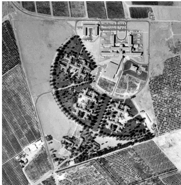
Figure 11. Aerial photograph of the East Campus, 1960
