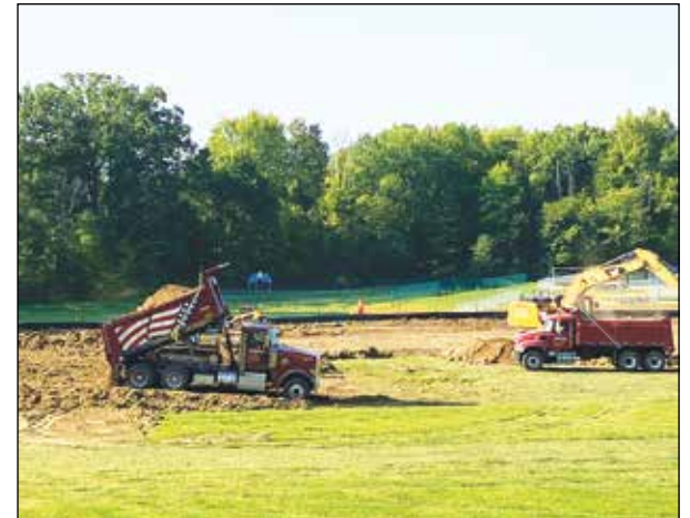
Images of the new baseball field being constructed.
