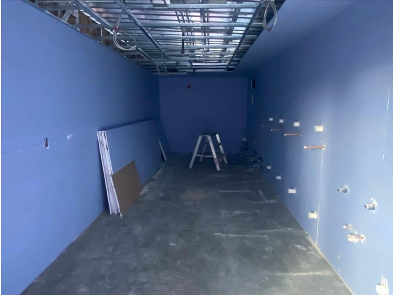
Sheetrock installation in the Grandstand bathrooms began this week
