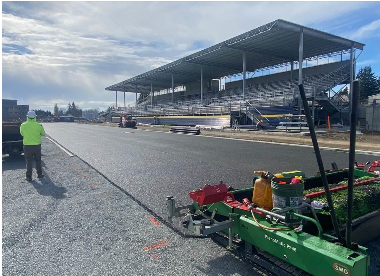
Installation of the rubberized layer that will sit below the astroturf
