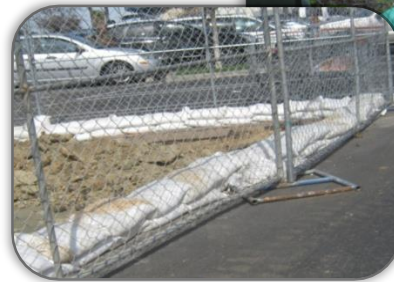
Gravel Bag Berm
