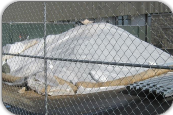
Use fiber rolls and gravel bags to protect perimeter and hold plastic in place
