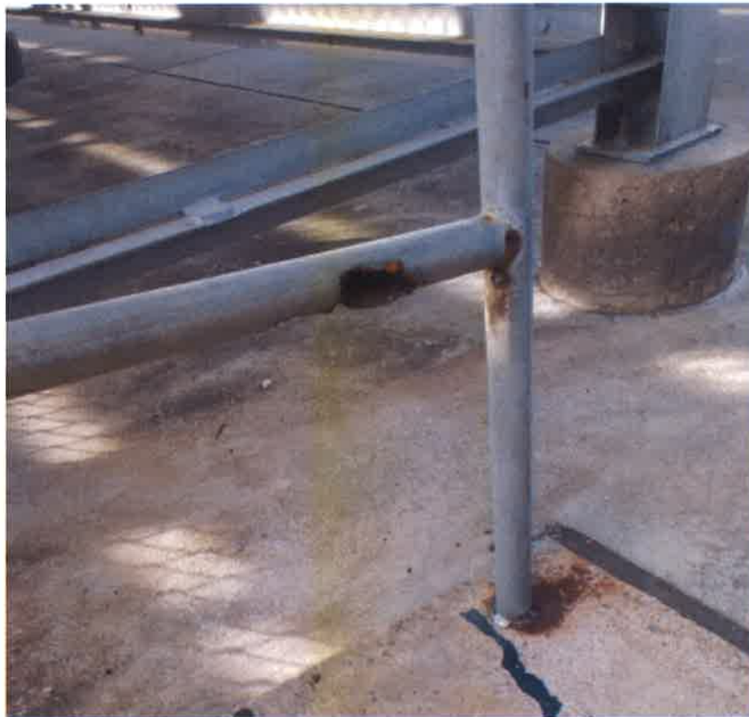
Photo 57: Deteriorated Handrail
