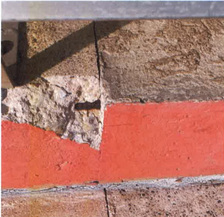
Photo 42: Spalling of Concrete with Exposed Rebar on Step "U"
