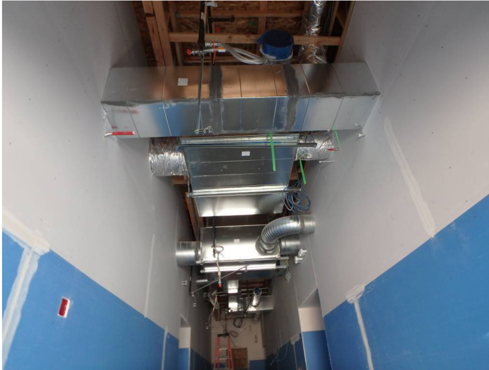
Ducting cross the main corridor
