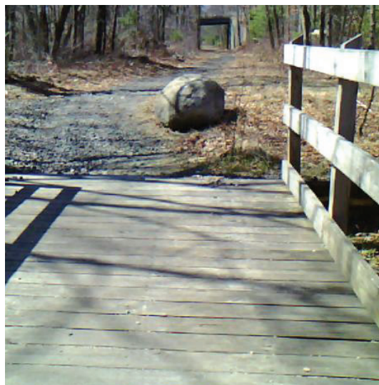
Bridge between Sand Dam Rd. and Lowell Davis Rd.
