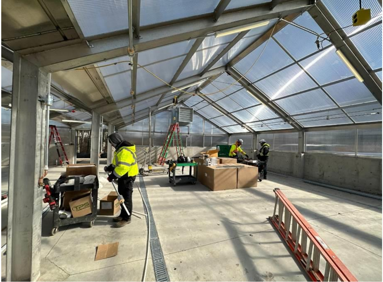
Crews making good progress on the Greenhouse
