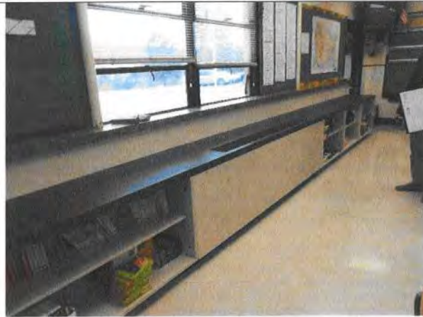
Casework: Built-in metal and laminate casework in classrooms in the original and 1989 construction is in good to fair condition.
