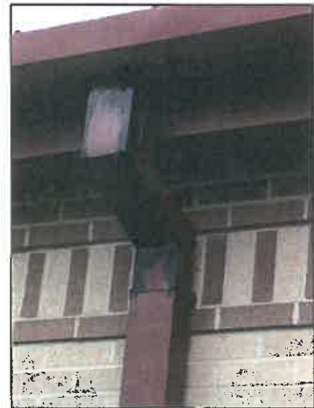
Biglerville ES Roof/Gutter System
