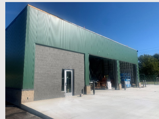
Maintenance Building (at Groves)
