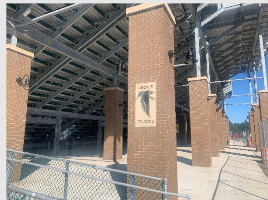
Piers Under Bleachers at GHS
