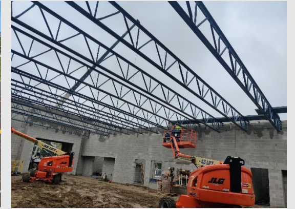
Steel Joists at Pierce
