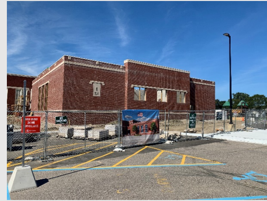
Addition at Pierce Elementary
