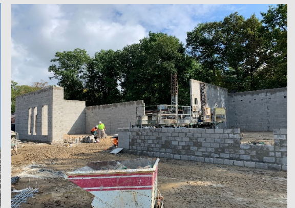
Addition at BATP (formerly Annex)
