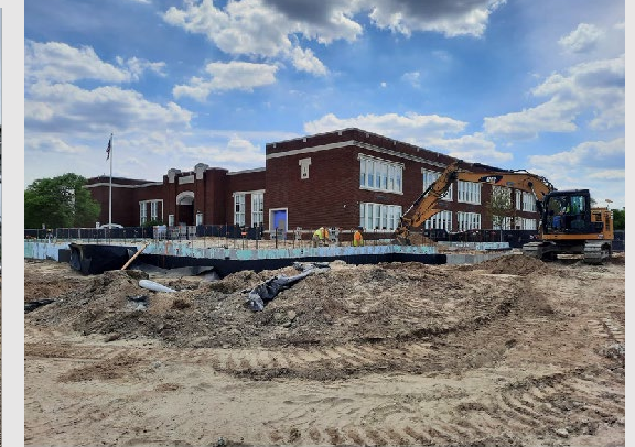
Addition at Pierce Elementary
