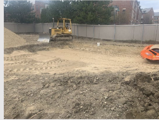
Building Pad at Transportation
