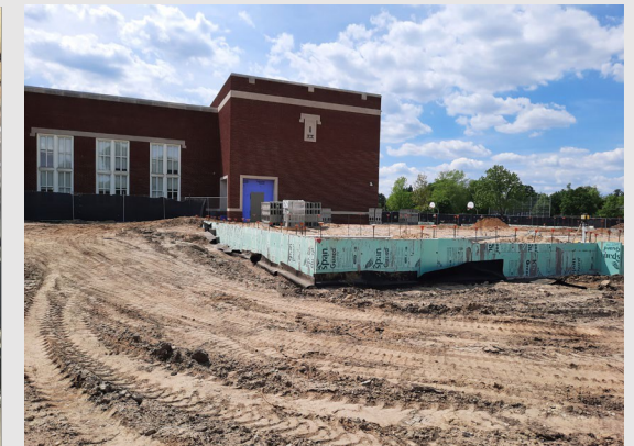
Addition at Pierce Elementary
