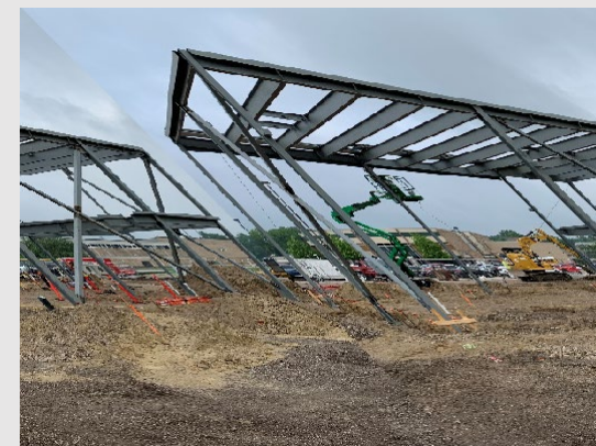
Maintenance Building (at Groves)
