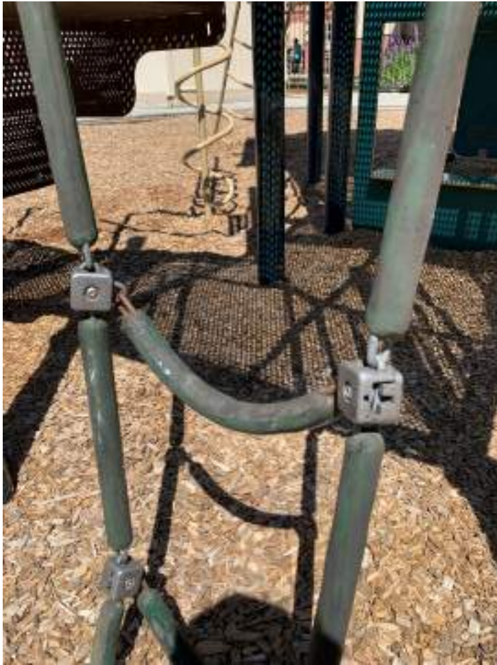
Deteriorating and corroded tensile climber. Pinch and laceration concern.
