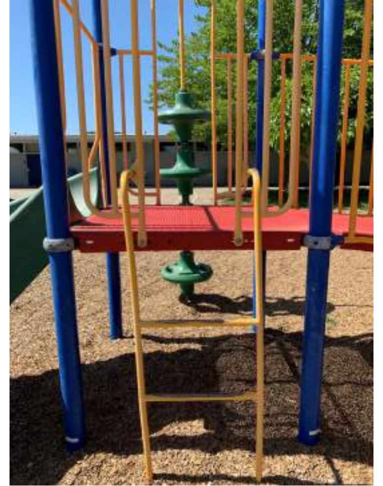
Bent/warped ladder.
