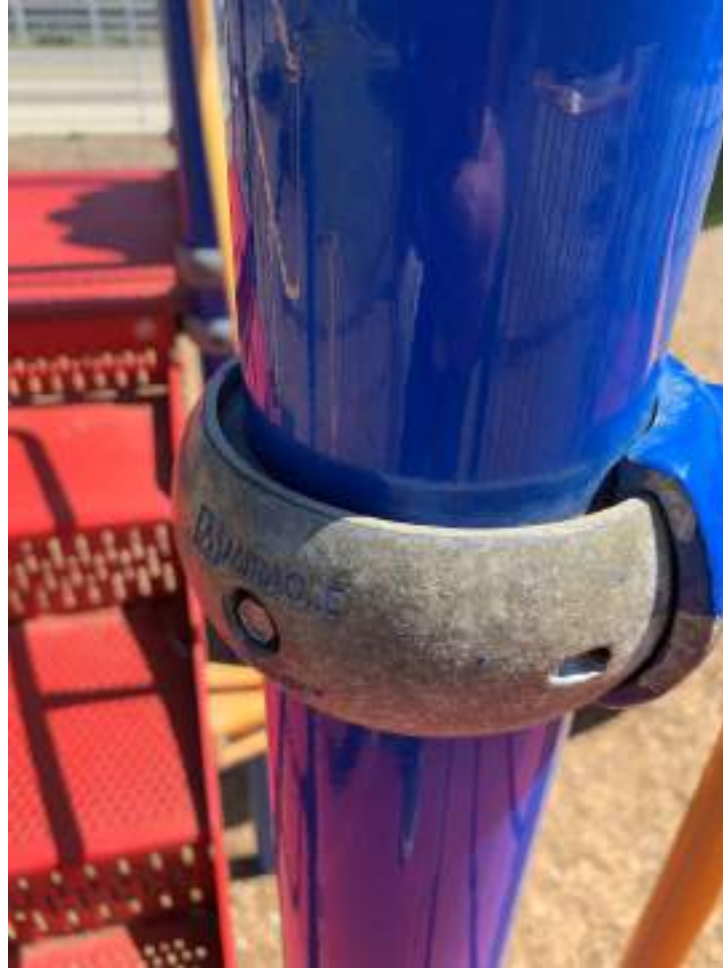
Corrosion on fasteners and clamps.
