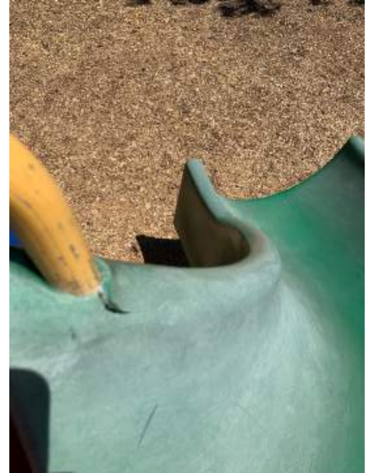
Slide Broken-Entanglement and laceration hazard.
