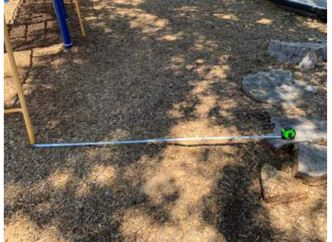
Use zone/Fall zone violation with Stumps.
