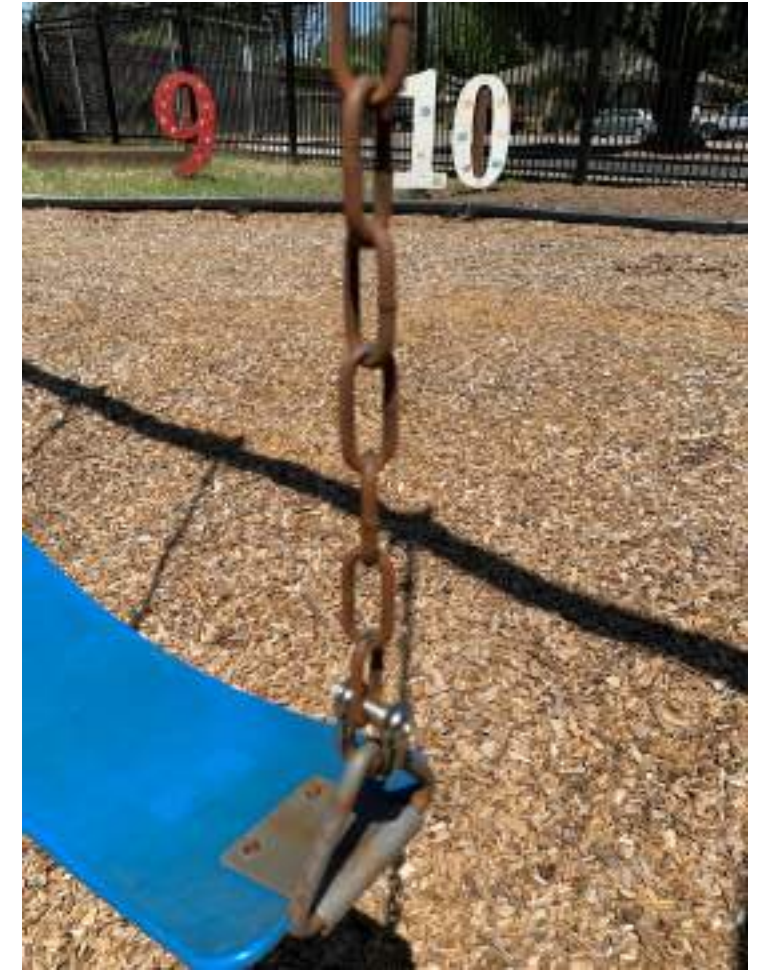
Corrosion on chains, seats, and fasteners.
