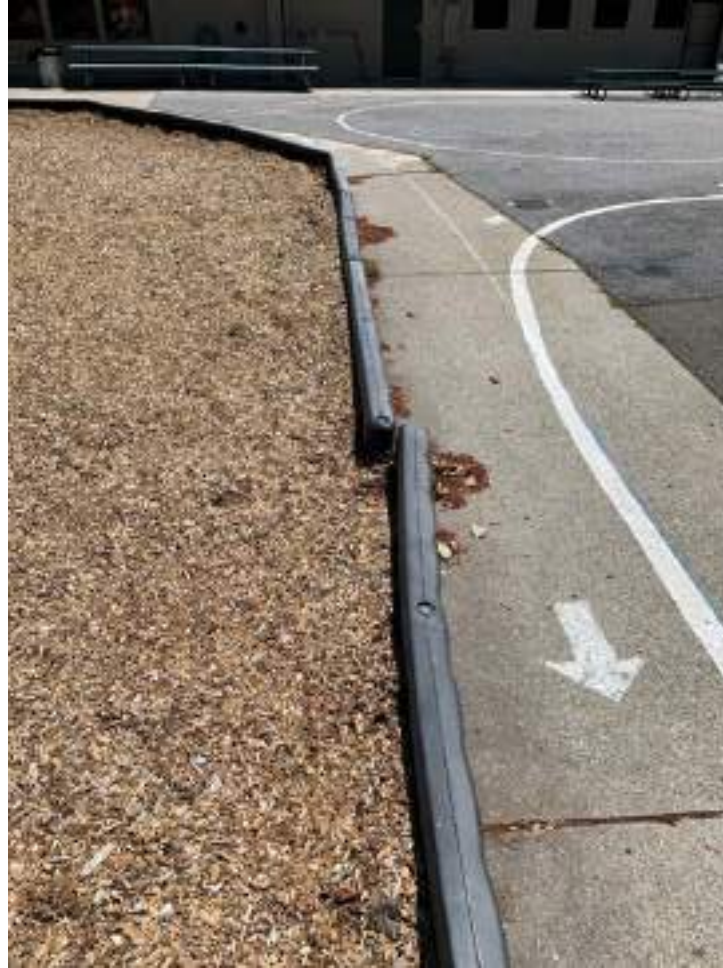
Wood fiber containment borders failing.
