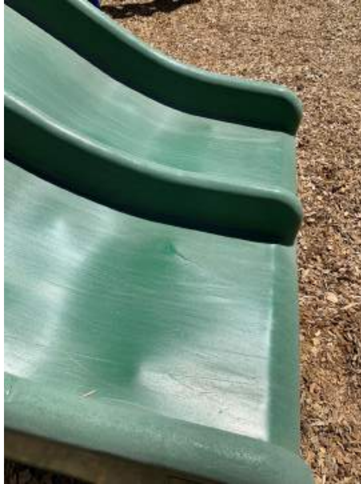
Double slide cracking at exit with large bumps where bolts are starting to protrude. Slope and slide run out questionable.
