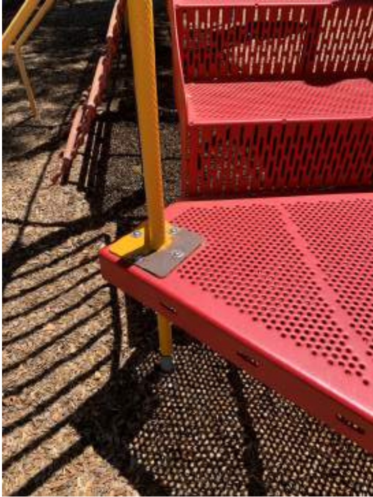
Transfer station missing step.
