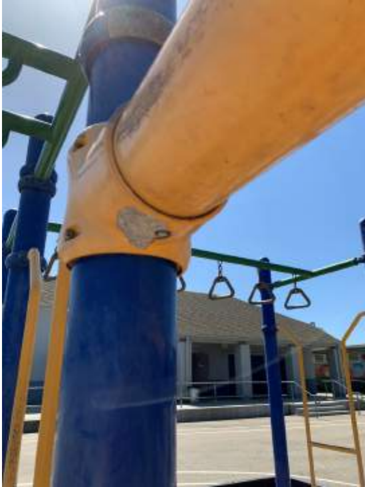
Corrosion and mold evident.
