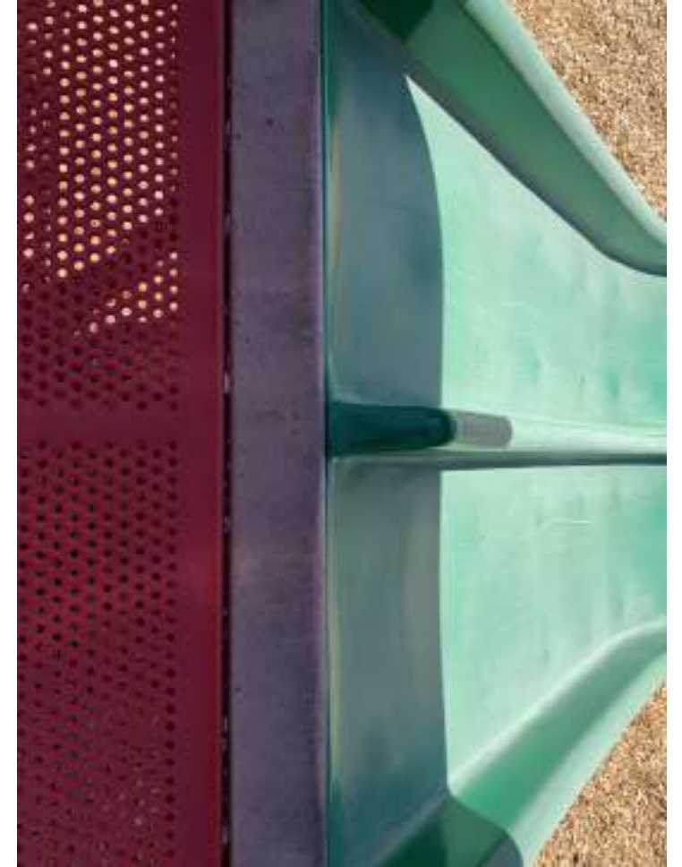
Caulking needed at slide entry to mitigate entanglement hazard. Page 64
