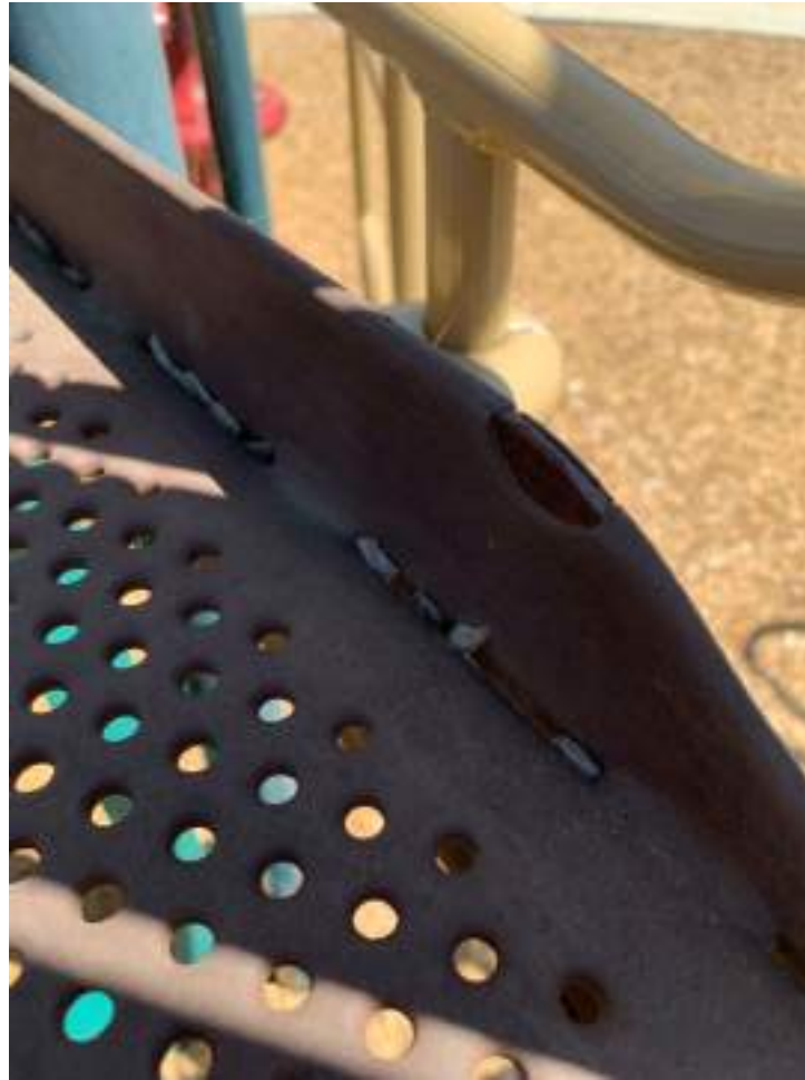
Exposed rusty edges on stairs and decks.
