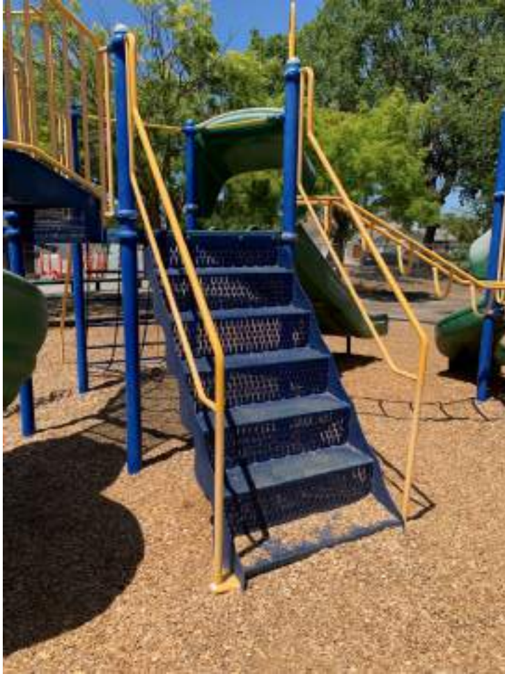
Stair railings not compliant for children under 5 years old.
