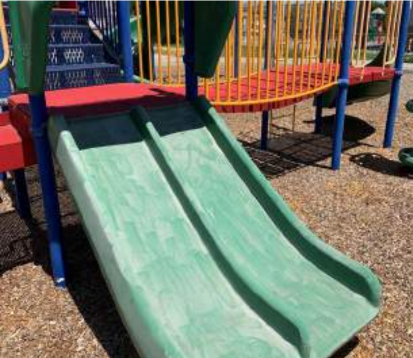
Deterioration of plastic slides make slides rough and scratchy.
