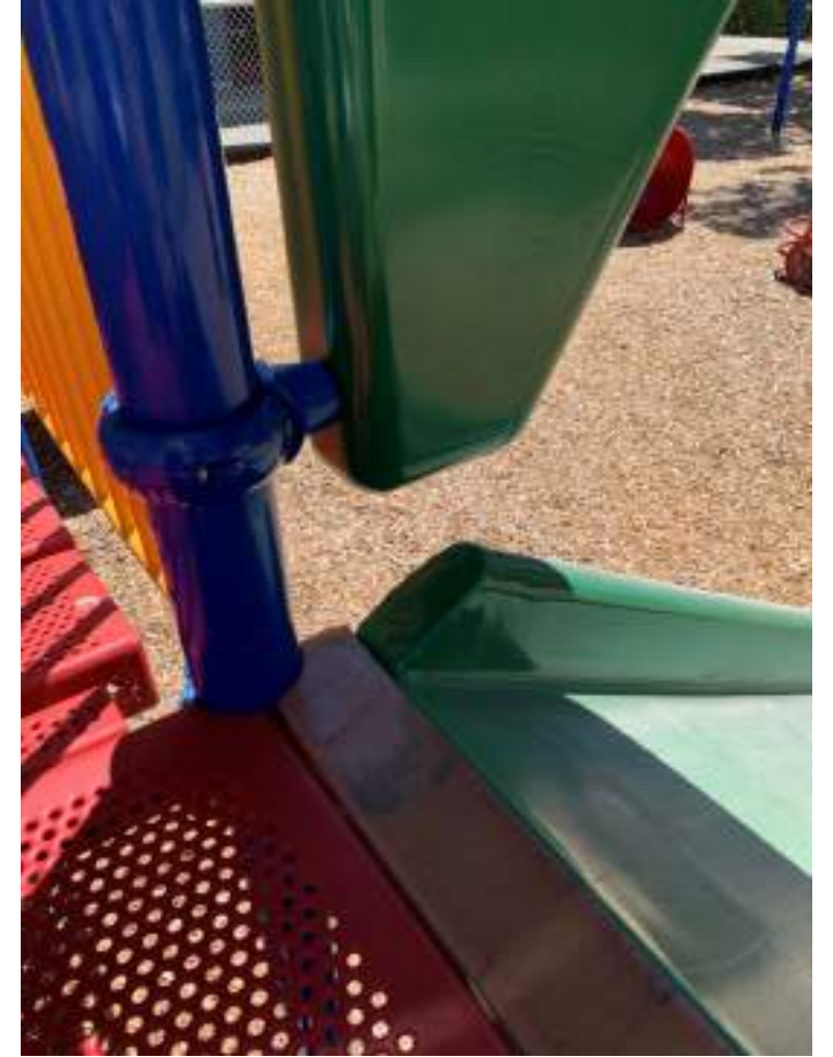
Potential partially bound neck entrapment.
