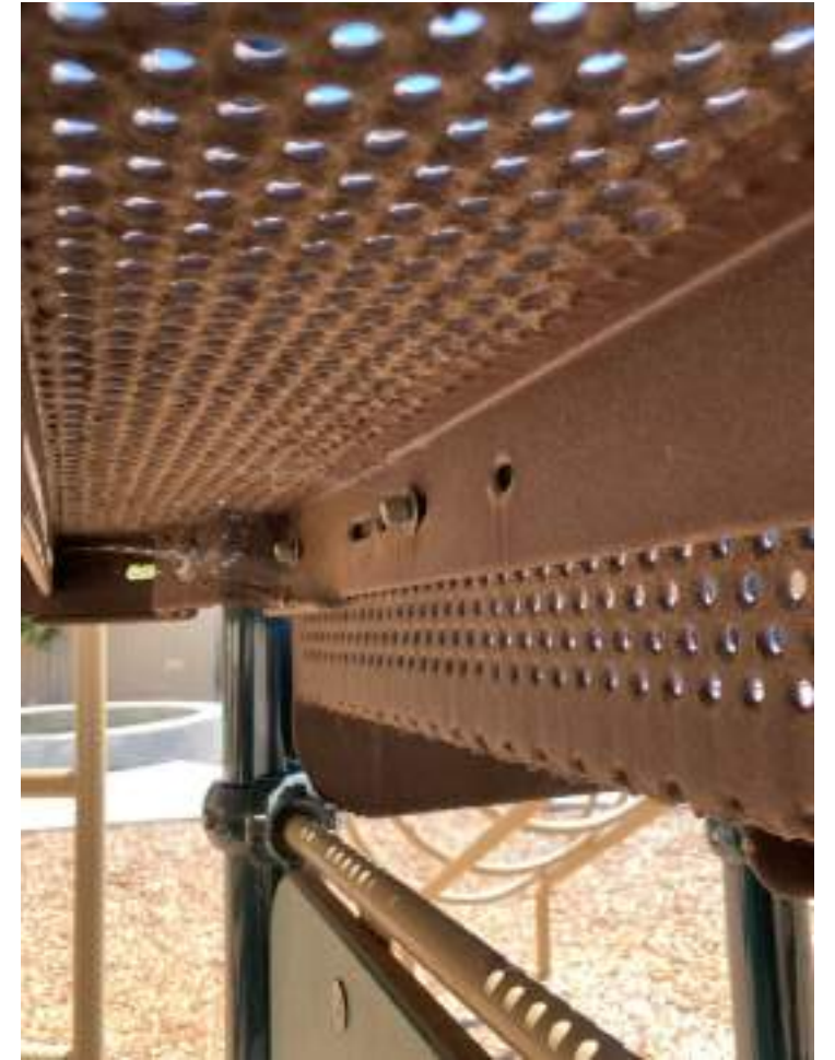
Broken bolts and bolts pulling out of deck connection to stairs. Protrusion hazard. Page 67
