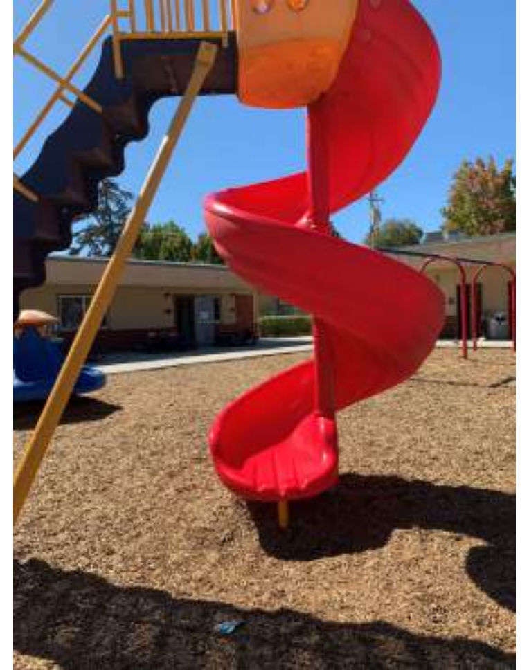
Support Post compliant but not conducive to safe flow of use. Page 70
