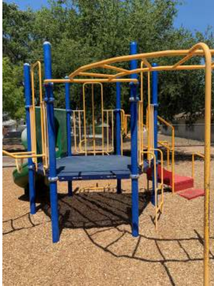
No entry enclosure for overhead climber from elevated deck.
