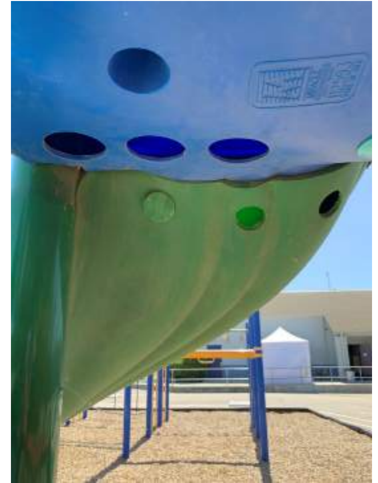
Holes in plastic slides allow insects to nest.
