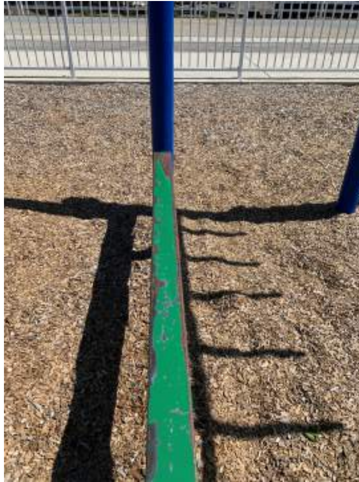
Rusted balance beam.
