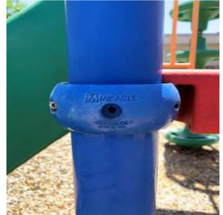
Missing bolts from support clamp
