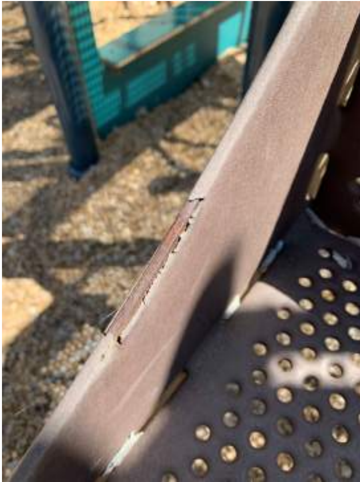
Exposed rusty edges on stairs and decks.
