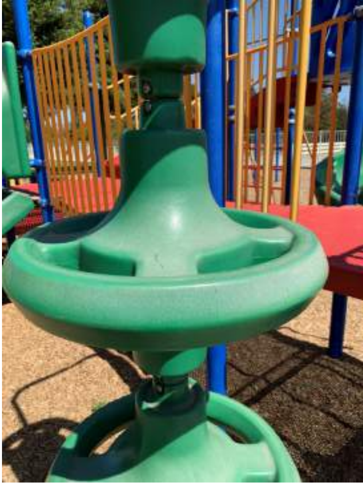
Loose on post and footing.
