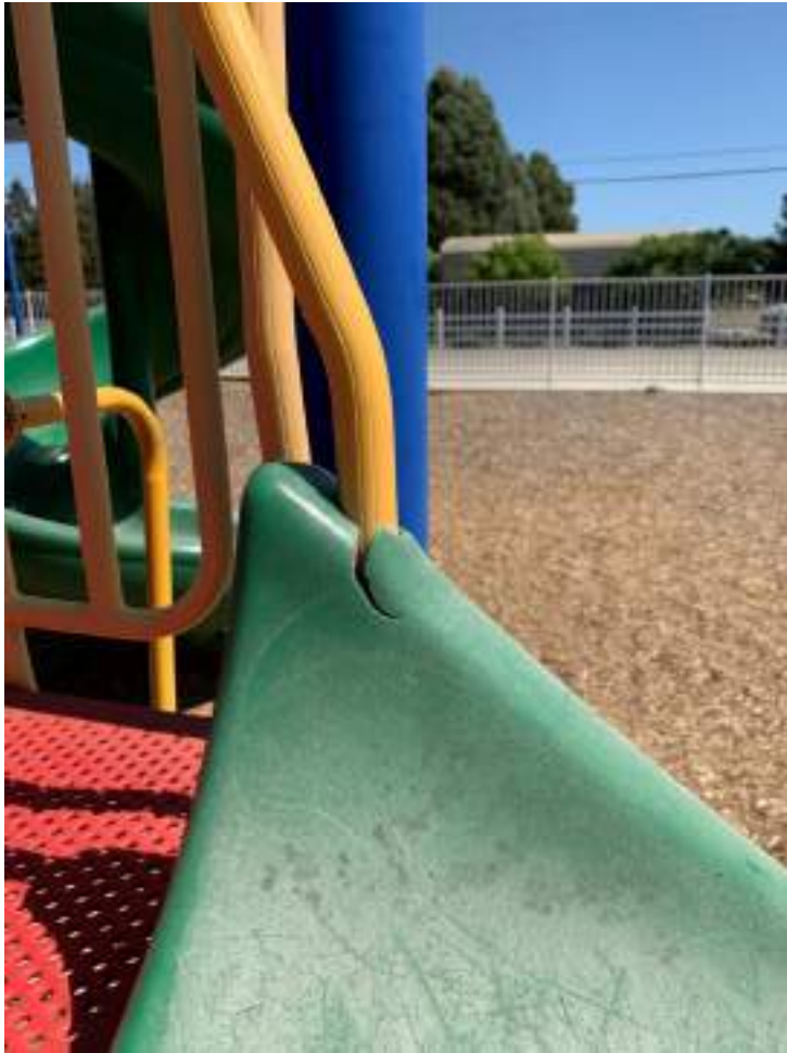
Broken Slide: Entanglement and laceration hazard.
