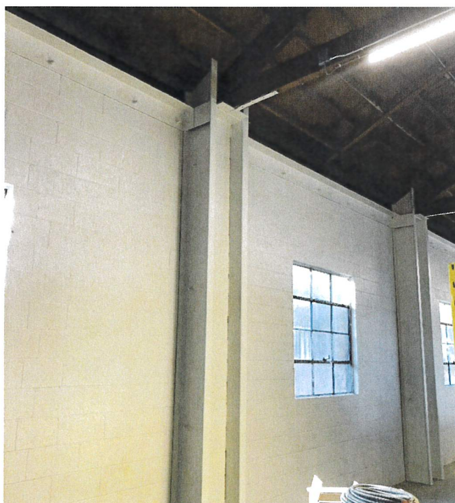
Steel Channel Columns and Angle Girts
