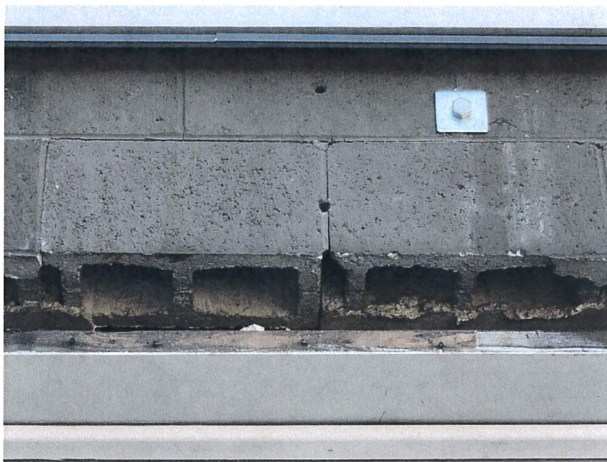
Cracking at Mortar above Modified Garage Door
