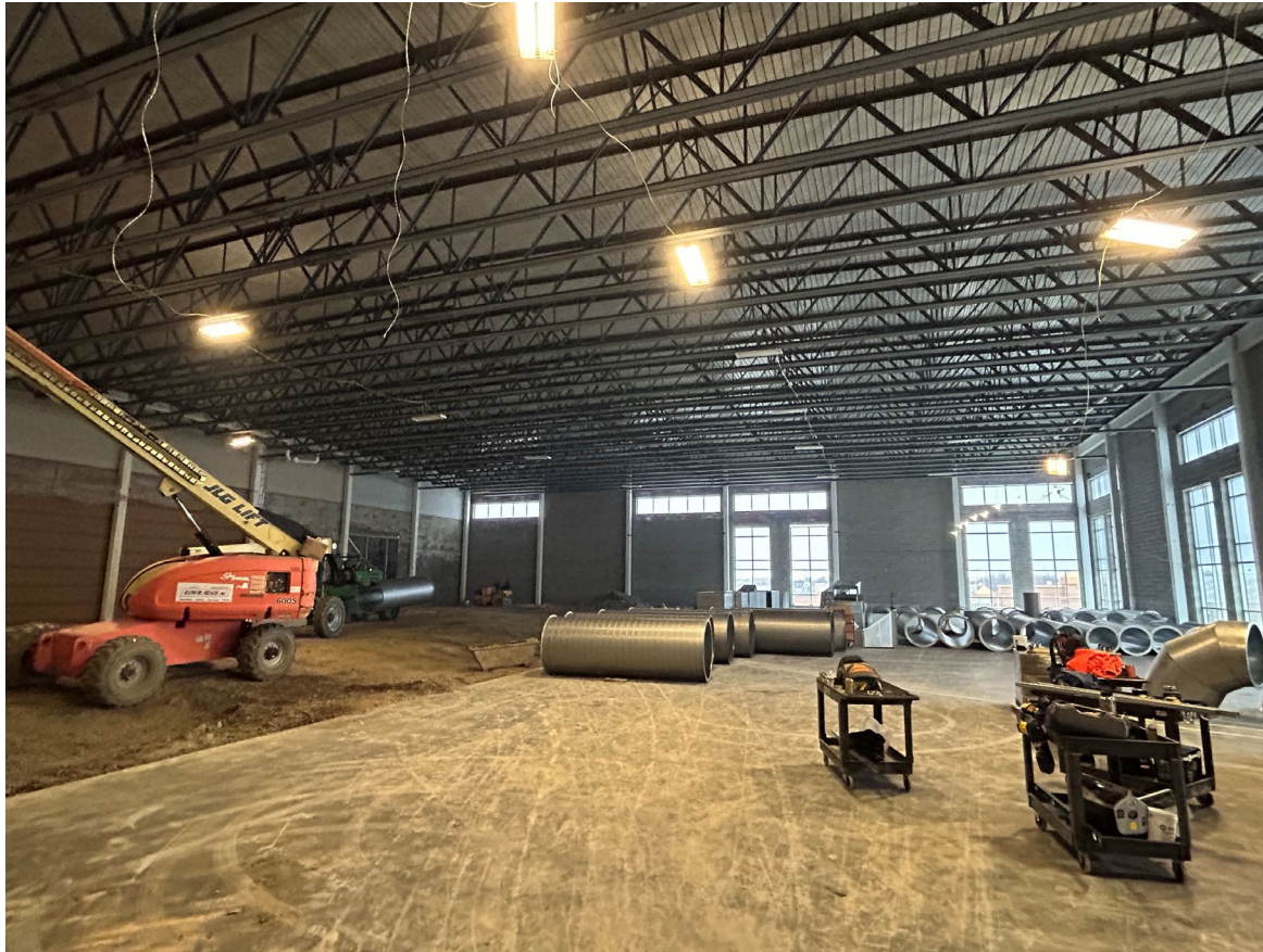
Unit T Athletic Addition Interior
