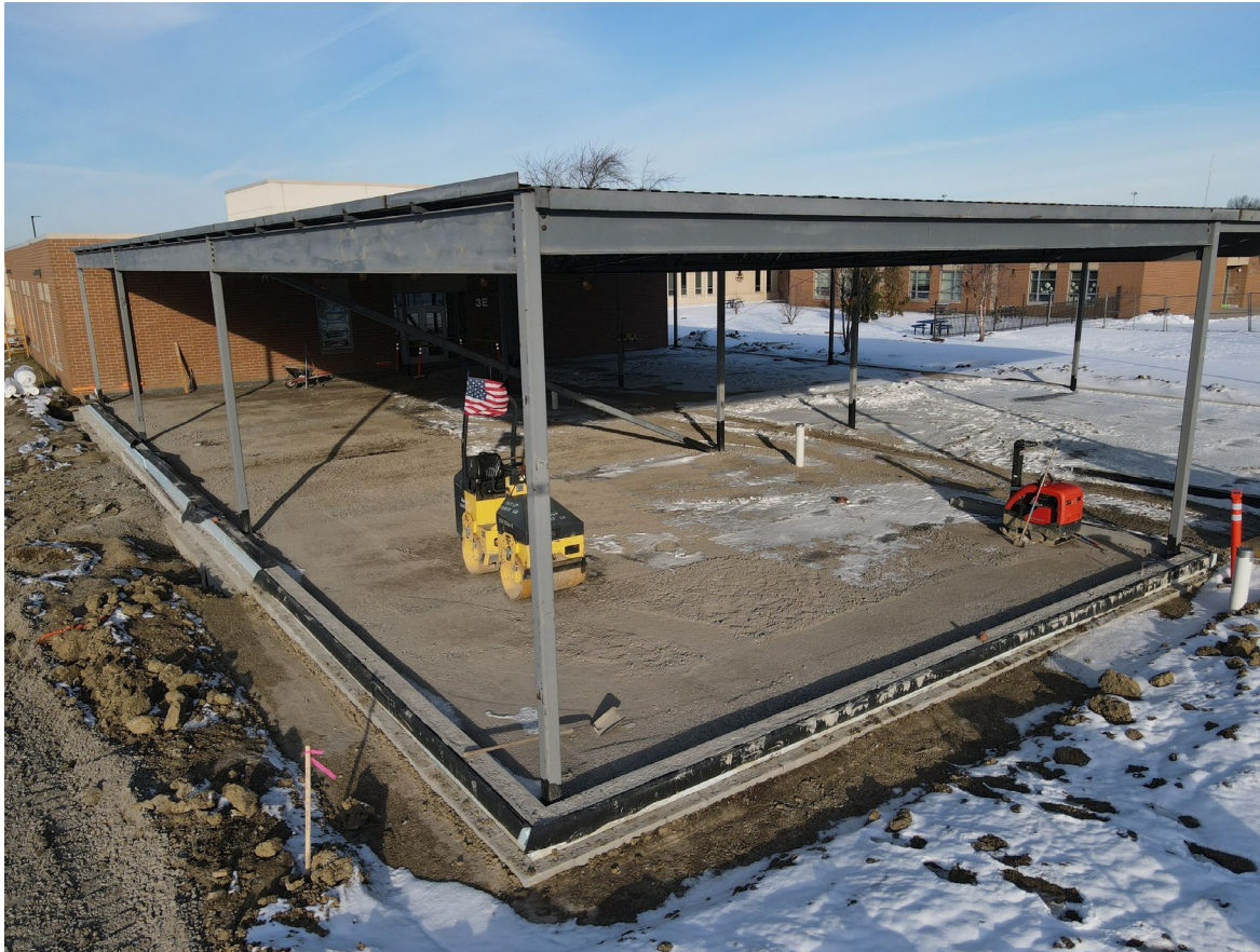
Unit D Classroom Addition
