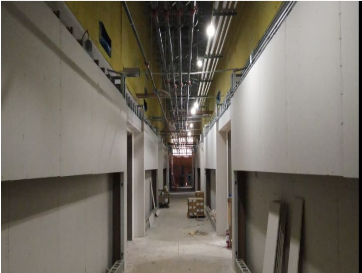
Classroom Addition Interior
