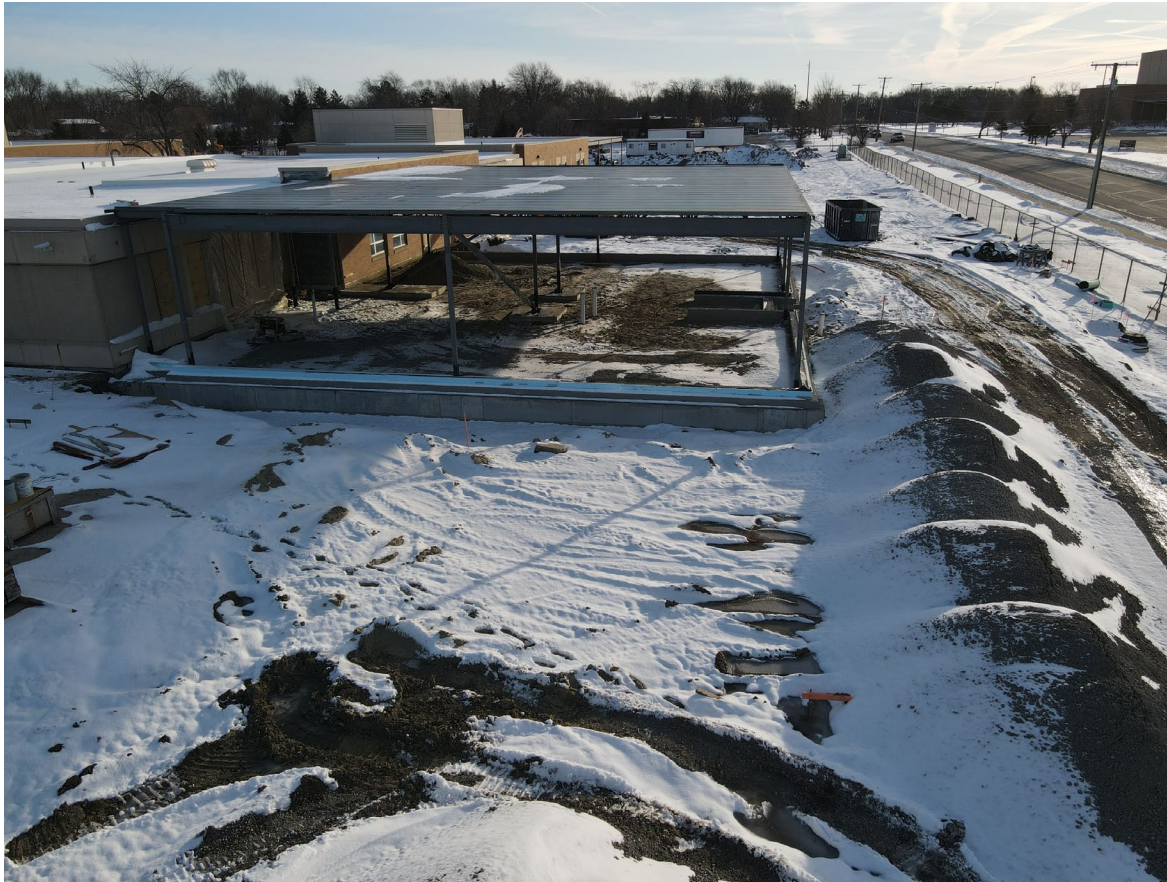
Unit E Classroom Addition
