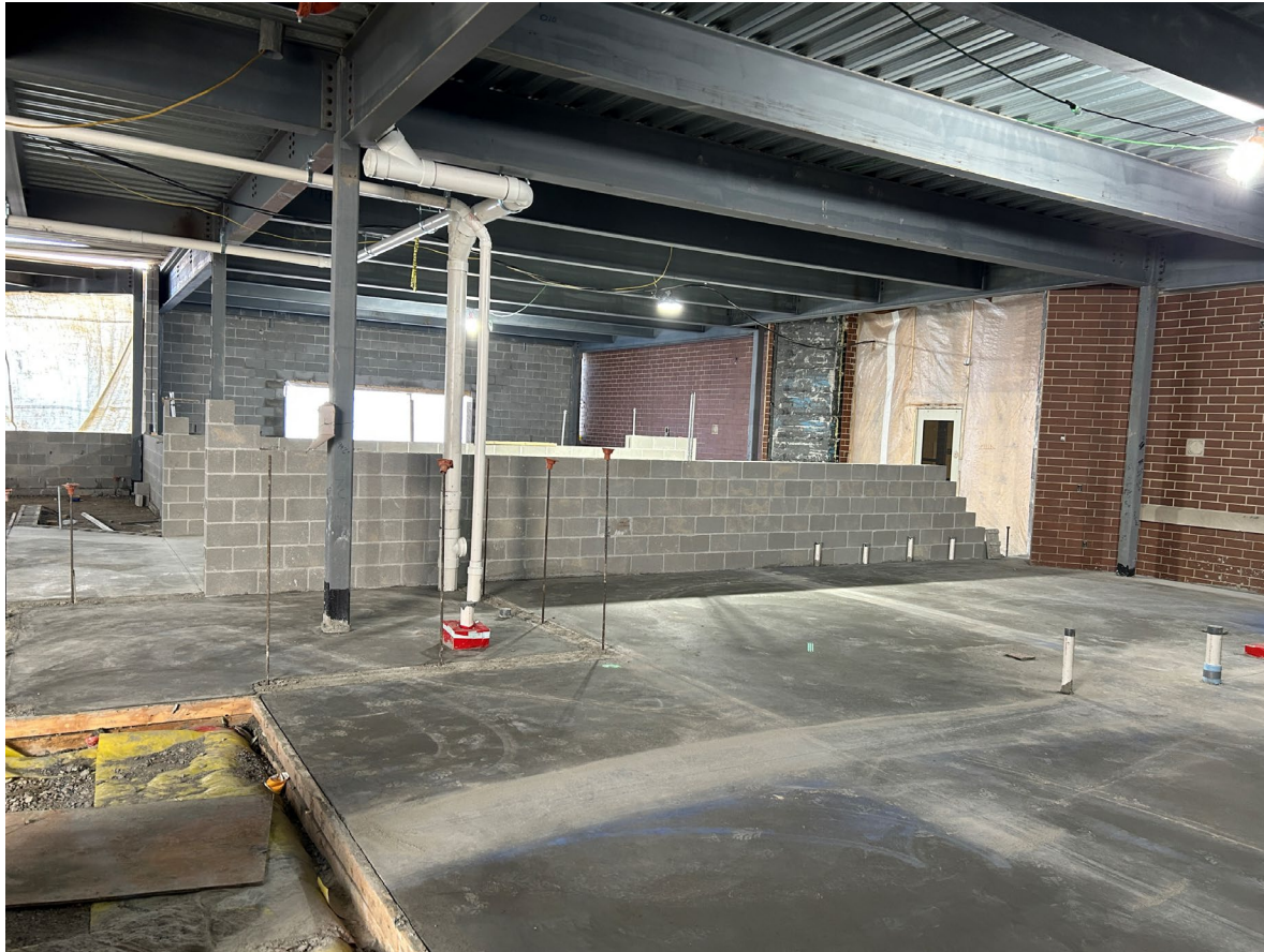
Classroom Addition Interior CMU
