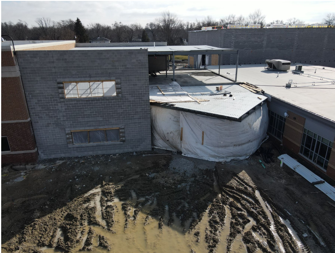
Classroom Addition Exterior CMU
