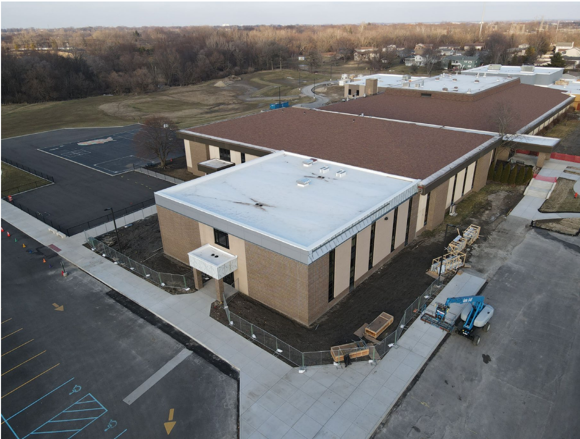
Classroom Addition Metal Panels
