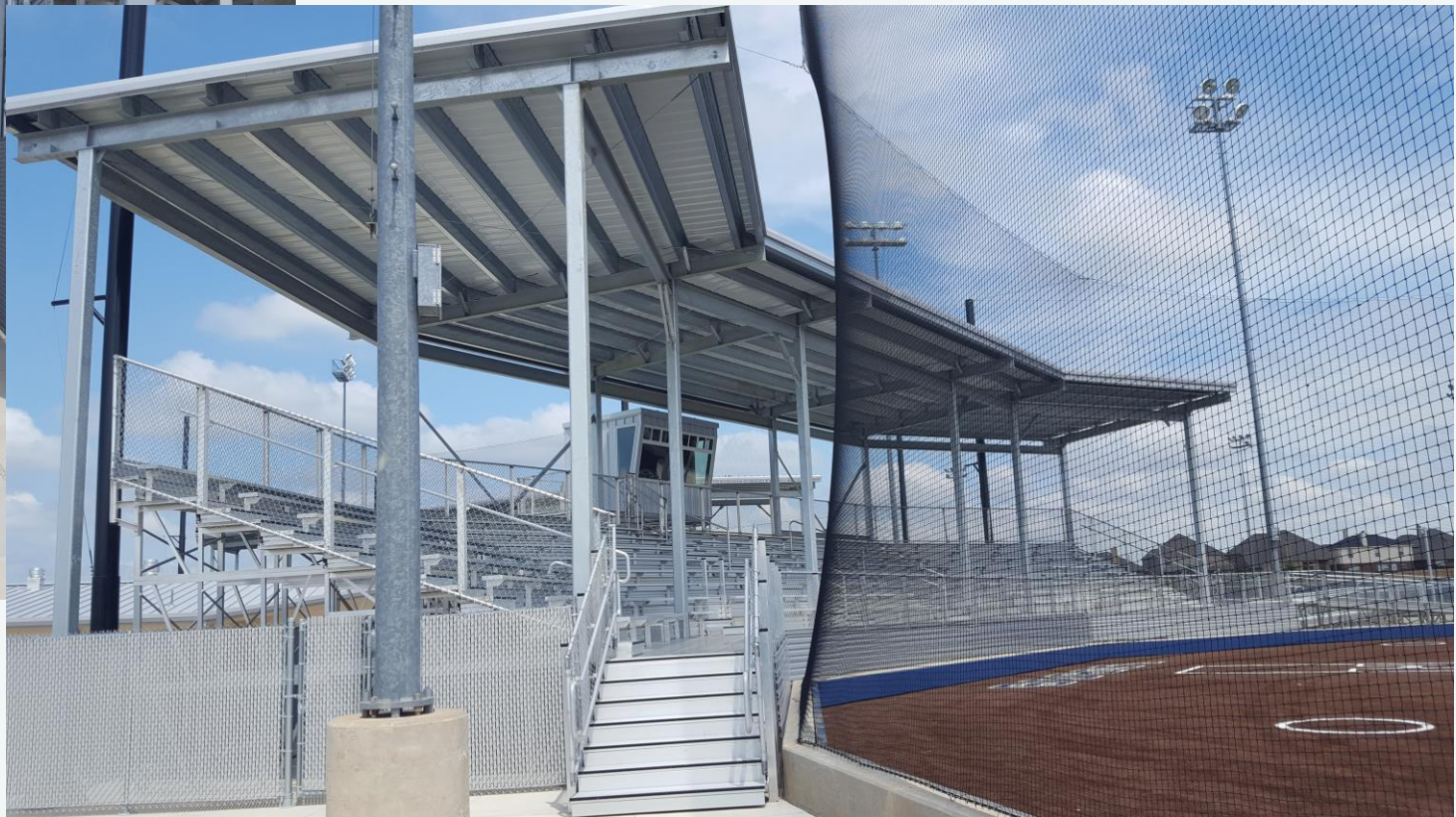
Covered Softball Bleachers & Press Box
