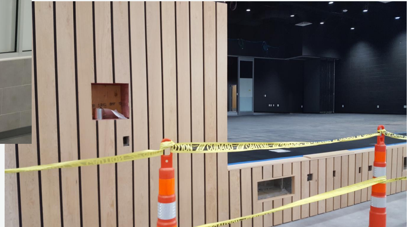
Wood facing at stage front
