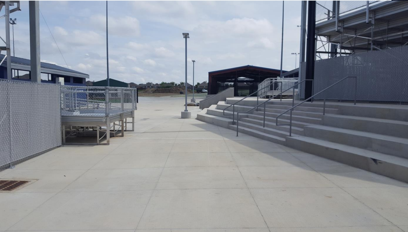
Concourse Looking East
