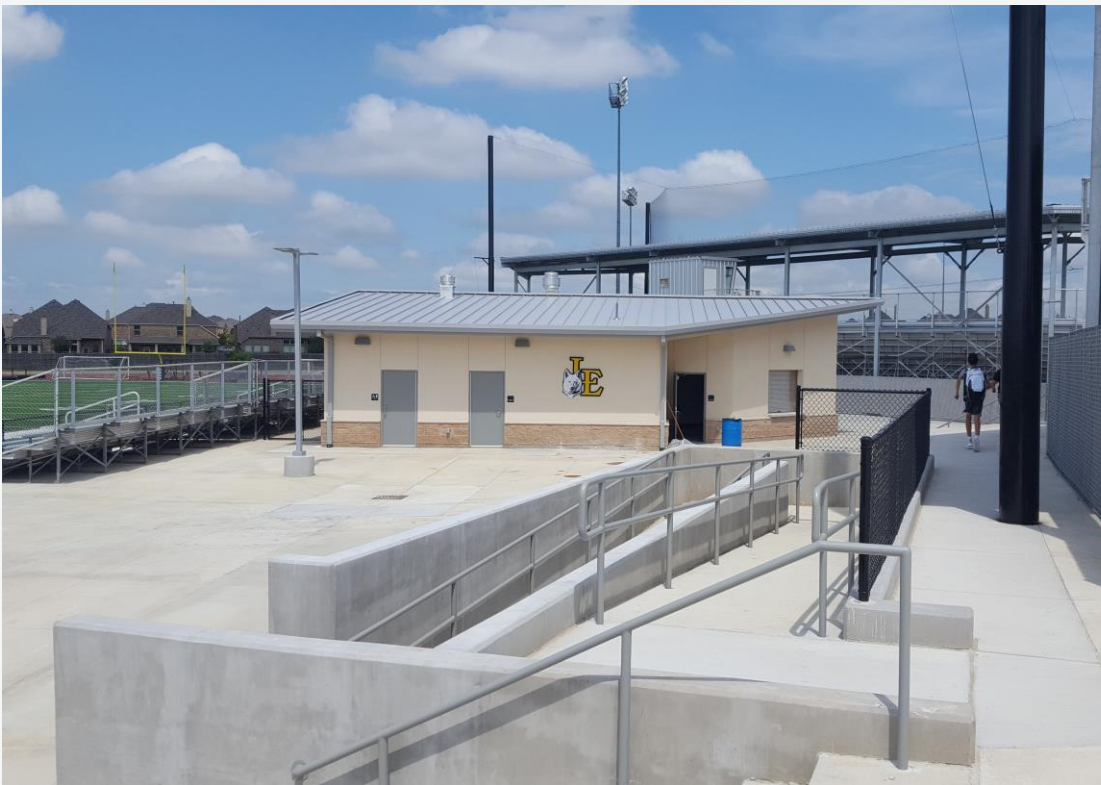
New Concessions Building
