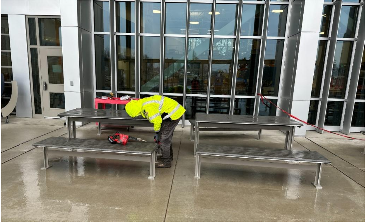
Bench and table installation in the common area courtyard
