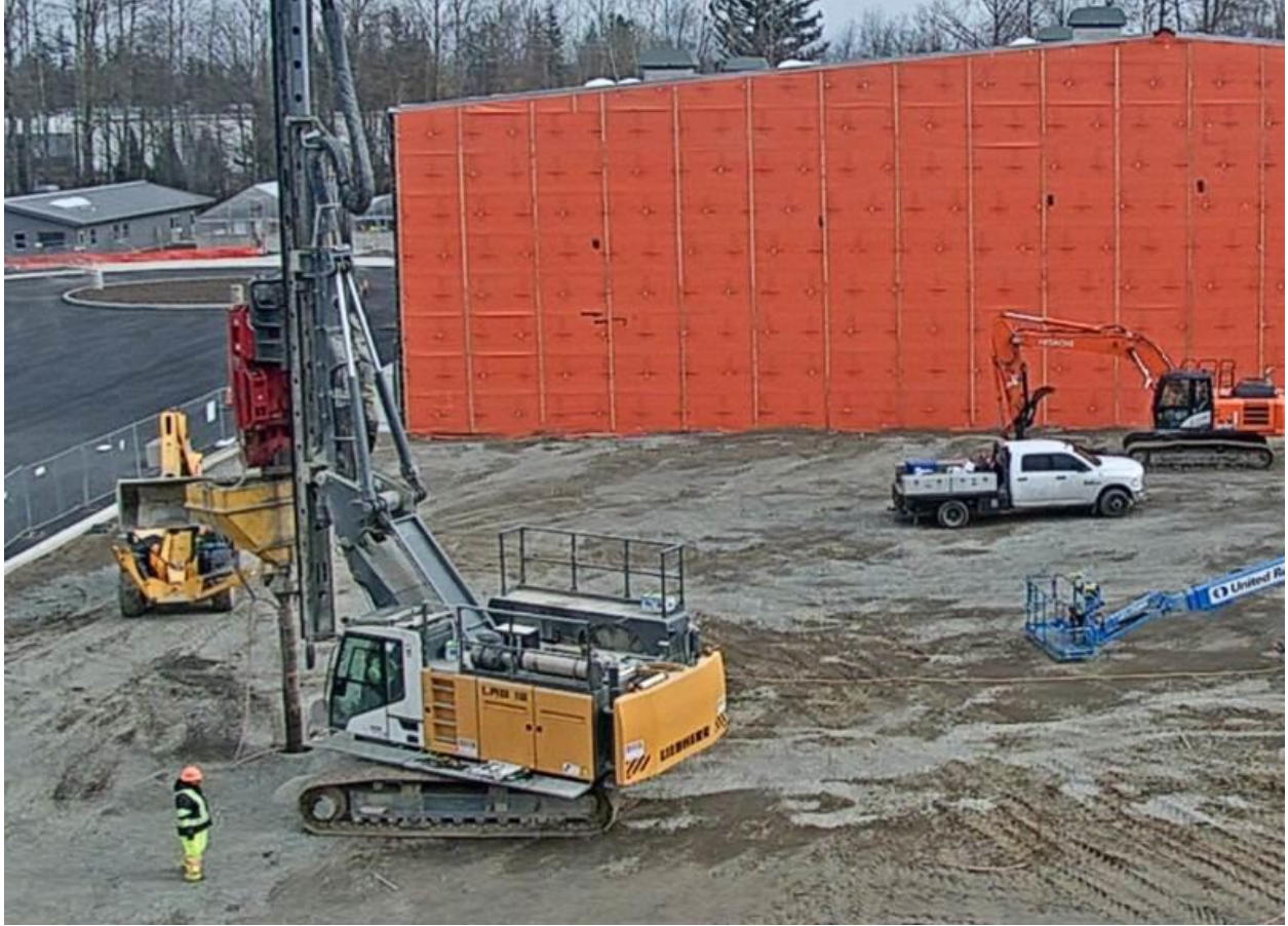
Geopier installation at the CTE Wing site
