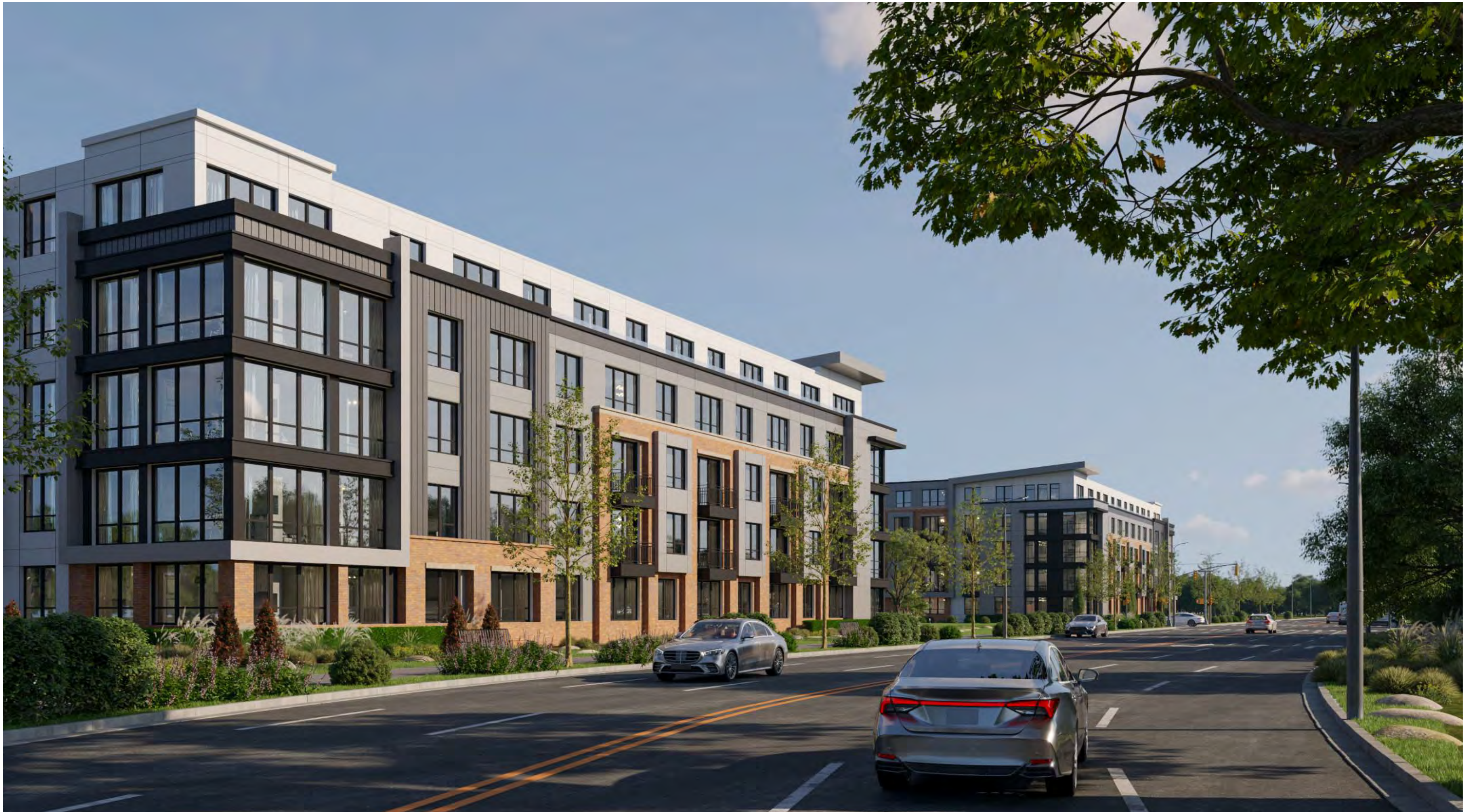
VIEW OF TROUT BROOK DRIVE LOOKING SOUTH
