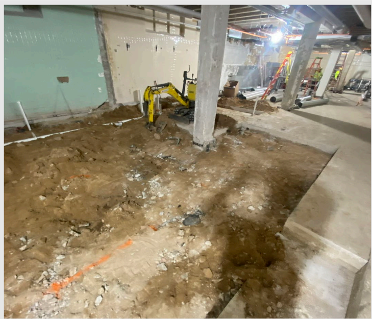
In the lower-level locker room renovations, underground plumbing was installed, and the new concrete floor was poured
