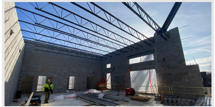
Following the completion of the first-floor masonry walls, steel roof joists have been set to begin enclosing the space
