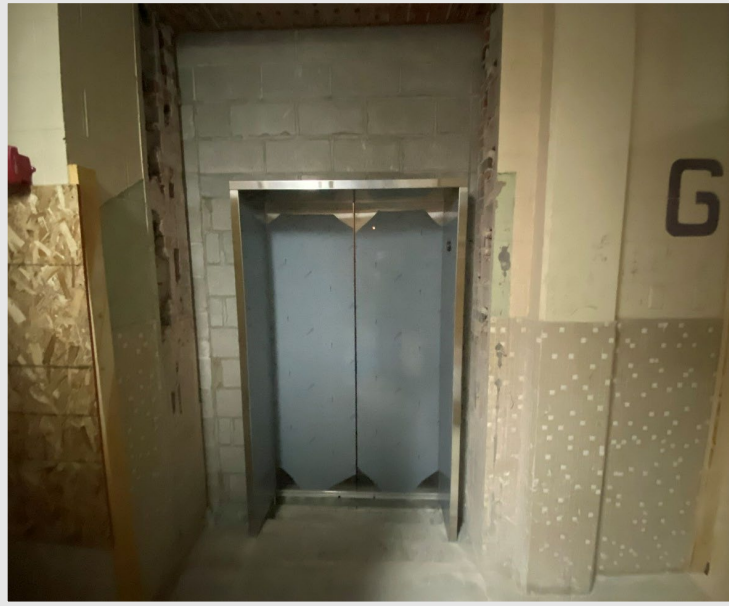
The new welcome center lobby elevator is scheduled to be completed this winter
