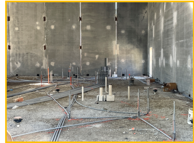
GYM Underground MEP
