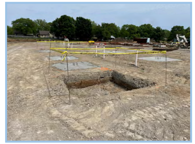
Prep for Spread Footings
