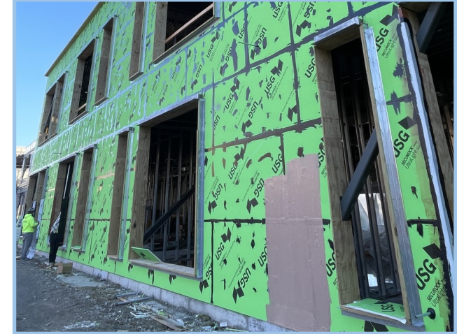
Detailing Prep Before Air Barrier
