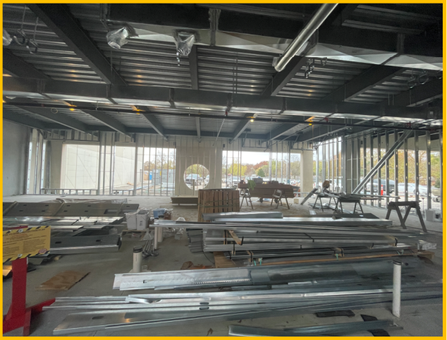
Area A Interior Stud Framing
