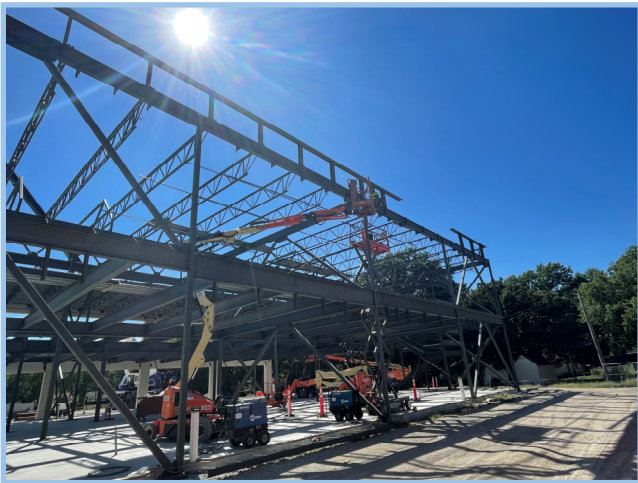
Area B Steel & Detailing
