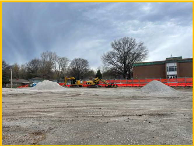
Building Pad Prep
