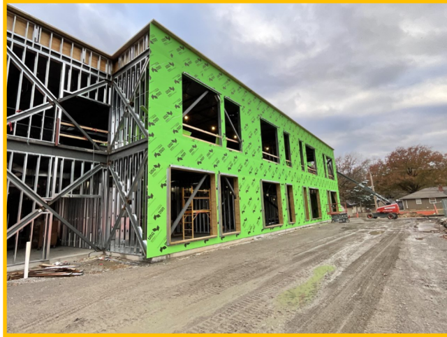
Area B Exterior Sheathing
