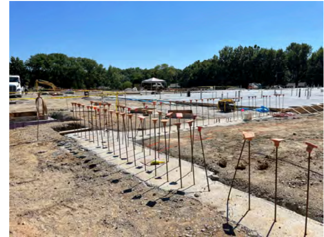
Continued Footings to Gym Area
