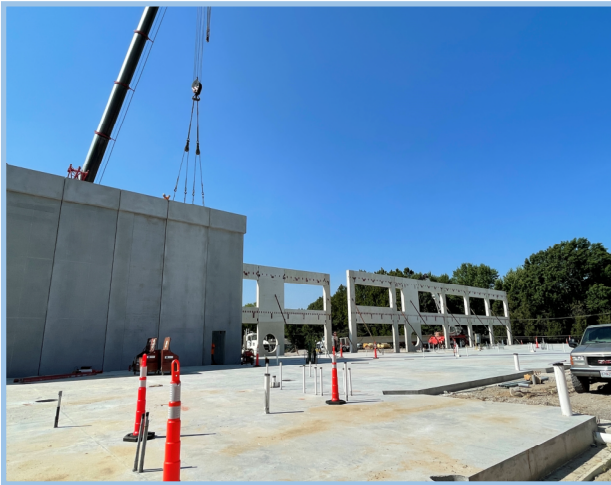
Setting Gymnasium Precast
