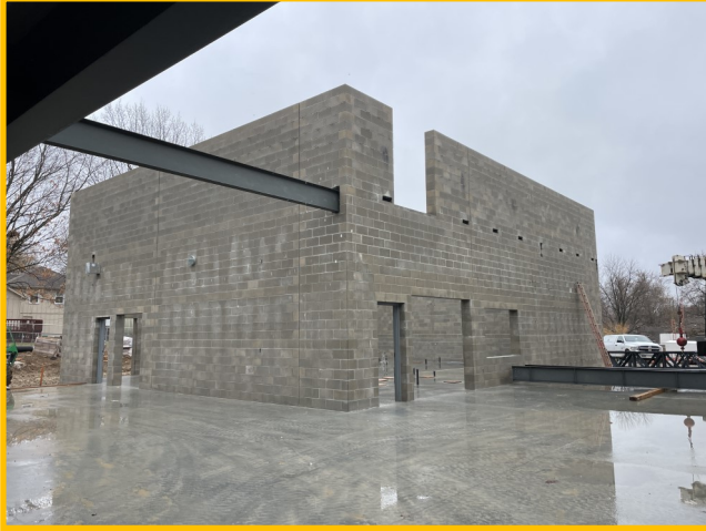
Kitchen CMU Walls
