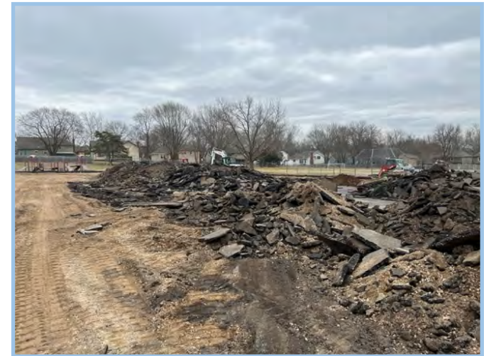
Prep For New Building Pad
