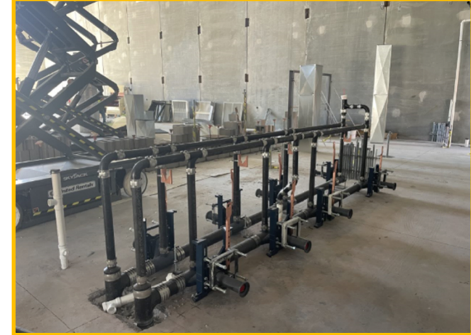
Gym Rough-In and CMU Walls
