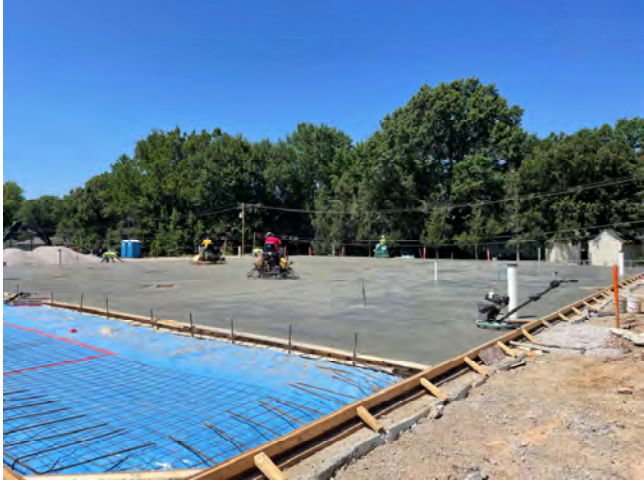
Section 1 Slab on Grade
