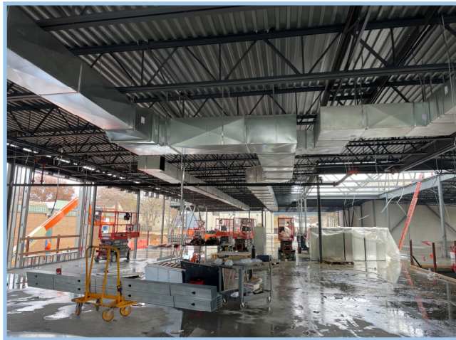
Level 2 Area B Overhead & Framing
