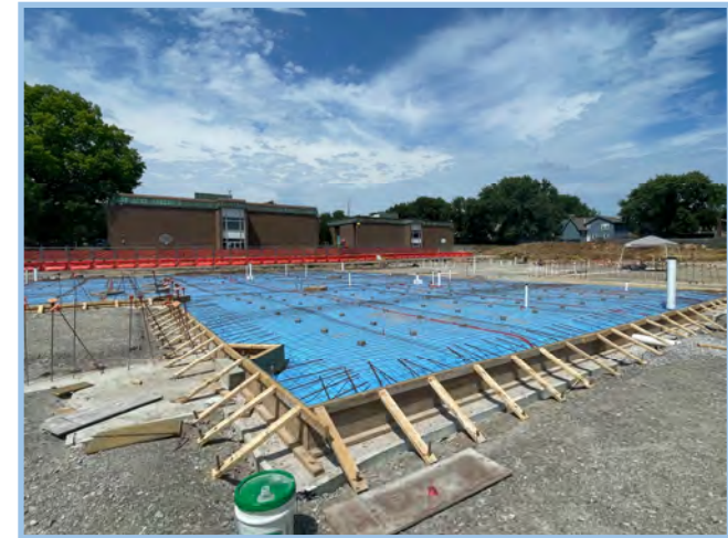
Formwork & Prep for Slab Section 2
