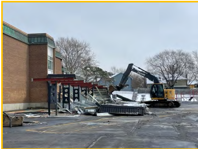
Removed Existing Canopy
