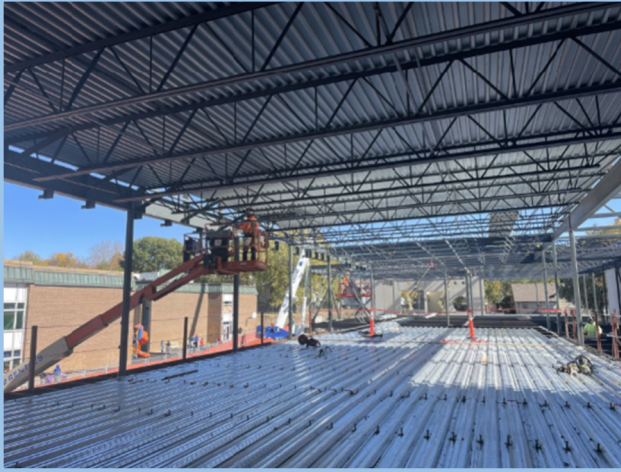
Steel Erection & Detailing
