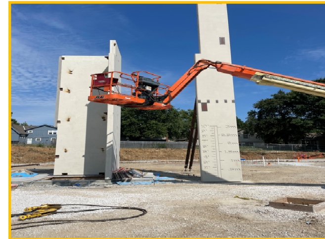
Feature Wall Precast
