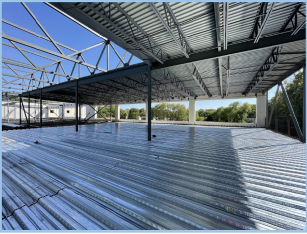
Area B Steel & Decking
