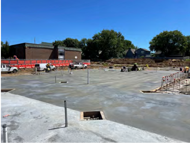
Section 3 Slab on Grade Poured
