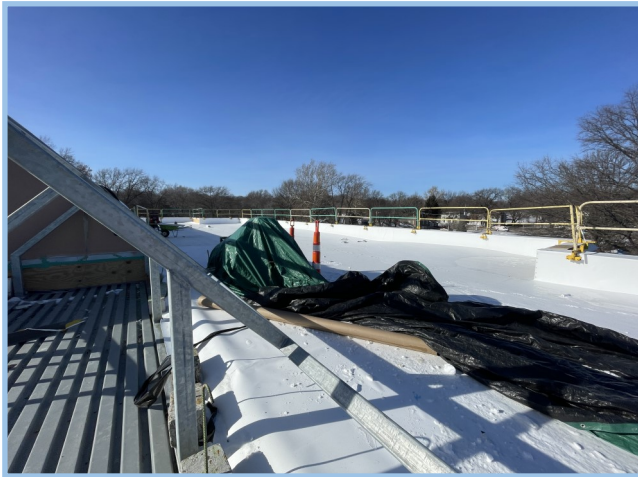
Area B Roofing
