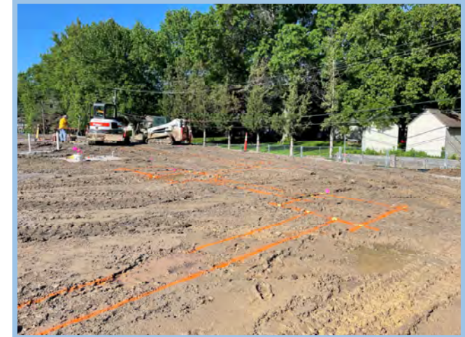
Continued Footing Layout and Excavation
