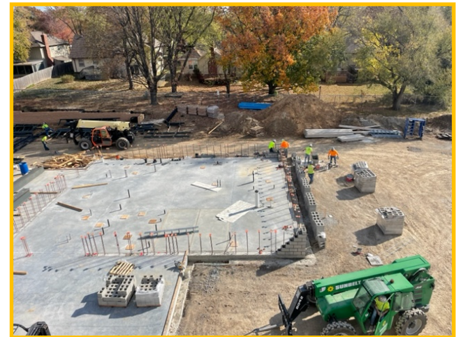
Area A Kitchen CMU Walls
