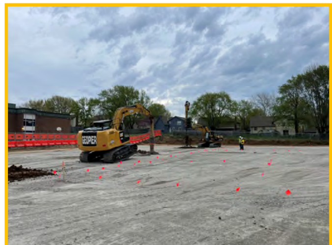
Completed Aggregate Piers
