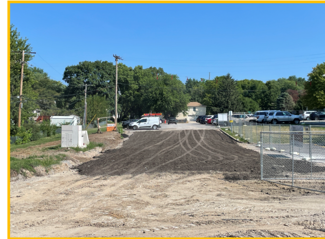
Construction Entrance Asphalt Prep.
