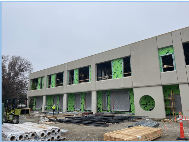
South Elevation Sheathing
