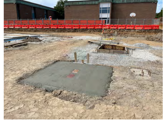
Precast Footings Poured
