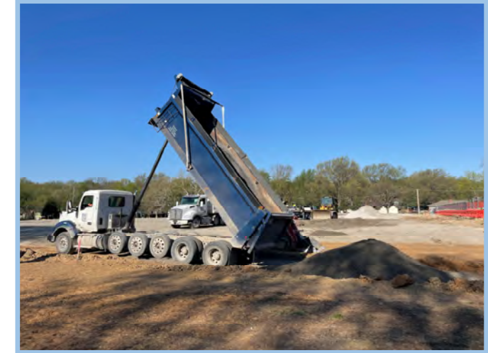
Raising Grade At Laydown Area
