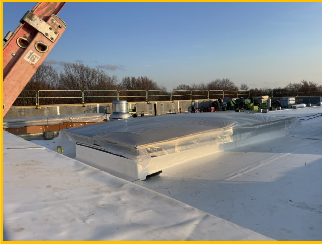
Gym Roofing Continuing
