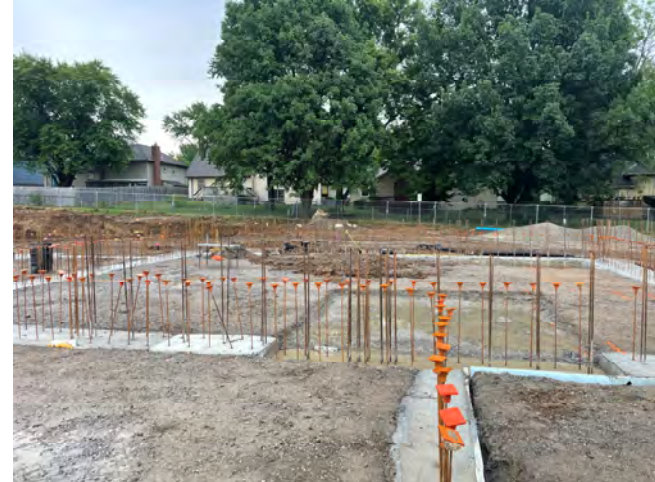
Kitchen Footings Completed
