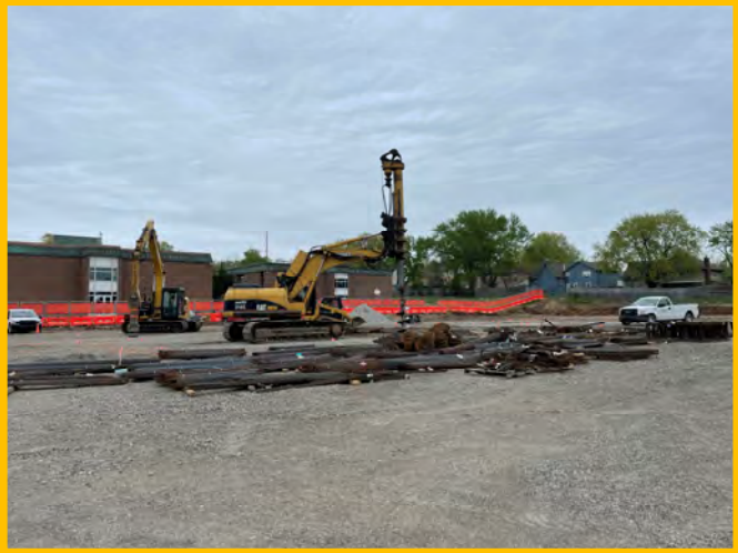
Footing Reinforcement Delivery
