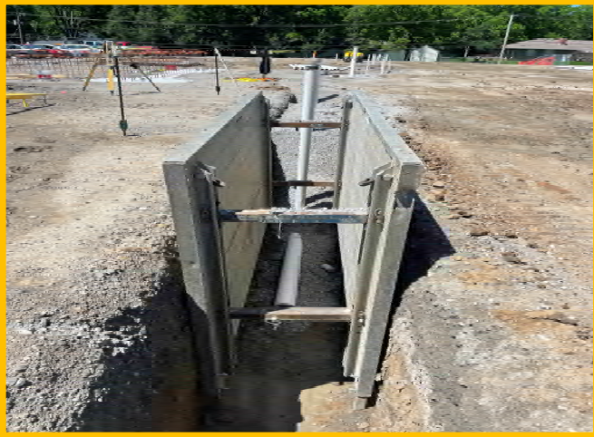
Plumbing Underground Sanitary
