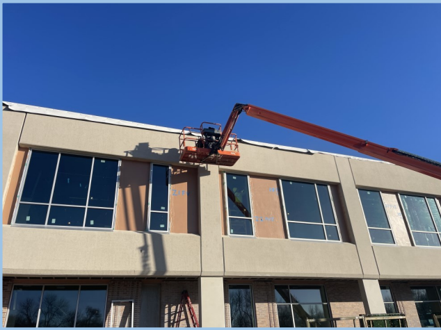
Finishing South Glazing
