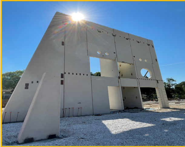
Feature Wall & Elevator Core
