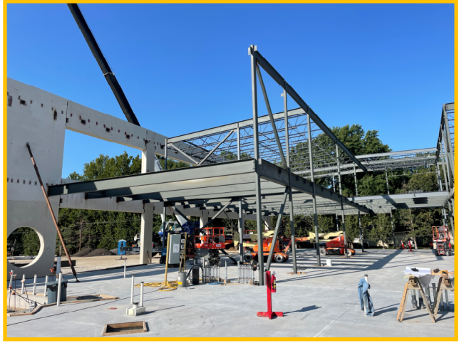
Area B Steel & Detailing
