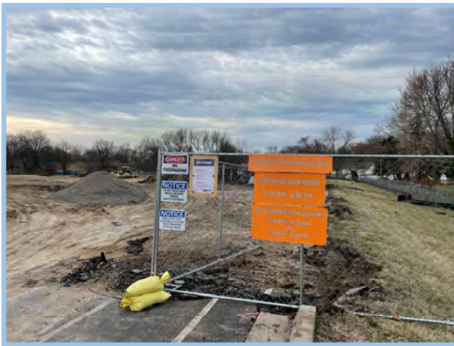
Temp. Fencing and Signage
