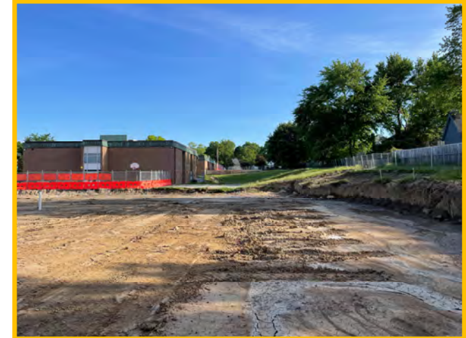
Relocated Fencing for Grading & Utility Install
