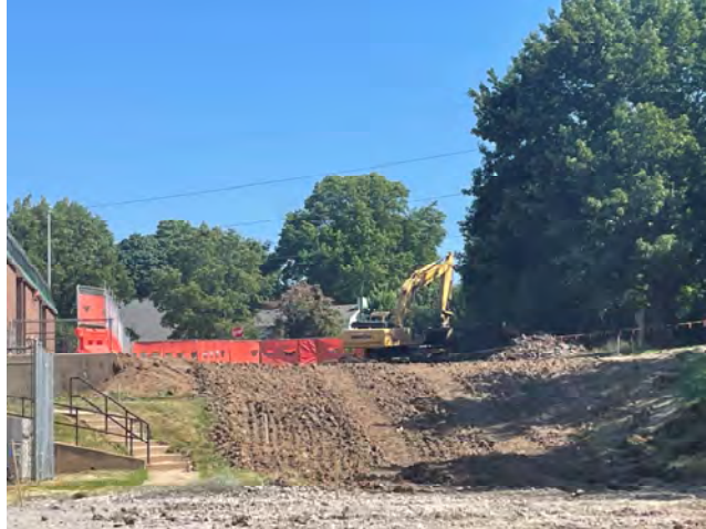
Grading on Northeast Corner
