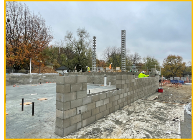
Area A Kitchen CMU Walls
