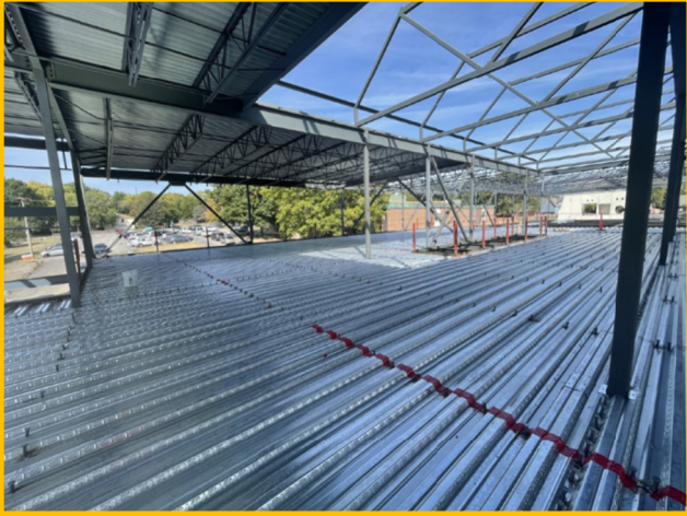
Area B Steel & Decking
