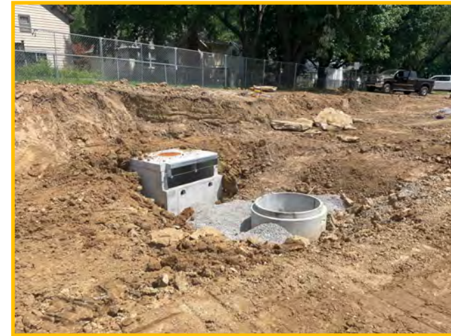
Continued East Storm Sewer
