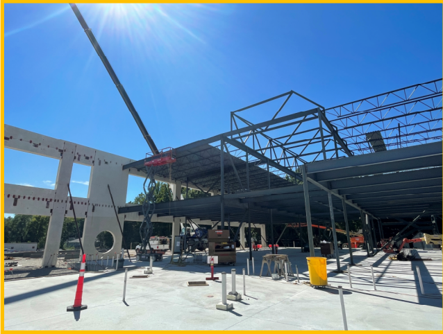
Area B Steel & Detailing
