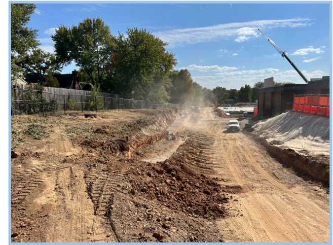
East Retaining Wall
