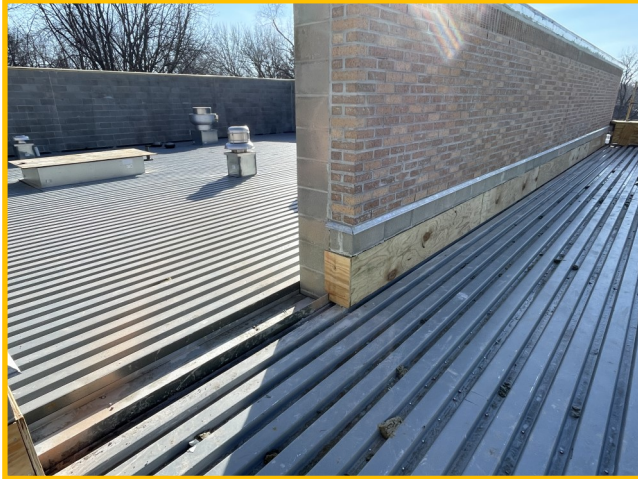
Brick at Kitchen Parapet
