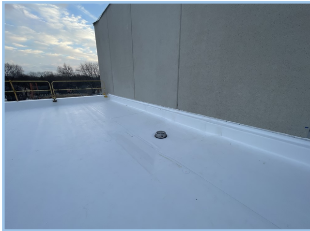
Roofing at Cafeteria
