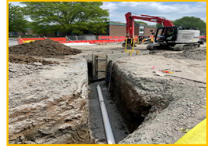
Install Plumbing Underground
