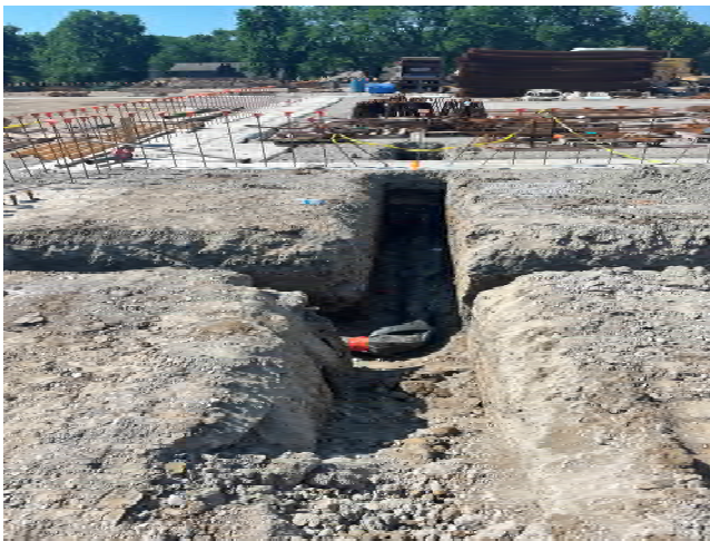
Plumbing & Electrical Underground
