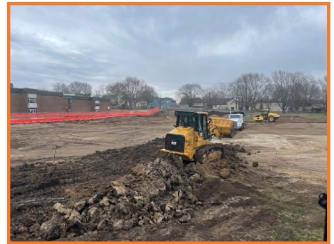
Continue Prep For New Building Pad
