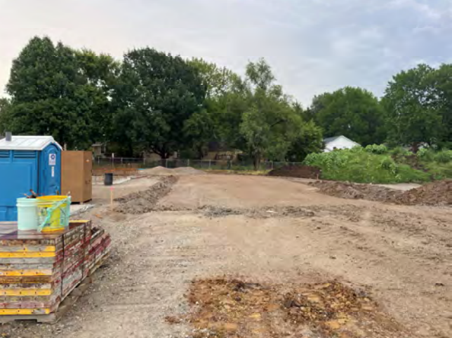
Crane Staging Area for Gym Precast
