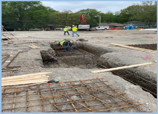
Footing Reinforcement Install
