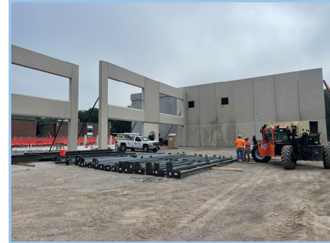
First Steel Delivery
