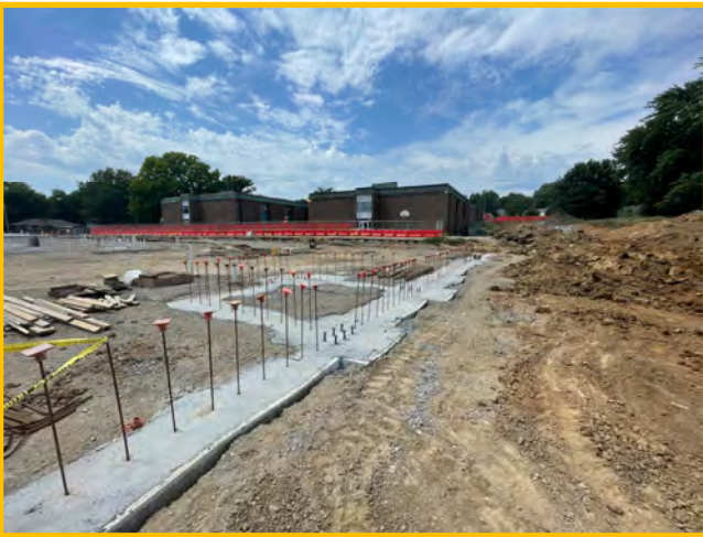
Poured Area A Footings
