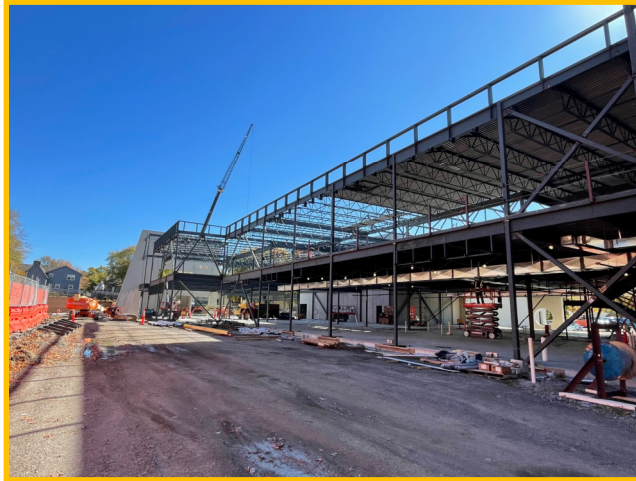
Steel Erection & Detailing
