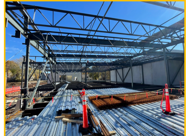
Sequence 2 Decking Install
