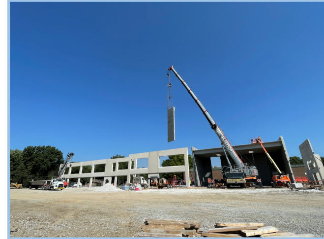
Area B Precast Complete
