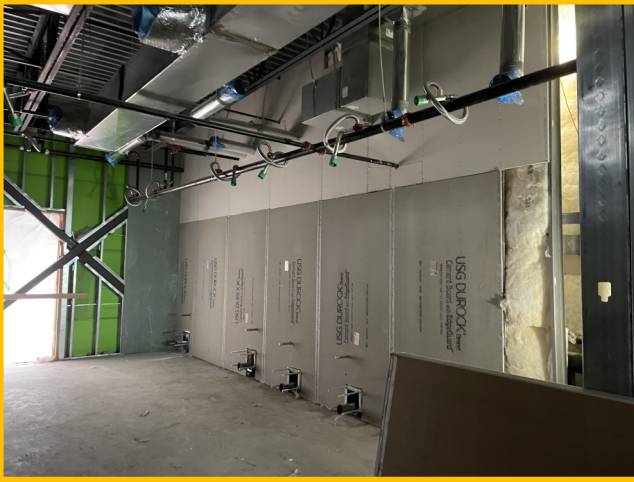
RR Backer Board Install for Tile
