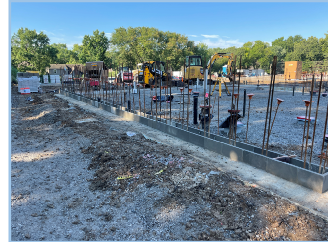
Begin Kitchen CMU
