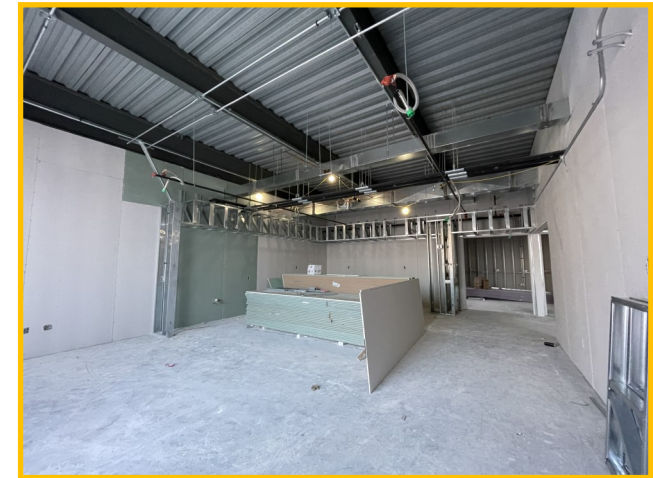
Drywall In Classrooms
