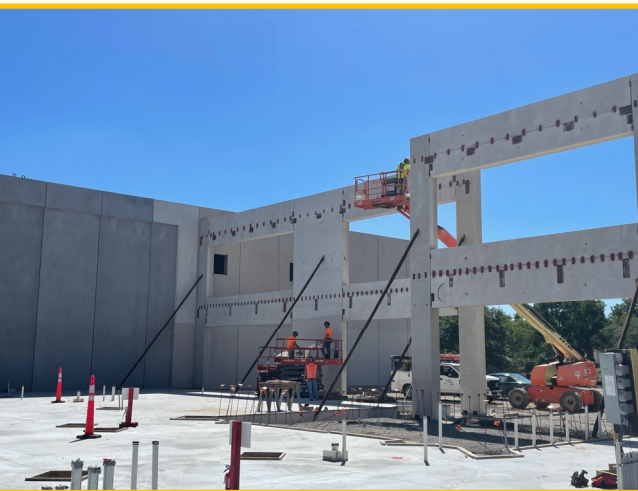
Finalizing Welding Connections
