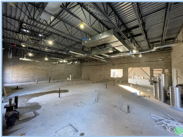
Kitchen Overhead Mechanical
