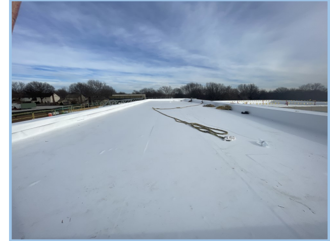
Area B Roofing
