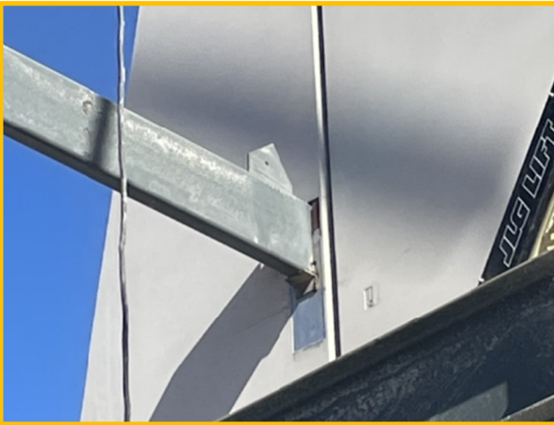
Area A Steel and Precast Connection
