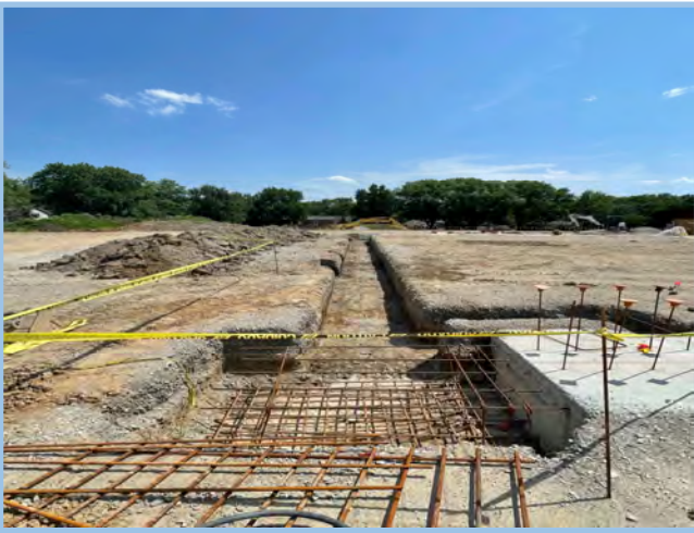
Prep For East Gym Footings
