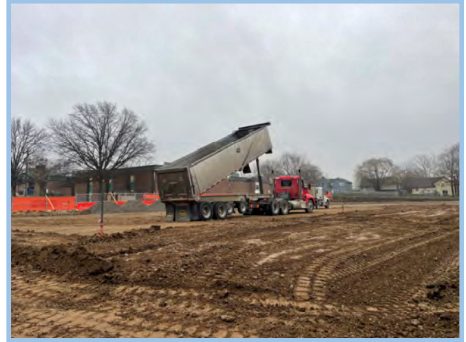
Imported Material For Building Pad
