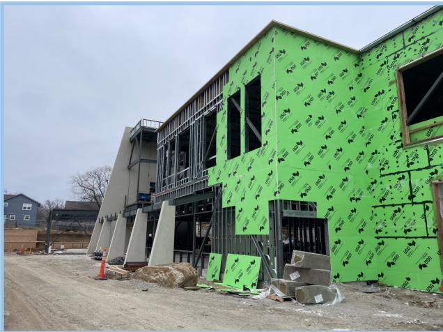
North Elevation Sheathing
