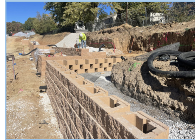
East Retaining Wall Build Up
