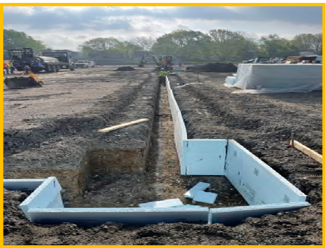
Foam Board Install
