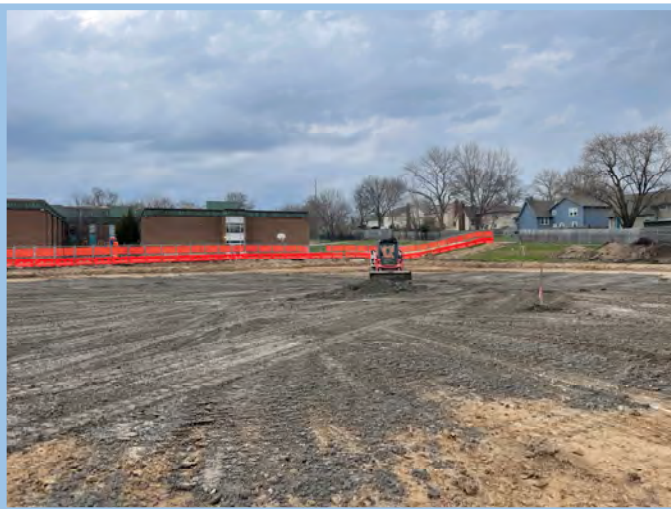
Building Pad Prep
