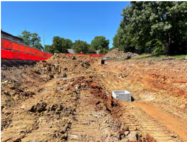
East Storm Sewer Backfilled
