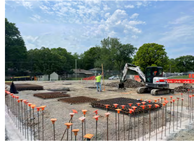
Prep for Spread Footings
