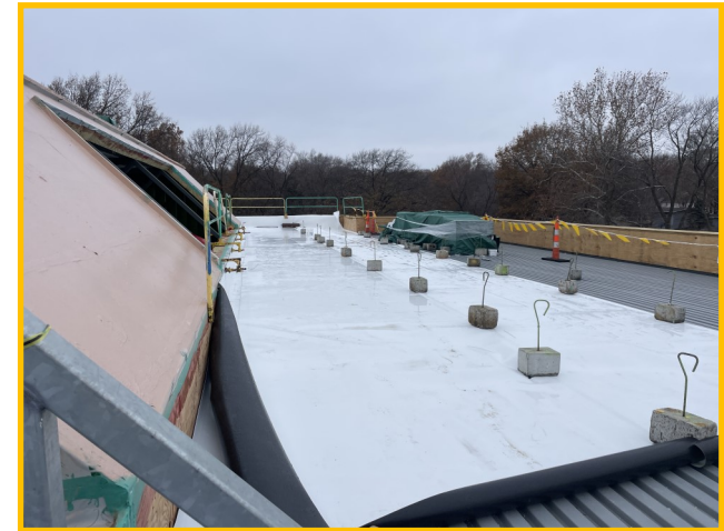
Area B Roofing
