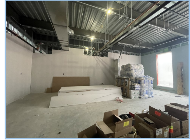
Area B Drywall
