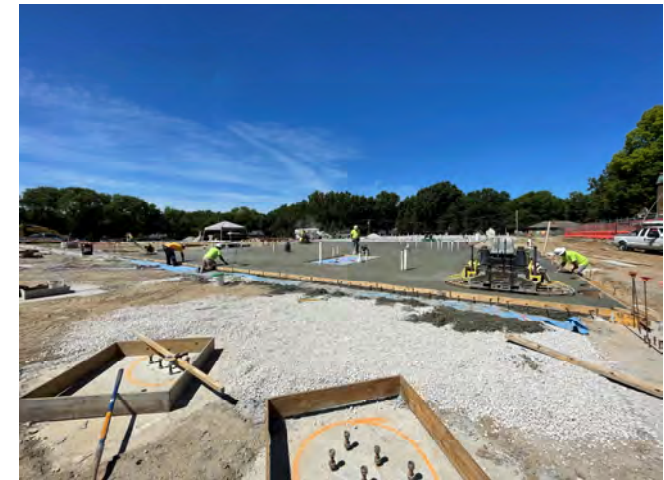
Section 3 Slab on Grade Poured
