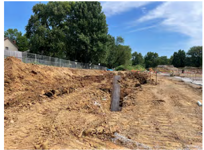
Domestic Water Utility Install
