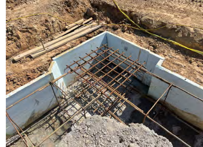
Continued Footing Formwork & Prep
