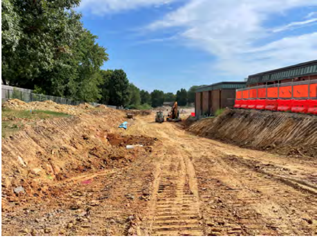
East Side Access Road Graded
