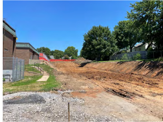
East Side Grading for Storm
