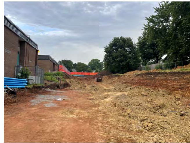
East Side Backfilled to Grade
