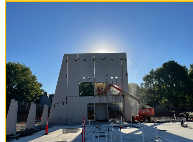
Cleaning All Precast
