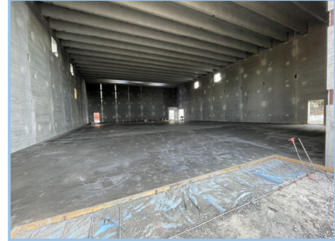
Gym Slab On Grade
