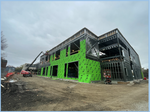
Area B Exterior Framing & Sheathing
