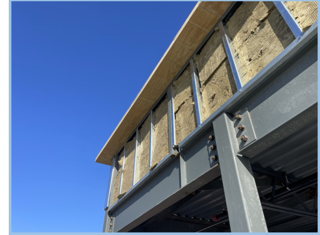
Parapet Blocking
