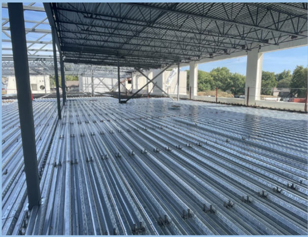
Area B Steel & Decking
