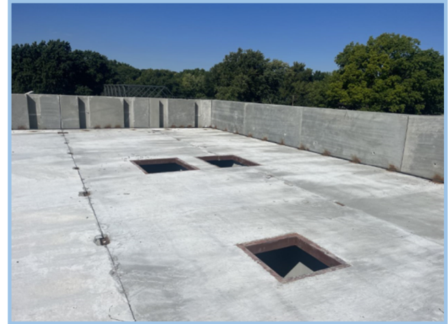
Prep Gym Roof for Unit Curbs
