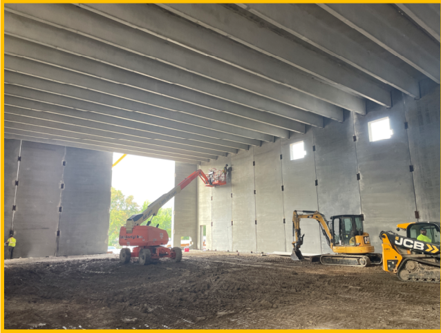
Finalizing Welding Connections
