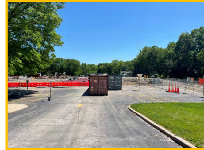
Connex Delivery—Temp Location
