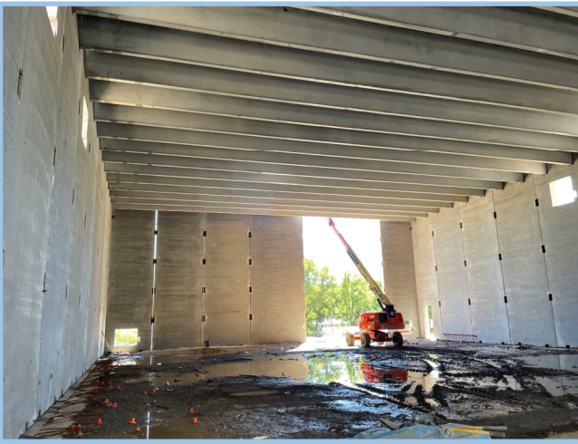
Gym Precast Complete
