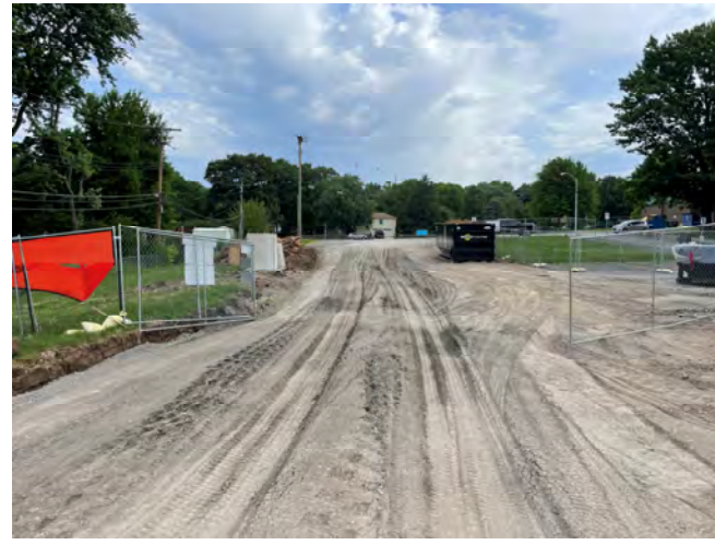
West Entrance Repair On-Going
