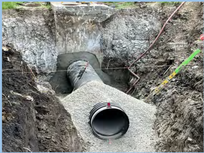
Storm Sewer Install
