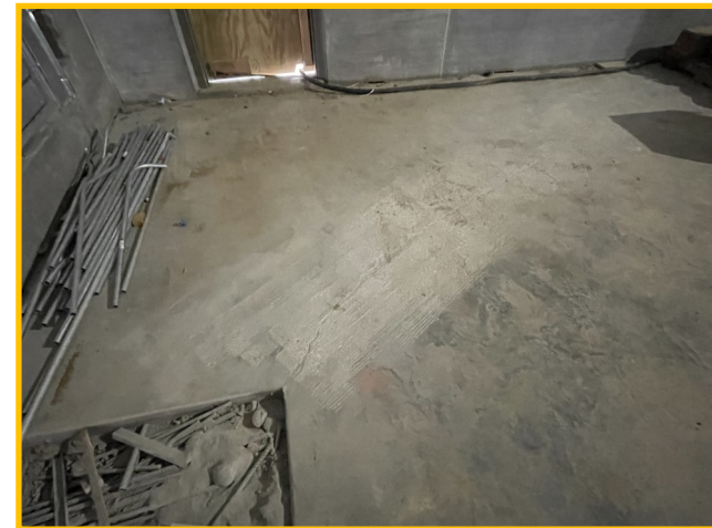
Gym Slab Prep for Wood Floor
