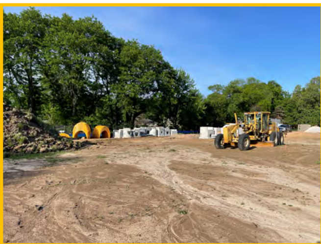
Prep Water Detention Material
