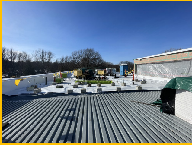
Area B Roofing
