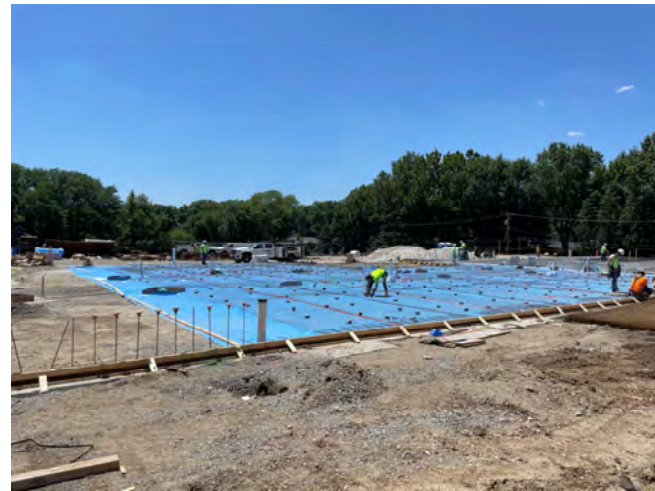
Formwork & Prep for Section 2
