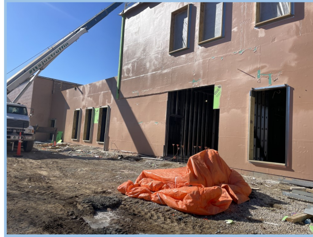
East Air Barrier Install
