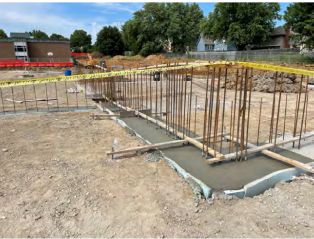
Gym Footings Poured
