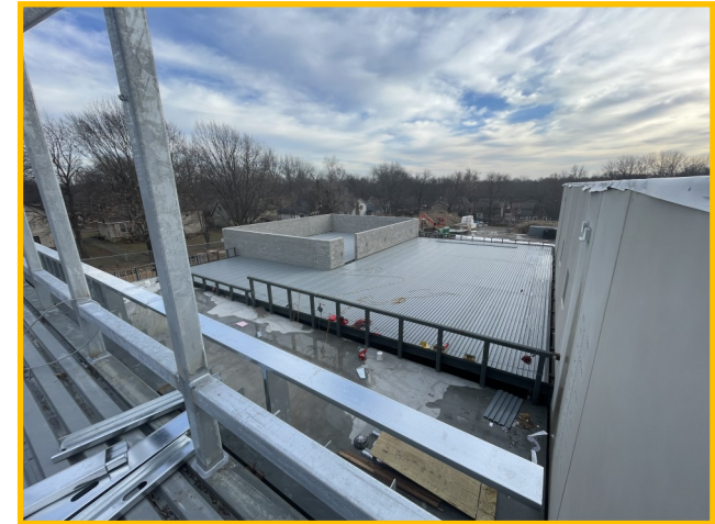
Remaining Steel Detailing
