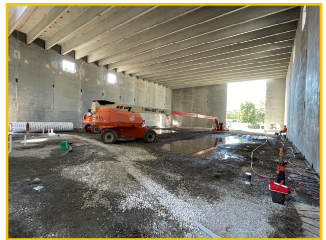
Underground MEP & Slab Prep
