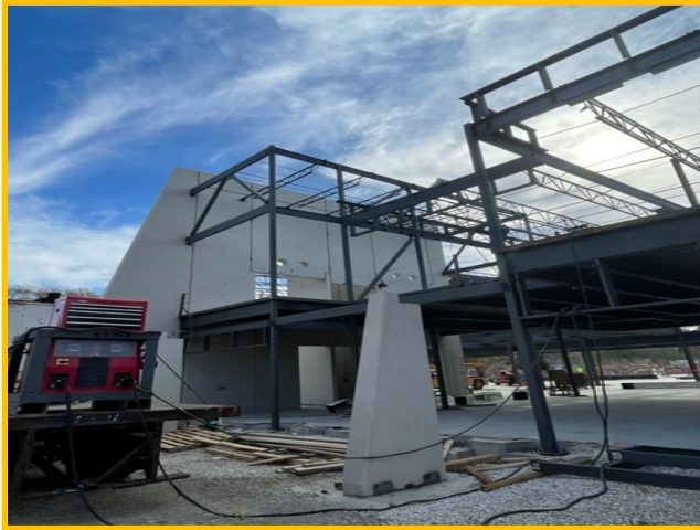
Steel A Steel Erection & Detailing
