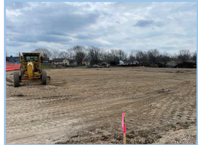
Compaction of Building Pad
