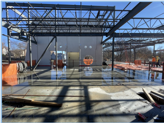
Steel Detailing Prior to Decking
