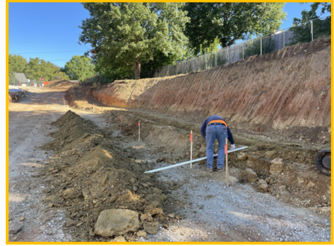
Retaining Wall Layout & Staking
