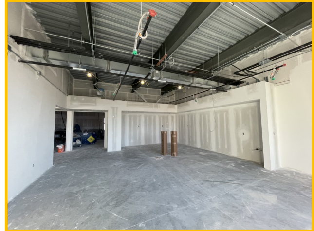
Drywall Finishing In Classrooms
