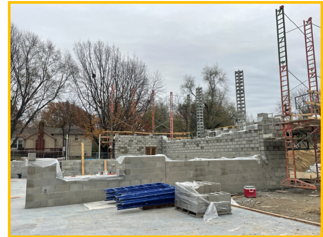
Area A Kitchen CMU Walls
