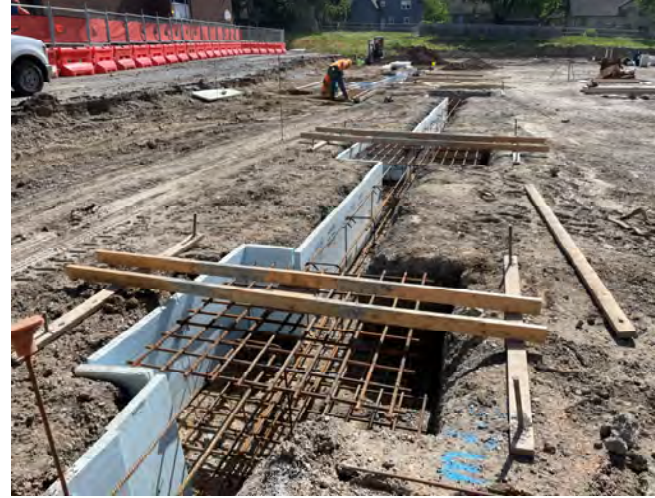
Continued Footing Formwork & Prep
