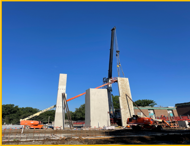
Elevator Core Precast
