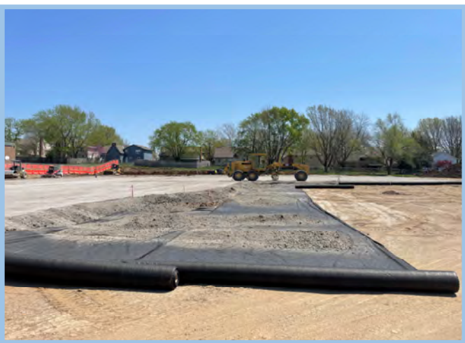
Laydown Filter Fabric
