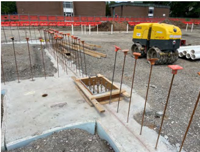
Continued Pouring Footings
