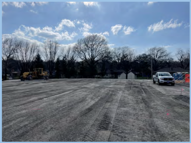
Building Pad Prep
