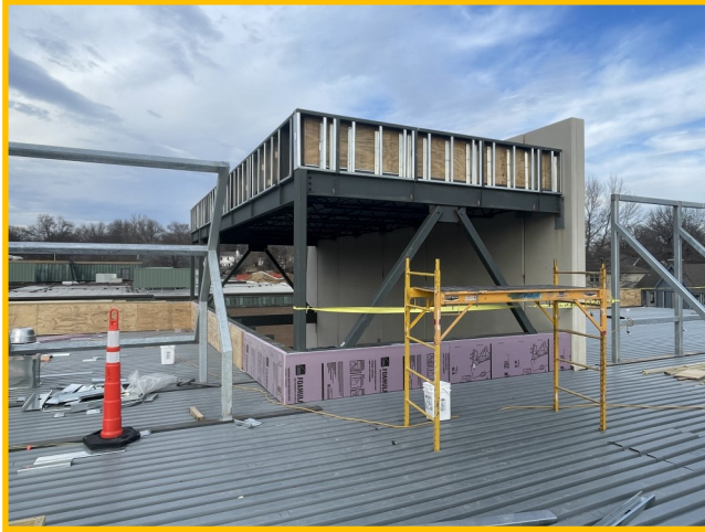
Area A Parapet Blocking
