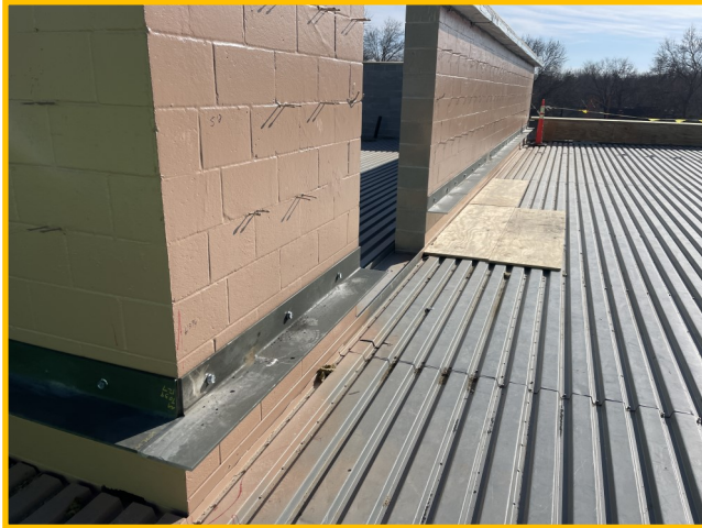
Steel Lintel for Masonry Set
