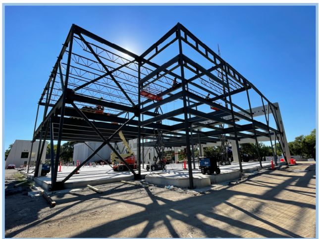
Area B Steel & Detailing
