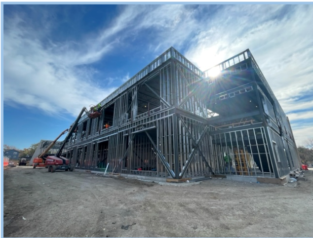
Area B Exterior Framing
