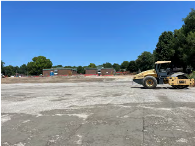
South Side Gravel Laydown
