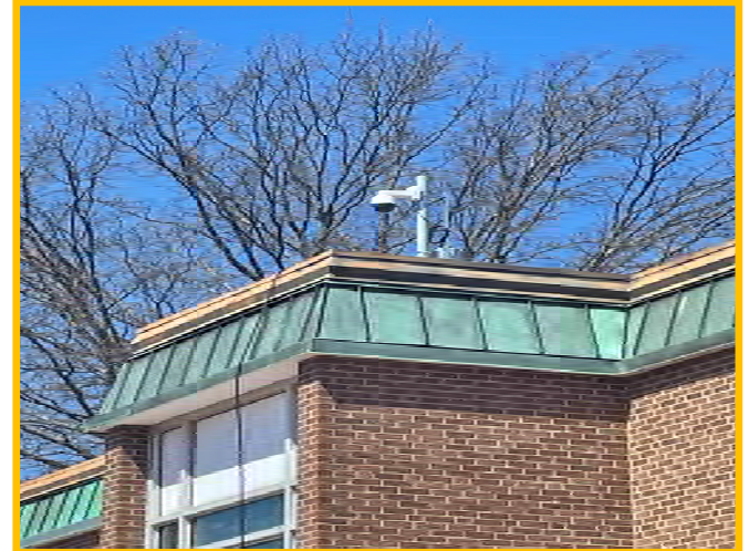
Installed Oxblue Camera
