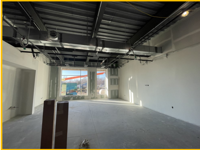
Classroom Drywall Install
