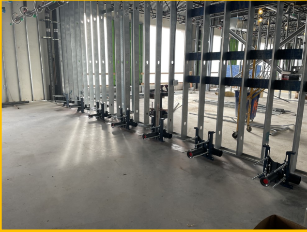
Level 2 Restroom Prep
