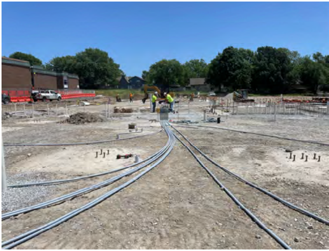
Plumbing & Electrical Underground
