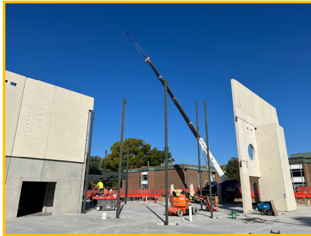
Area A Steel Erection
