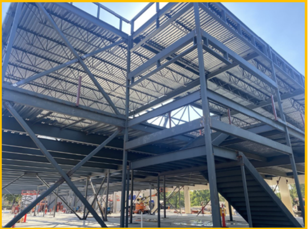
Area B Steel & Decking
