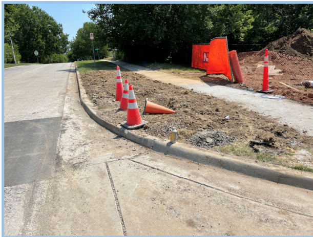
Completed Utility Tie-In
