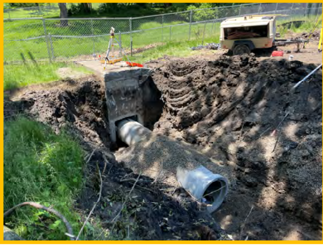
Continued Storm Sewer Install
