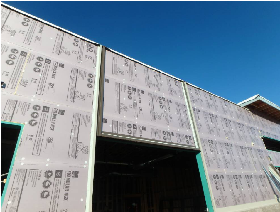
Siding trimwork over the east window of the south classroom
