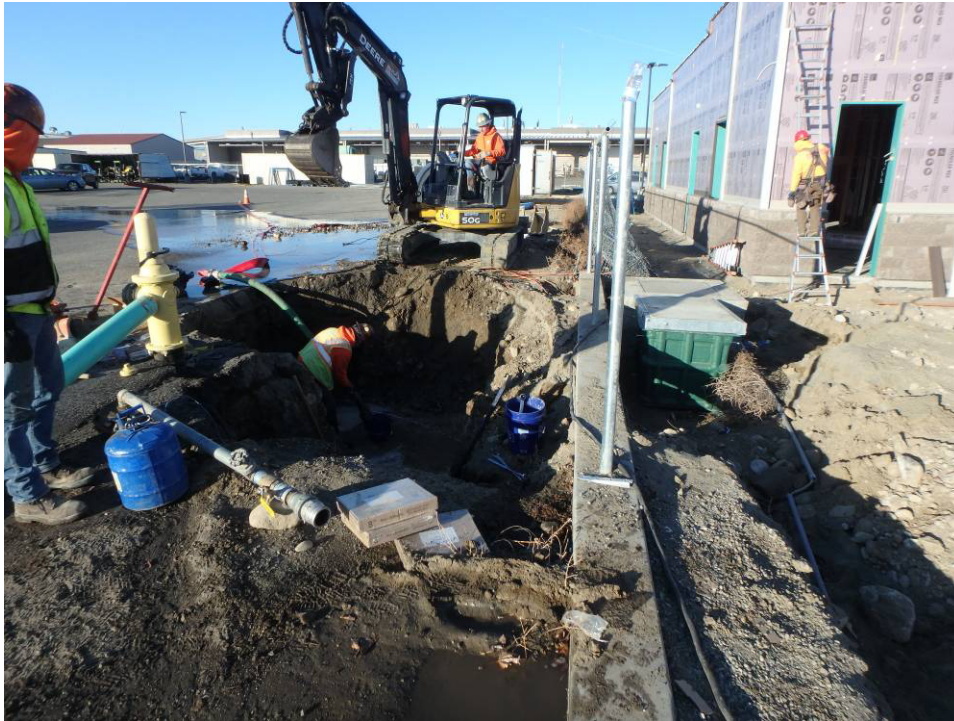
Trenching for the SE water line tie-in
