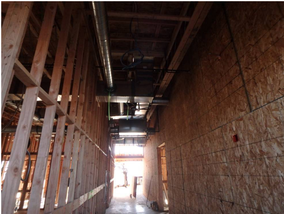
Looking east towards the main entry, new ductwork
