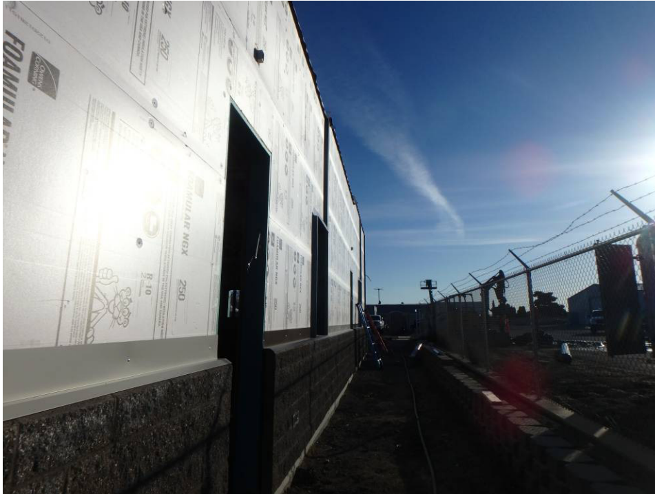
Looking east at the masonry work on the south elevation
