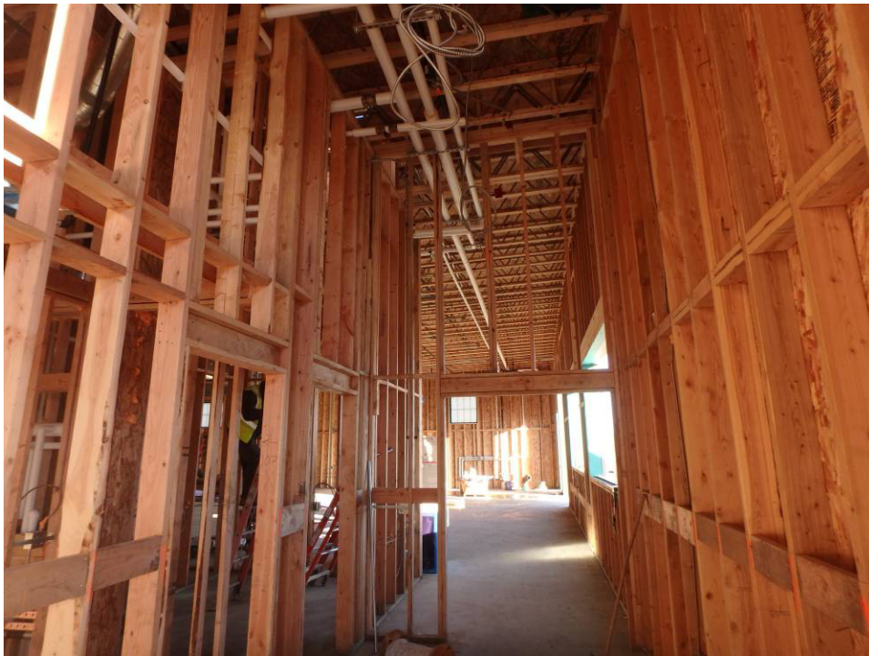
Looking north from the main entry
