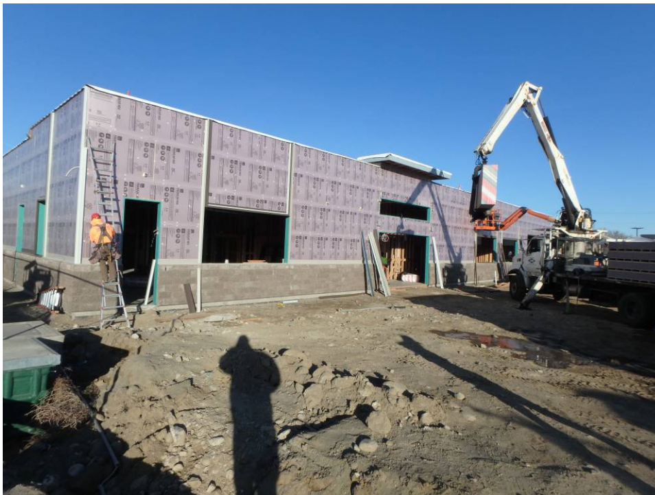
Southeast corner of the building
