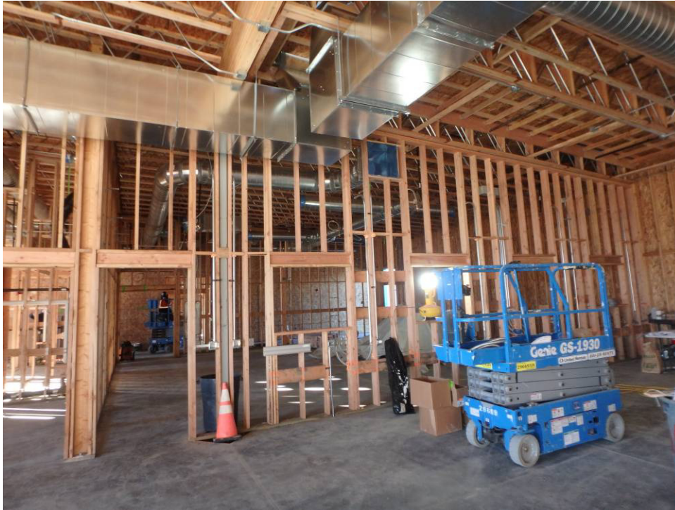
Looking at the south wall of the shop
