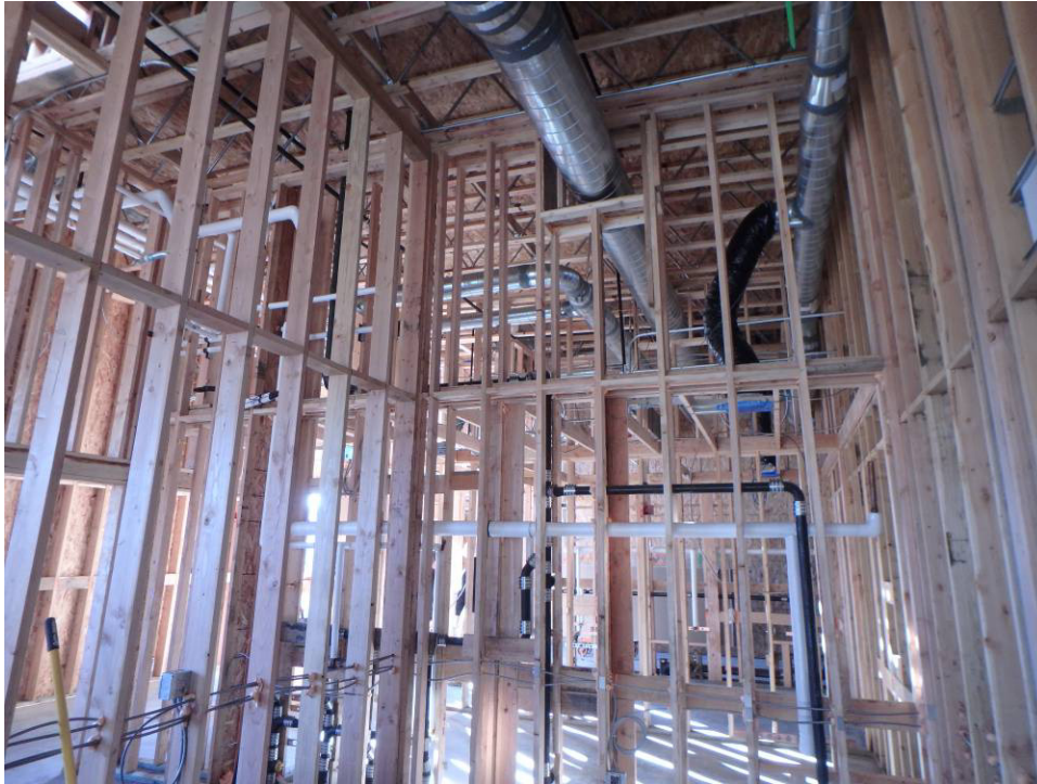
Looking south at the ductwork in the restrooms
