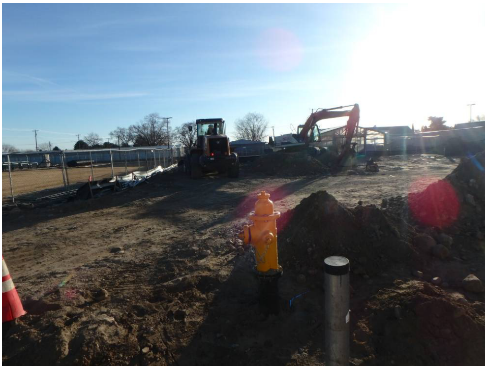
Looking east along the north property line
