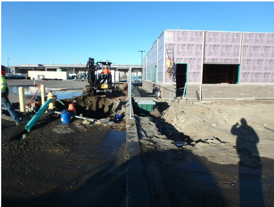
Southeast corner of the building, insulation board and masonry
