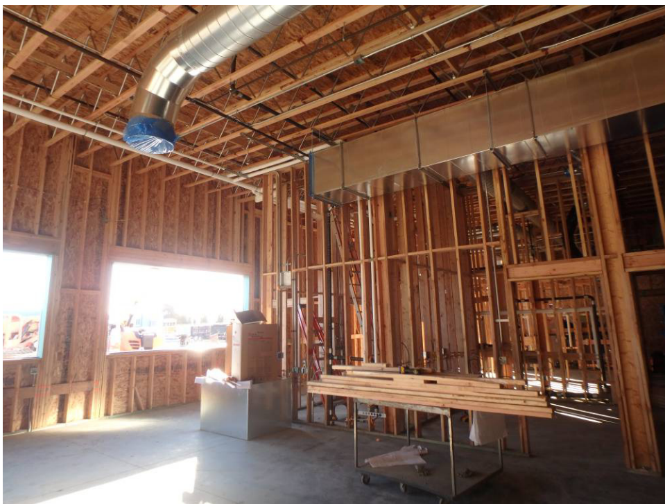
Looking at the southeast corner of the shop
