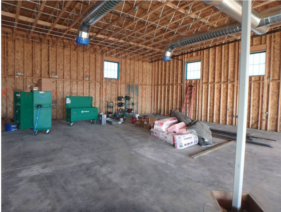
Looking at the northwest corner of the shop
