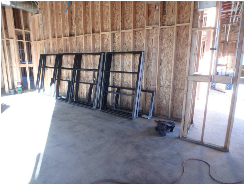
Delivered storefront frames
