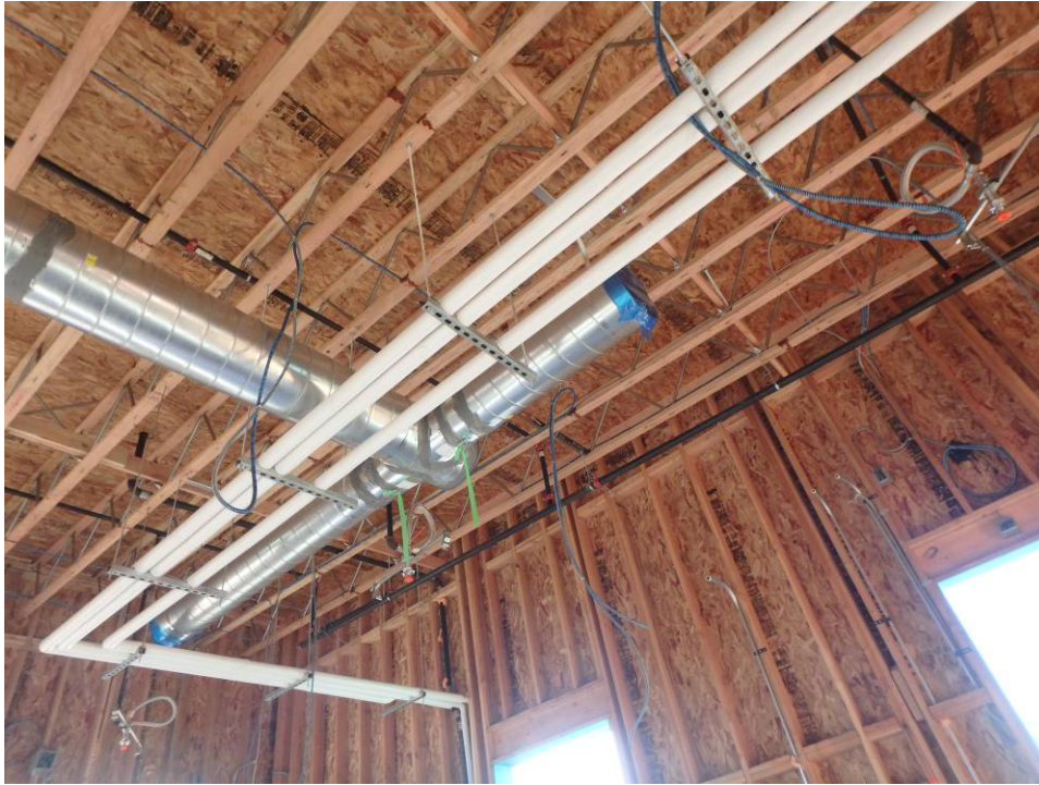
Ductwork over the south wall of the south classroom
