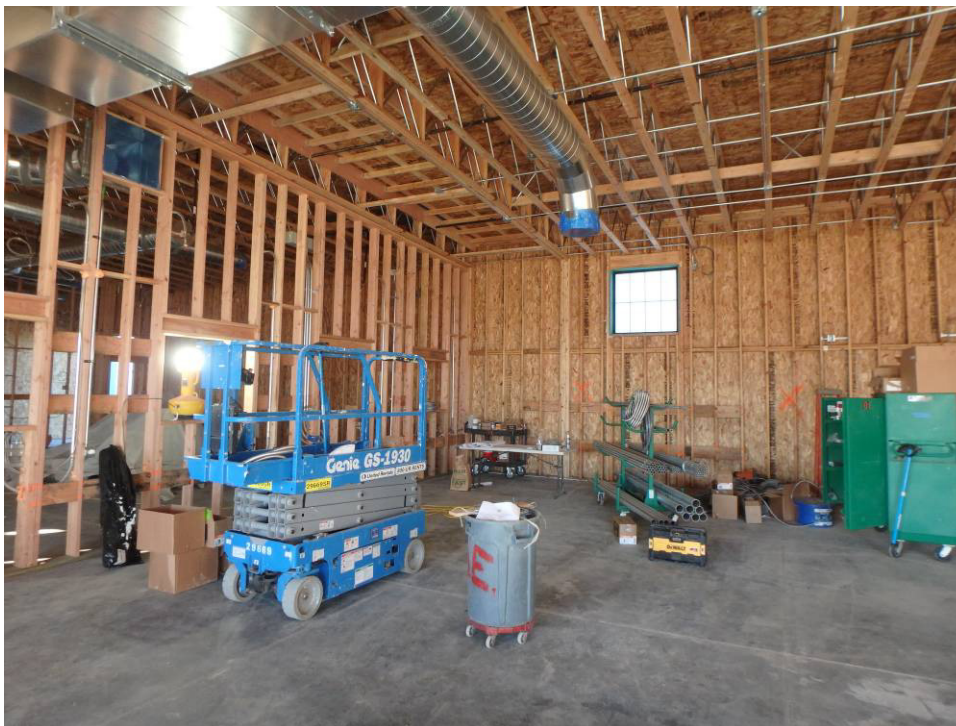
Looking southwest across the shop
