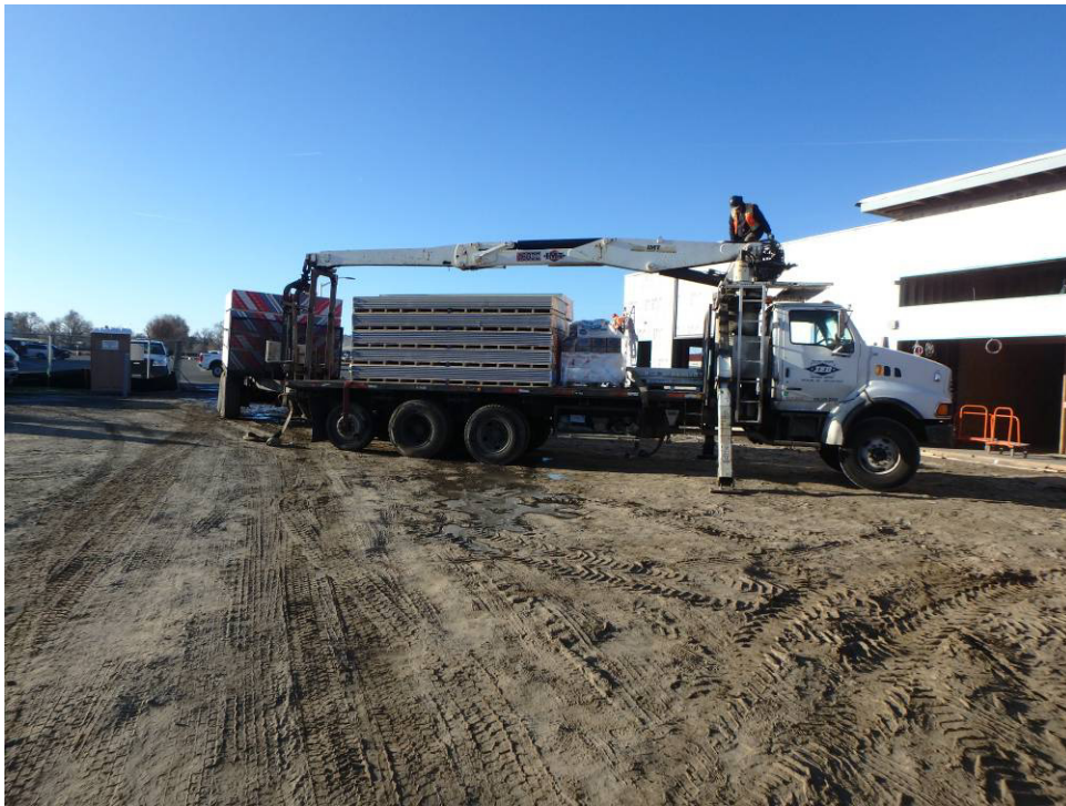
Unloading gypsum wallboard
