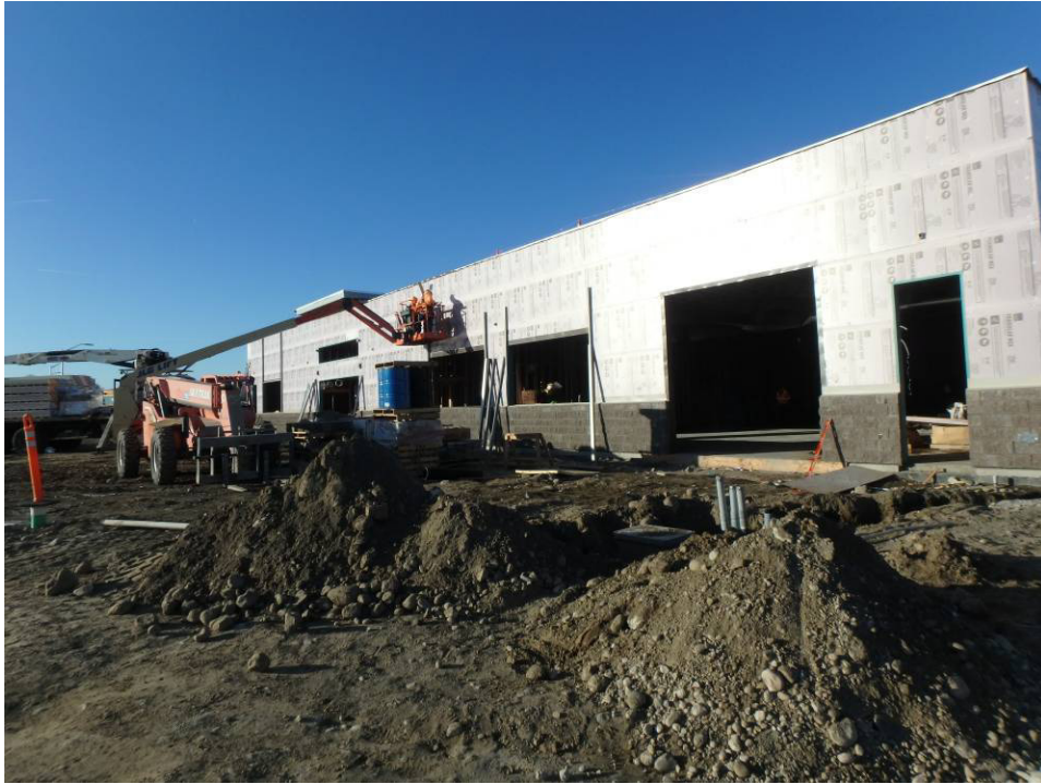
East elevation, installing trim parts for the siding
