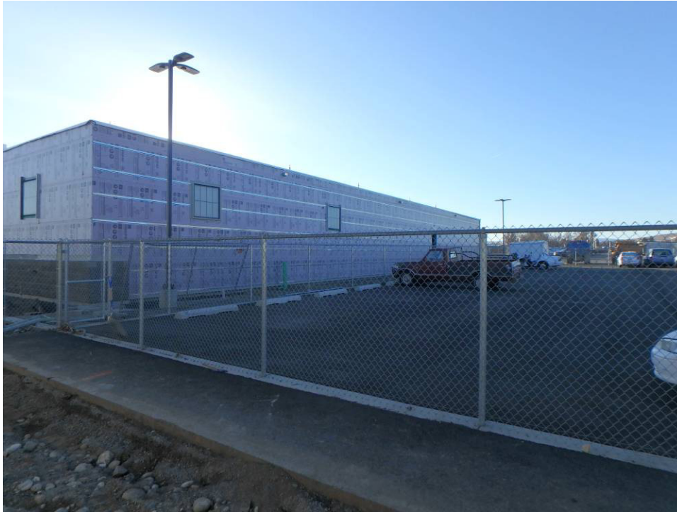
West elevation insulation board and siding furring
