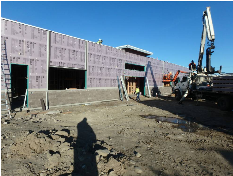
East elevation and the main entry
