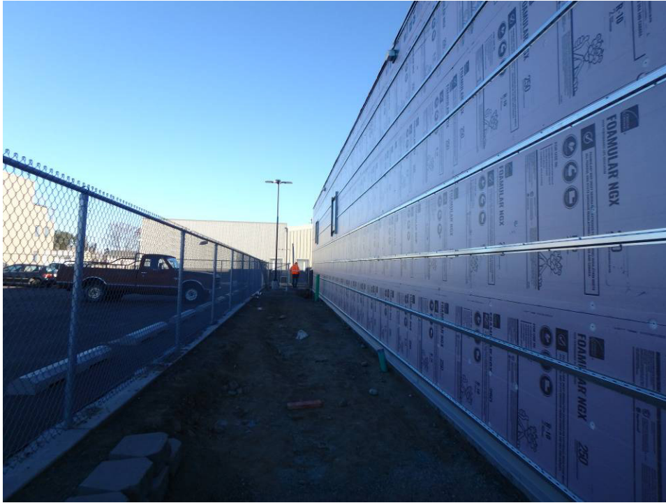
Looking north at the west elevation insulation board
