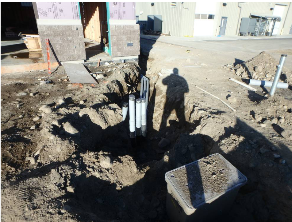
Conduit stub-ups in the NE landscape island
