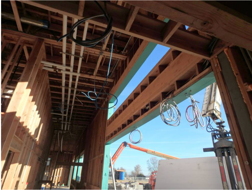
Entry framing and wiring
