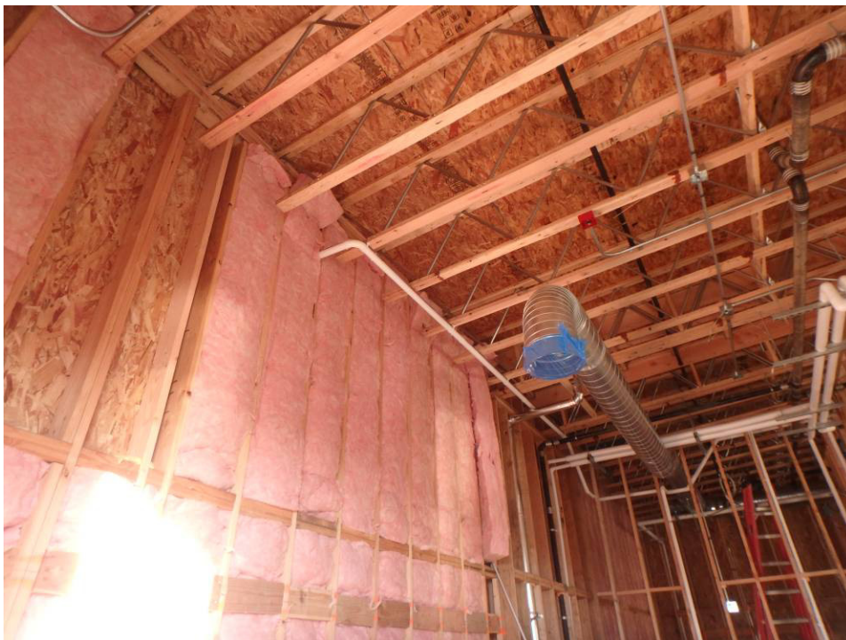
Wall insulation in the south end of the west wall
