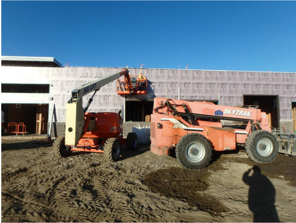
Installing siding trim on the east elevation
