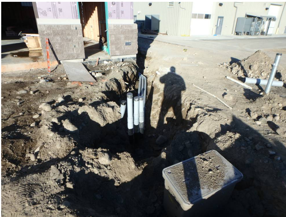
Conduits stubbed up in the NE corner of the building
