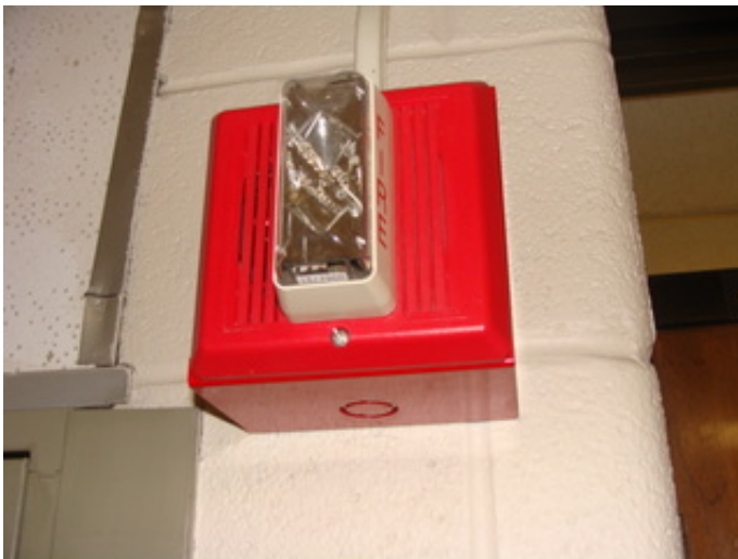
Typical Horn/Strobe Unit
