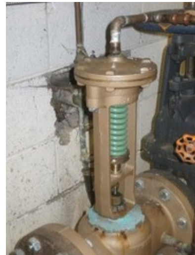
Domestic Water Pressure Regulating Valve
