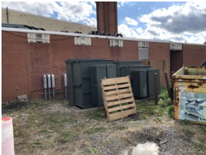
Two pad mounted transformers
