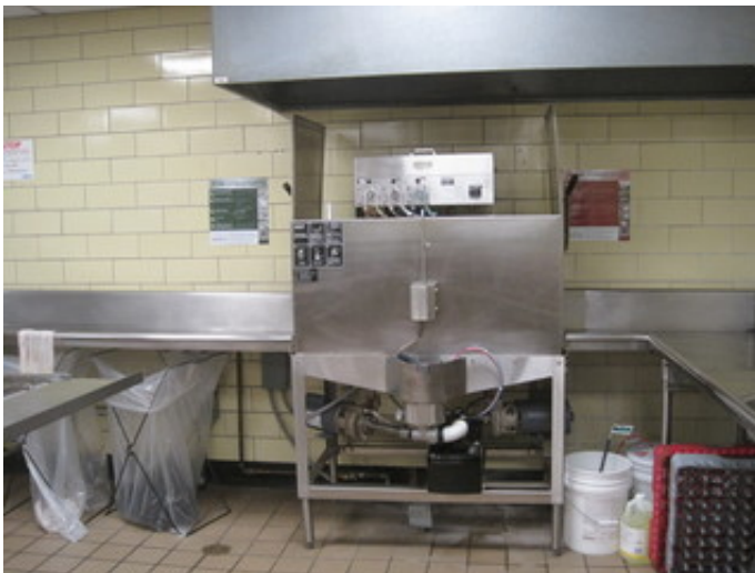
Grease Waste Interceptor Below Dishwasher
