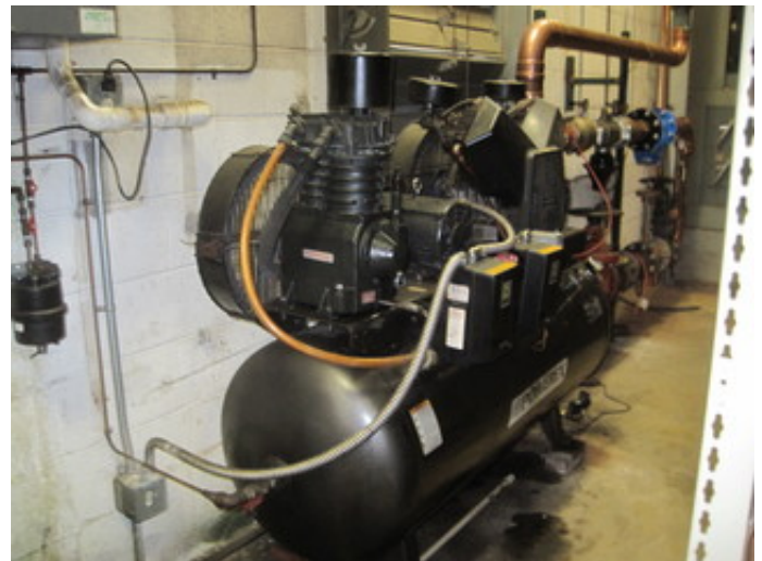
Temperature Control Air Compressor
