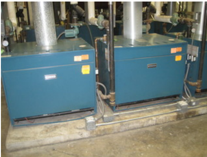
Heating Water Boilers
