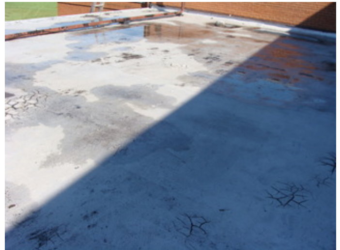
Standing Water on Adhered Membrane
