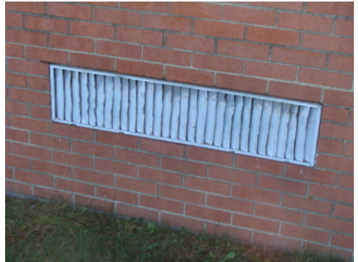
Unit Ventilator to Be Filled In
