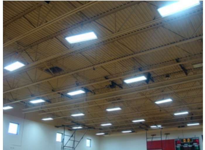
Steel Joists over Gym
