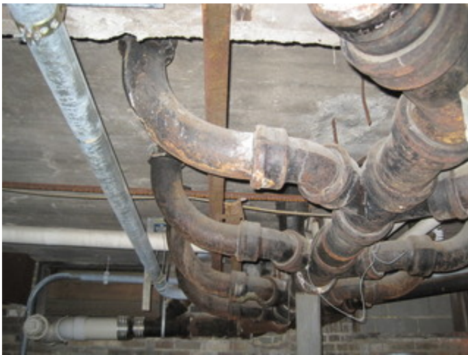
Cast iron sanitary piping
