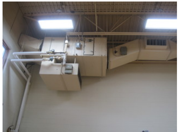
Gymnasium heating & ventilating AHU
