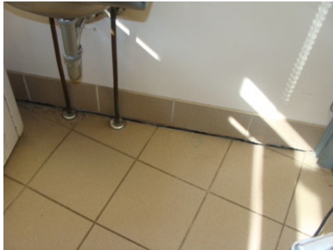
Interior Floor Settlement Issue That Is Currently Being Repaired
