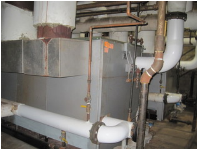
Steam heating boilers
