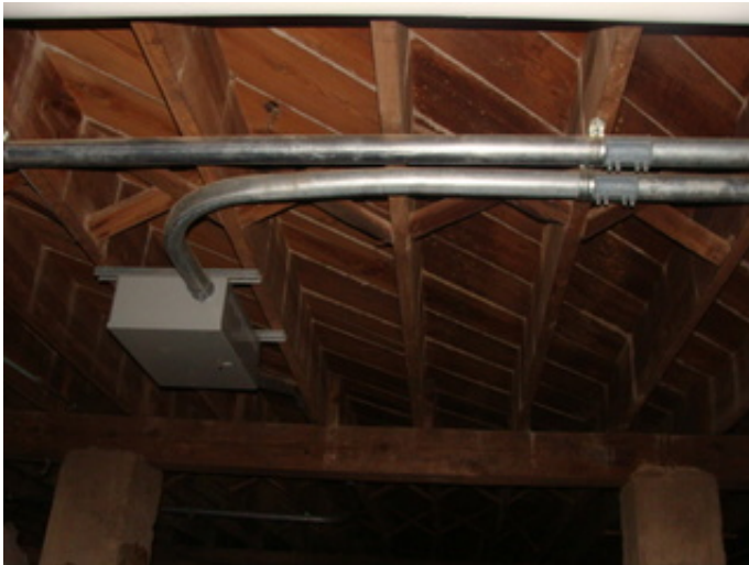
Wood Structural Framing Under Cafeteria
