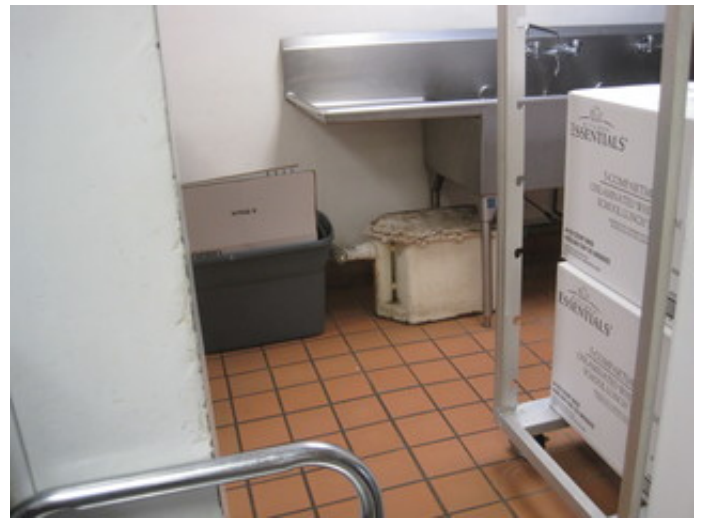
Grease Waste Interceptor
