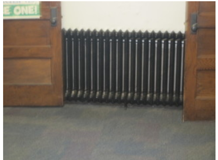
Steam cast iron radiator
