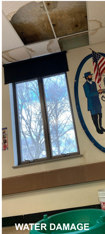
WATER INFILTRATION IN GYM
