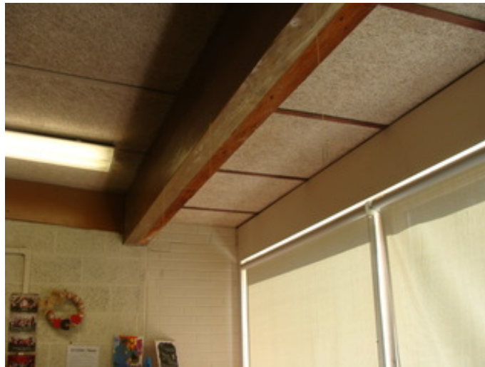
Area Where Exterior Wall Needed To Be Relocated
