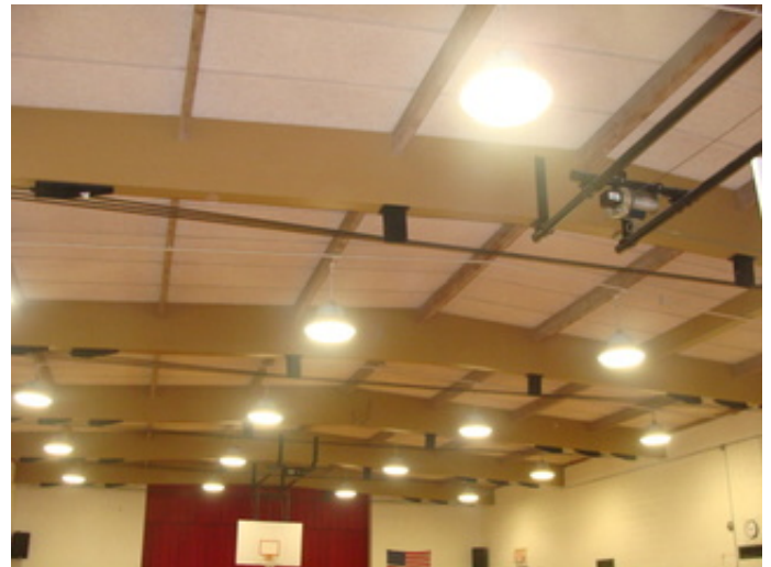
Wood Roof Trusses in Gymnasium
