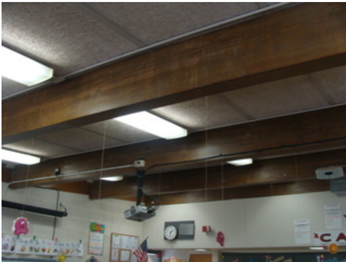
Wood Roof Beams in Classroom
