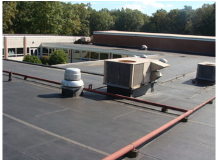
Existing EPDM Roofing
