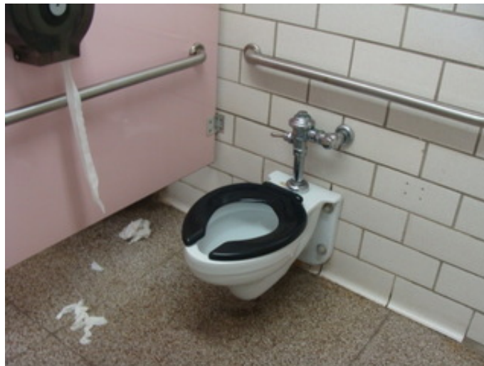
ADA wall-mounted toilet
