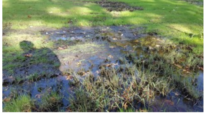
Severe Ponding Areas Behind Building
