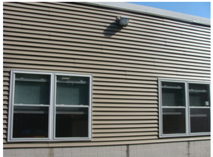
Typical Classroom Windows
