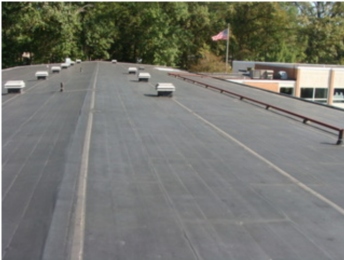
Existing EPDM Roofing
