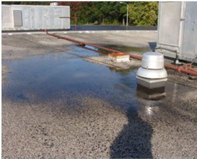
Northeastern Ohio weather elements have taken a toll on our aging exterior building envelope systems, such as roof and exterior masonry facades, allowing for air and water infiltration.
