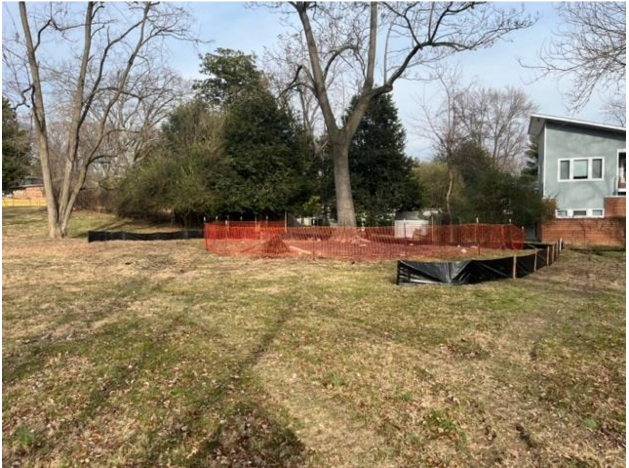
Figure 3: Sediment and erosion control silt fencing
