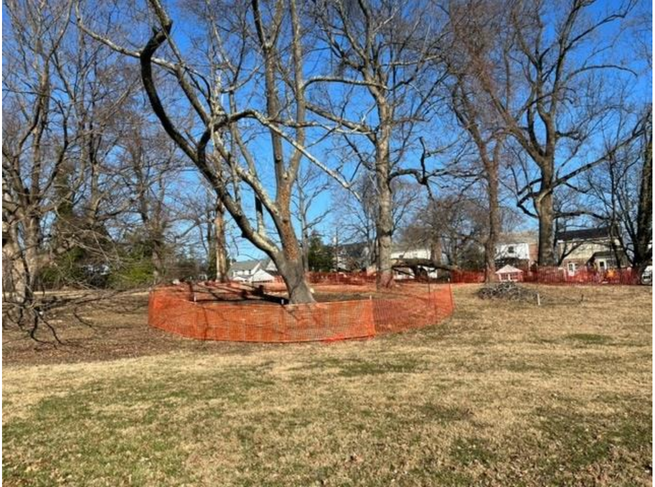
Figure 2: Heritage critical root zone protection fencing
