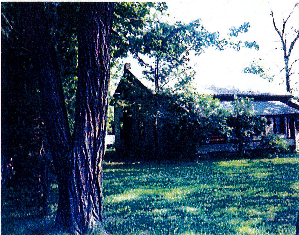
Mr. Flemming and later Mr. Frederick's home corner of Wadsworth and Lisbon Street
