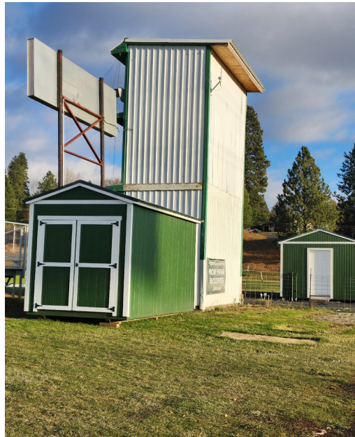
New storage shed at PHS football field.
