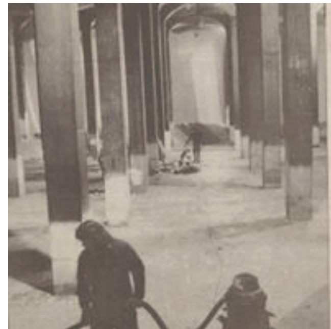
CLEANING THE INTERIOR OF THE OLD MOUNT TOM STORAGE TANK (CIRCA 1990)
