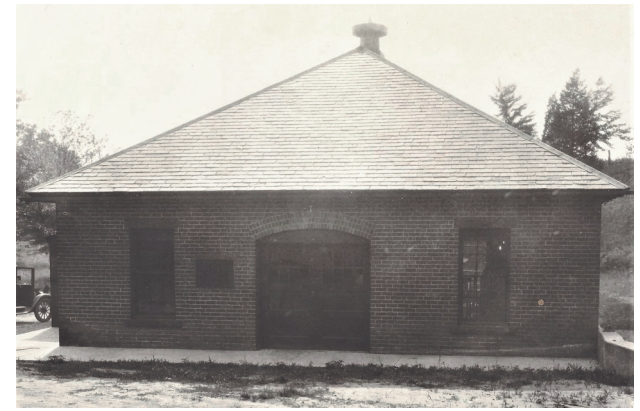
HENDRICK STREET PUMPING STATION CIRCA 1915
