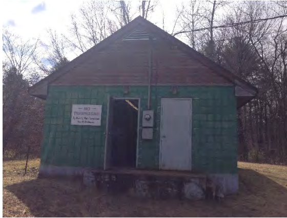
Figure 4-12. Gilbert Road Station – Exterior
