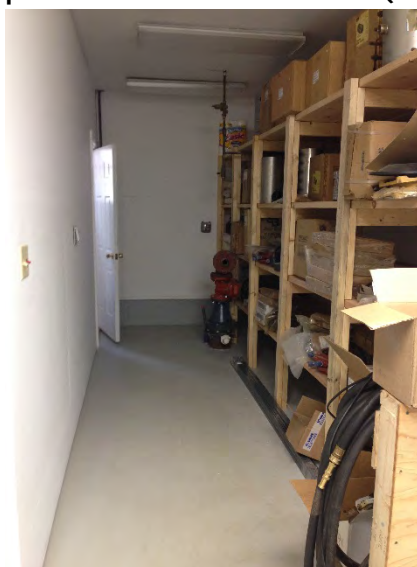
Figure 4-11. Pequot Road Station – Interior (Former Pipe Area)
