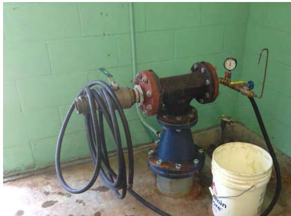
Figure 4-14. Gilbert Road Station – SWD Sample Station
