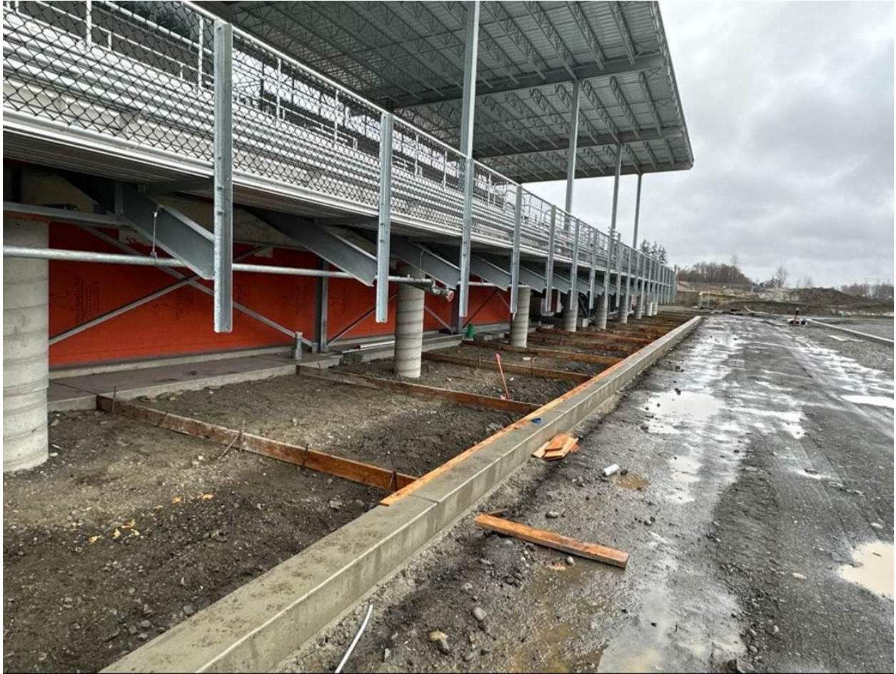
The concrete barrier between the track and the Grandstands is now installed
