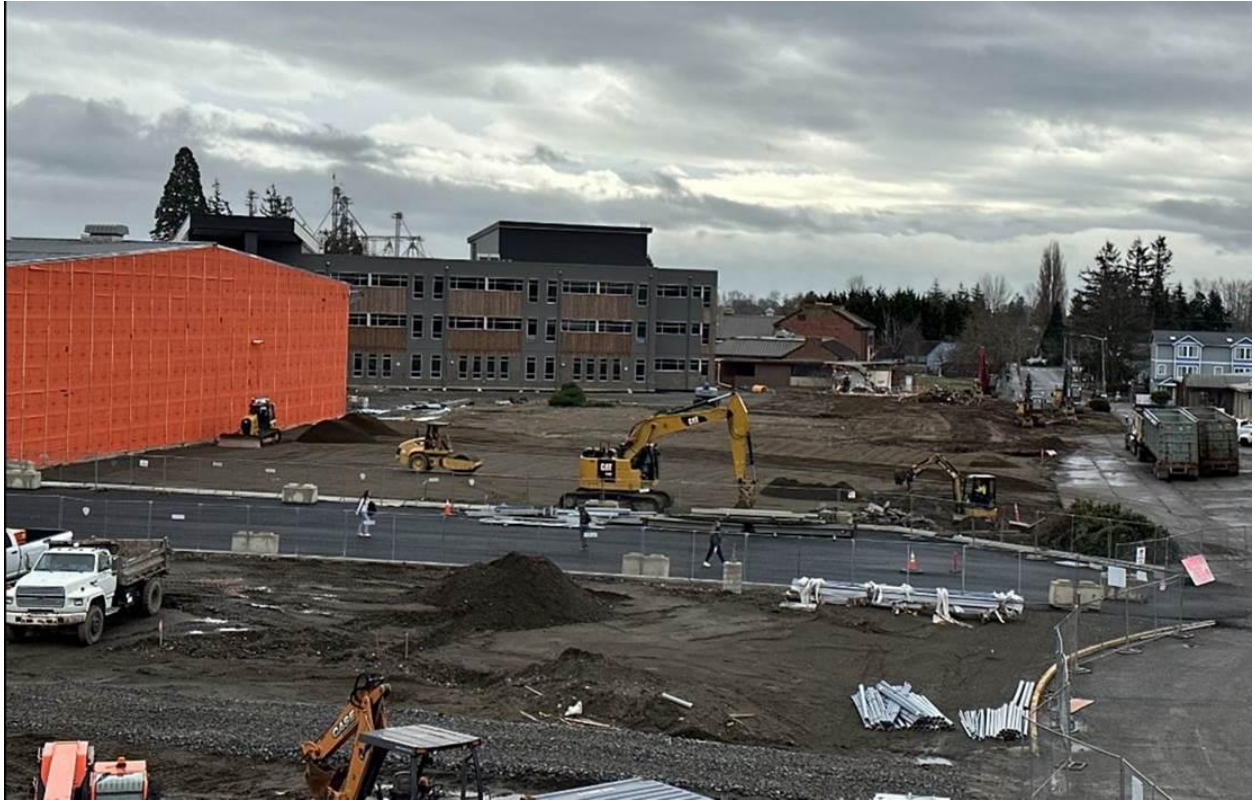
Now that the old building is gone, crews are preparing the pad for the CTE Wing
