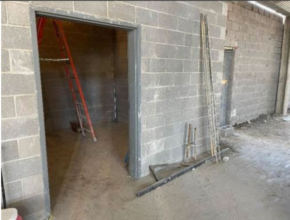
Masonry walls with hollow metal door frames
