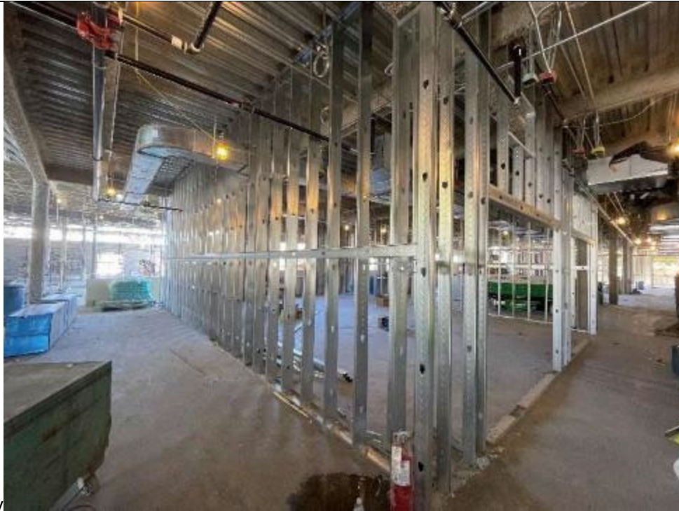
Metal stud framing at area C
