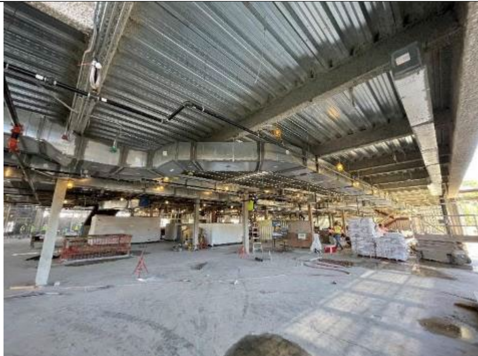
Ductwork installation area C
