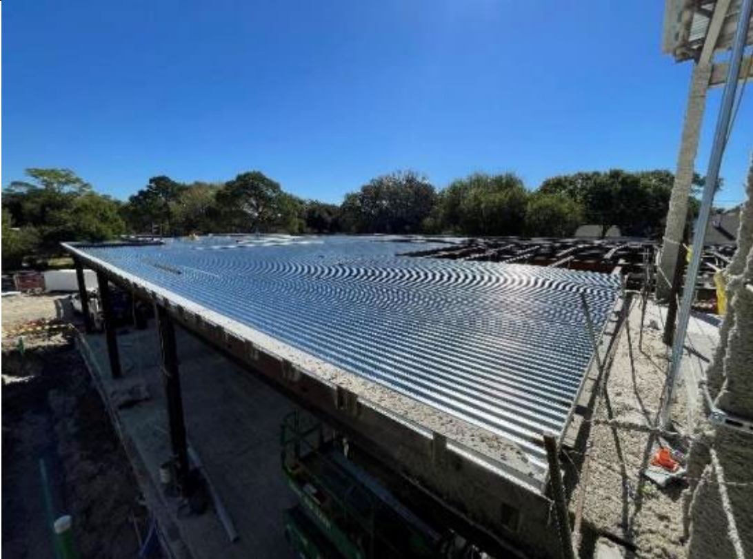
Metal deck at area A
