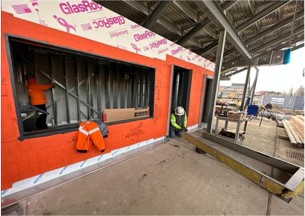
Exterior work around the Grandstand concessions area
