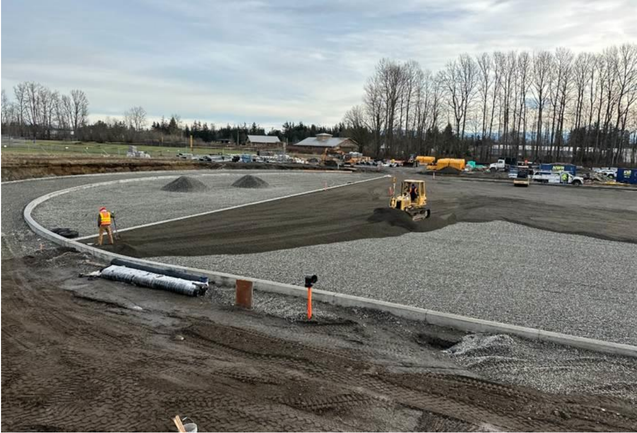
Final gravel being installed on the football field
