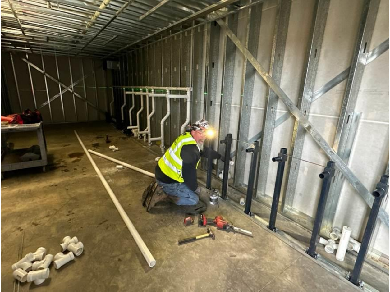
Plumbing being installed in the Grandstand bathrooms
