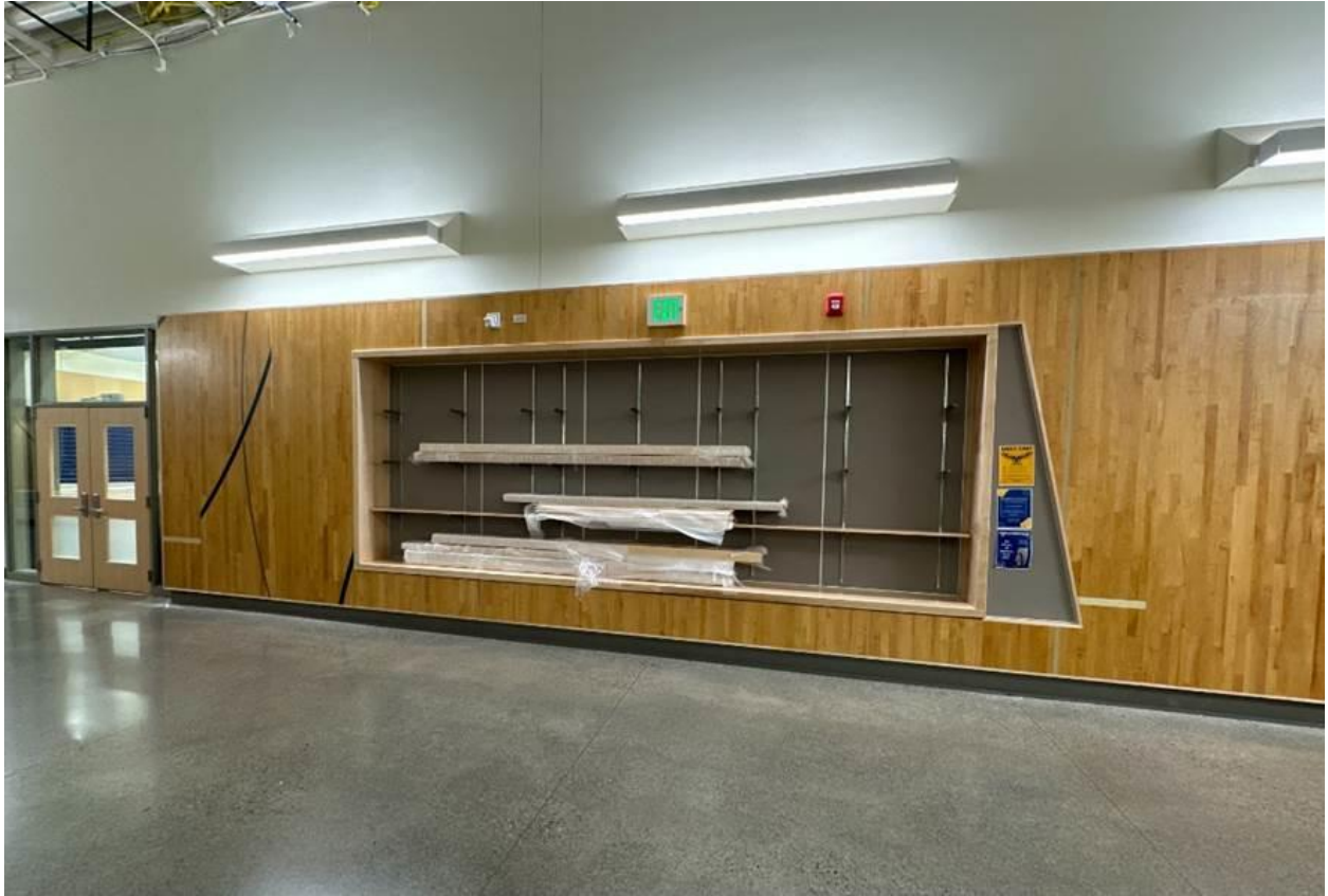
Reclaimed flooring from the old gym installed around Athletic Wing display case
