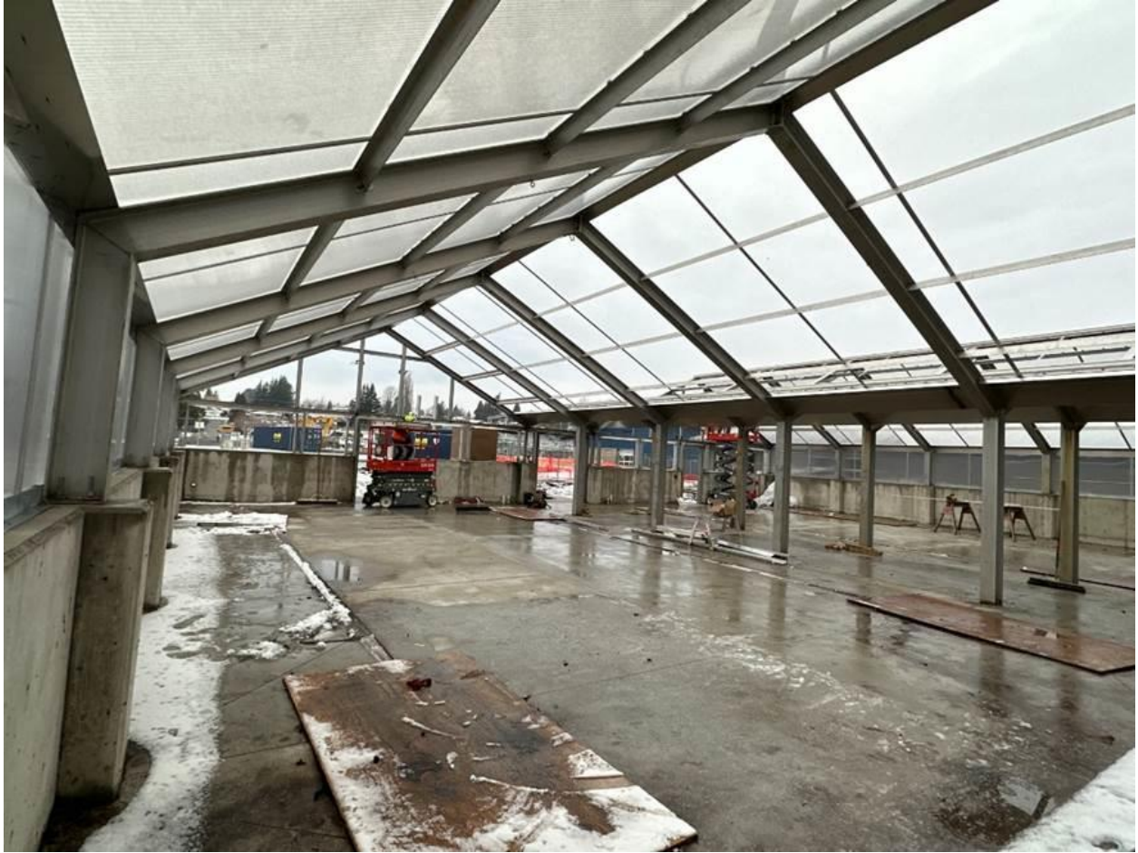
Greenhouse plexiglass panels being installed
