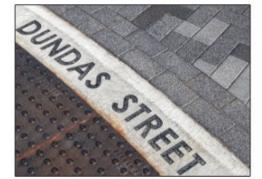
Detectable Warning Pavers - Subtle Wayfinding Specialty Interlocking Unit Pavers - Warm Tone
