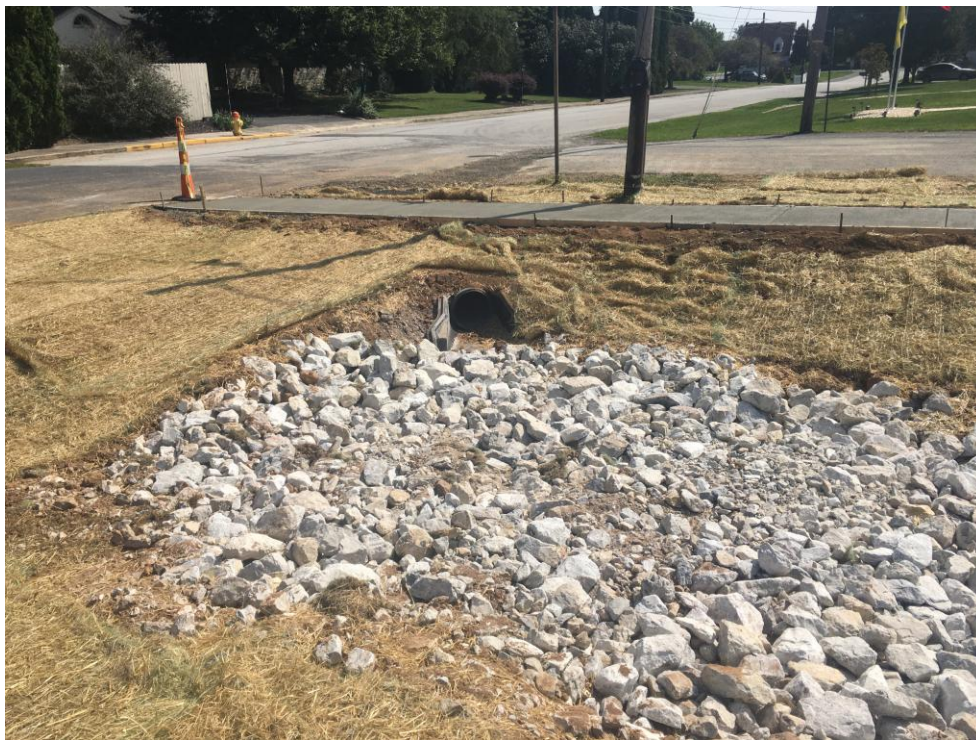
View of riprap outlet to Fohl St. inlet; note new sidewalk.
