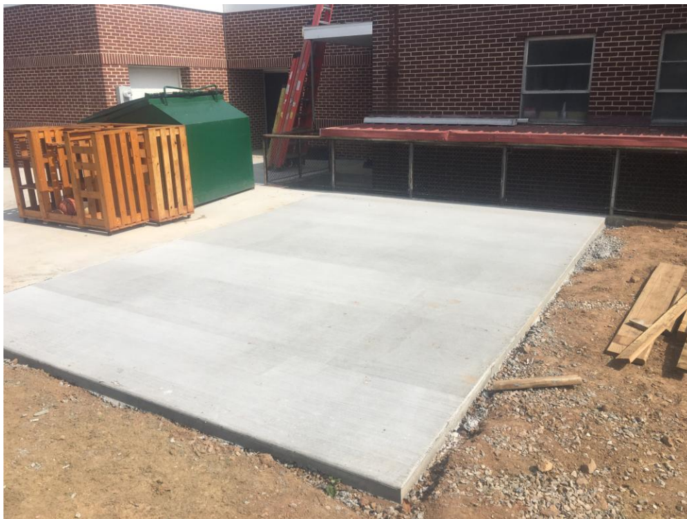
View of new concrete pad for shed.
