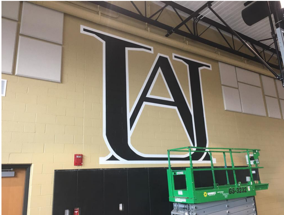
View of new logo being applied to Gym wall..
