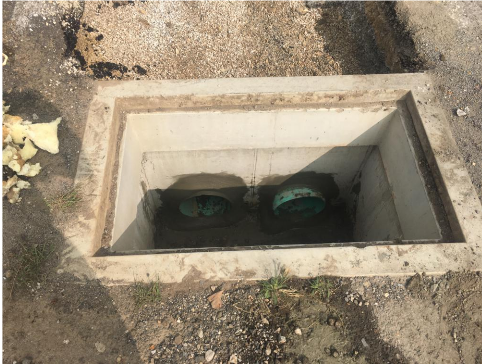
View of Fohl St storm inlet on south side of street.
