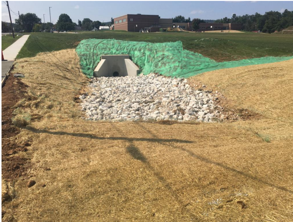
View of new end wall for Fohl St. storm water piping.
