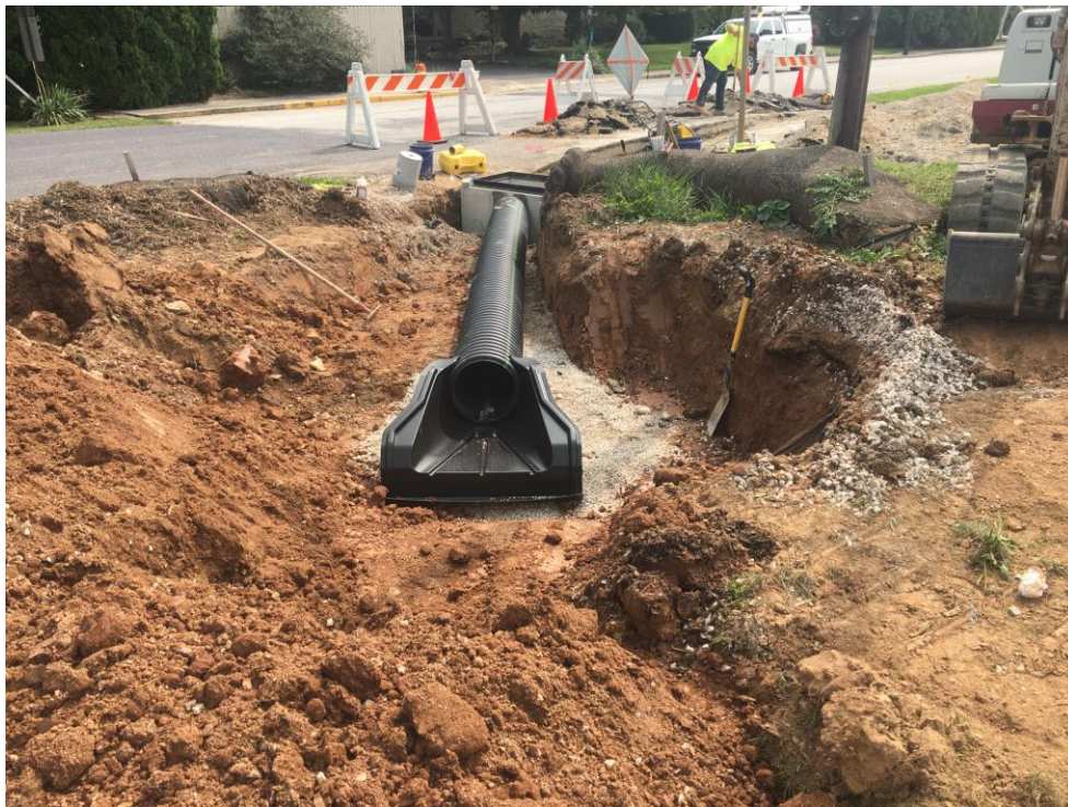
View of inlet pipe from District property to street inlet on Fohl St.
