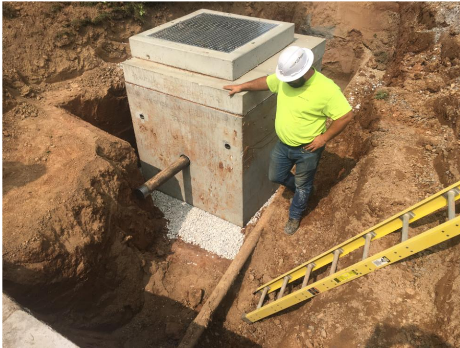
Water Meter pit being installed.
