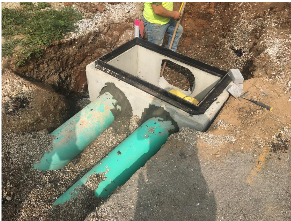
View of Fohl St storm water piping being installed.
