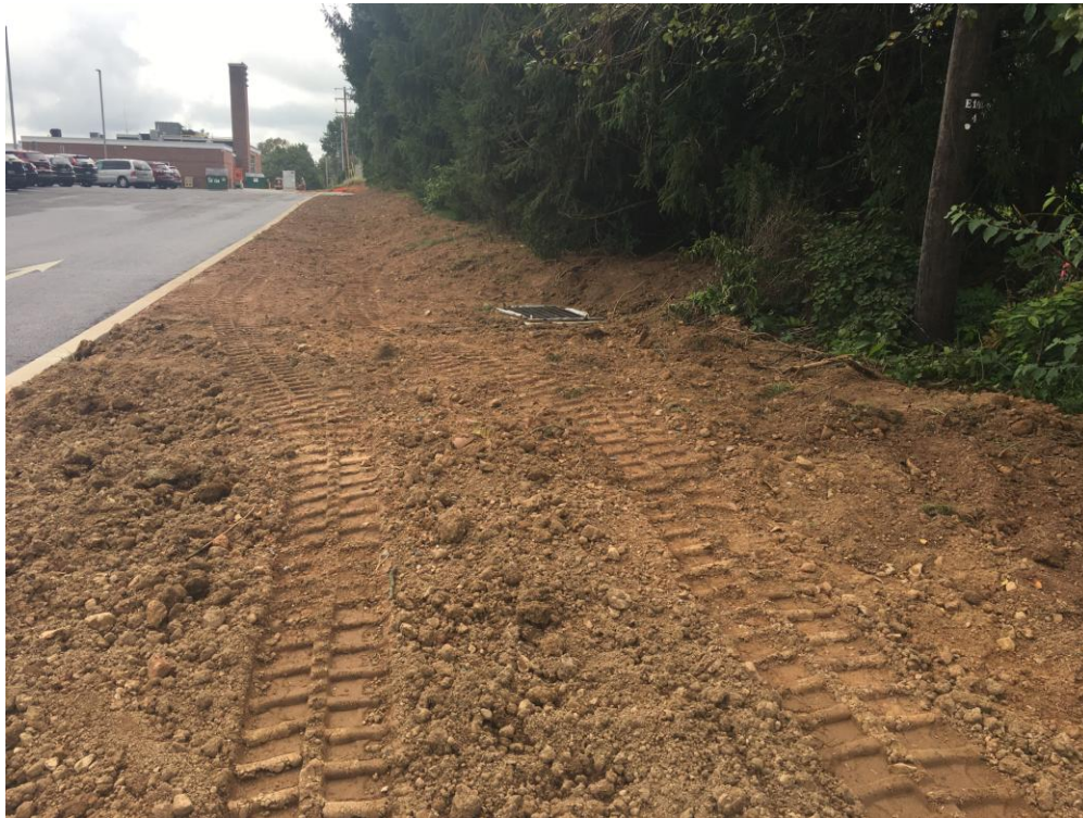
View of Channel 1 at rear parking lot.
