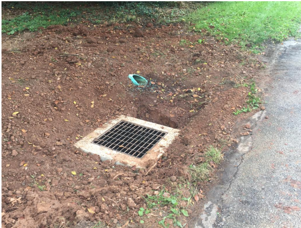
View of catch basin required by Borough for sump pump outlet.
