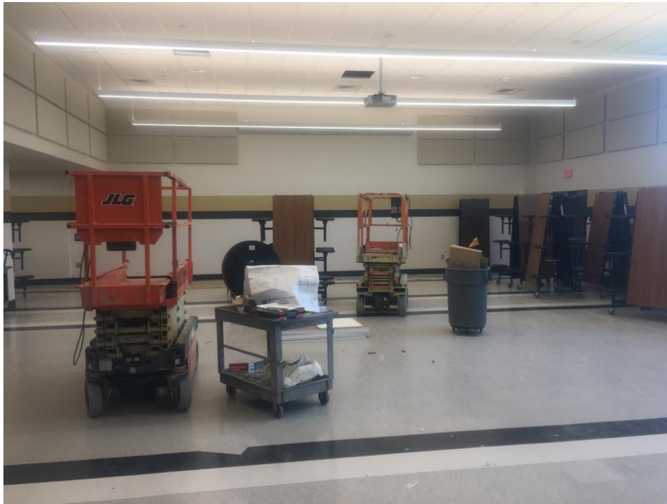
View of completed Cafeteria lighting.
