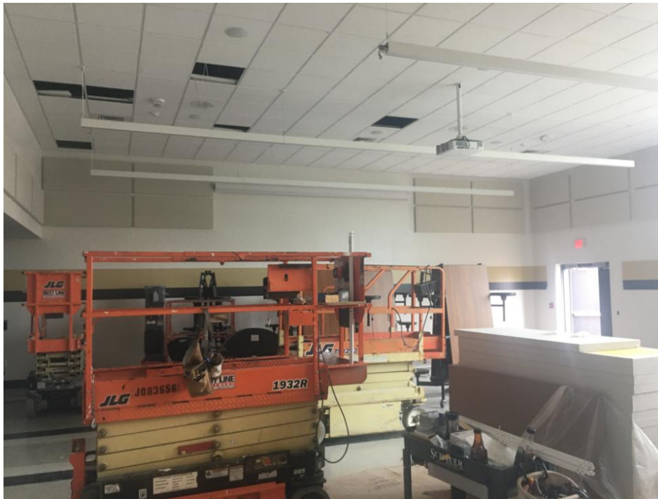
Lighting and acoustic panels being installed in the Cafeteria.
