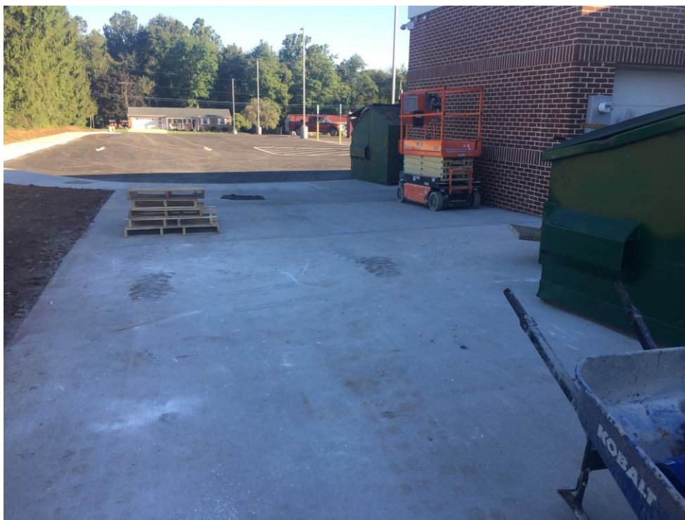
View of completed trash pad at rear of Kitchen.
