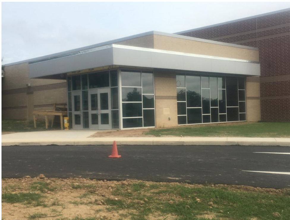
View of fascia being completed at Gym entrance.
