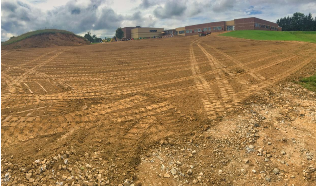
Panoramic view of topsoil and grading on Queen St side.
