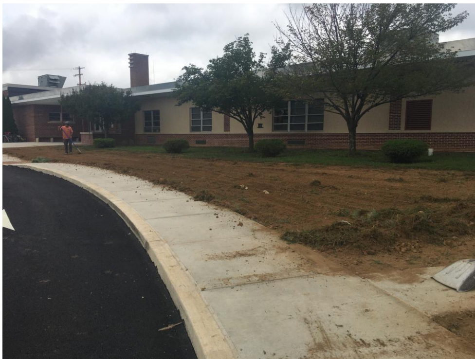
View of landscaping and cleanup starting at front of building.
