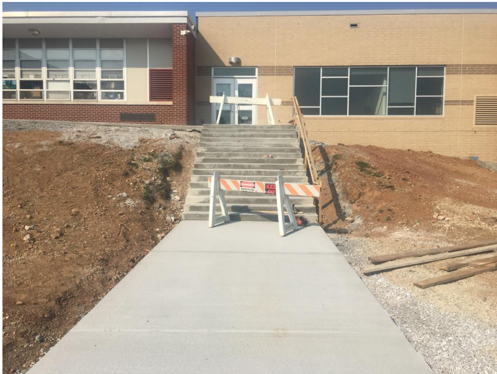
View of new playground steps with temporary railing installed.
