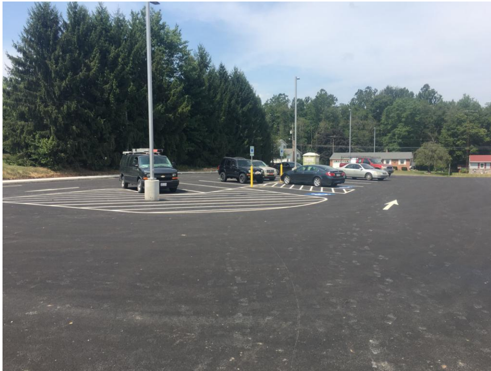
View of rear parking lot after lining.
