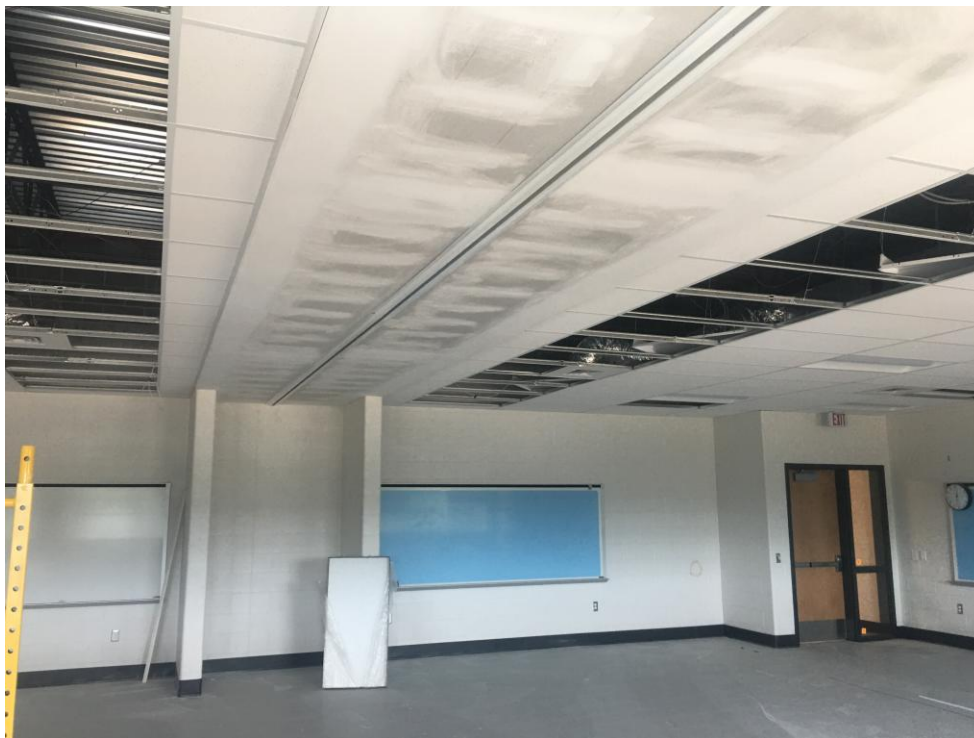
View of completed soffit and partition track in LGI.
