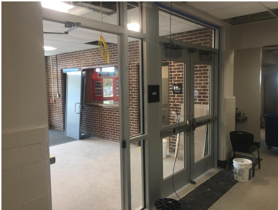
View of new entrance doors being installed.
