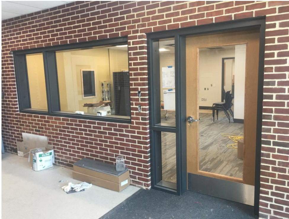
View of new Admin Office entrance.
