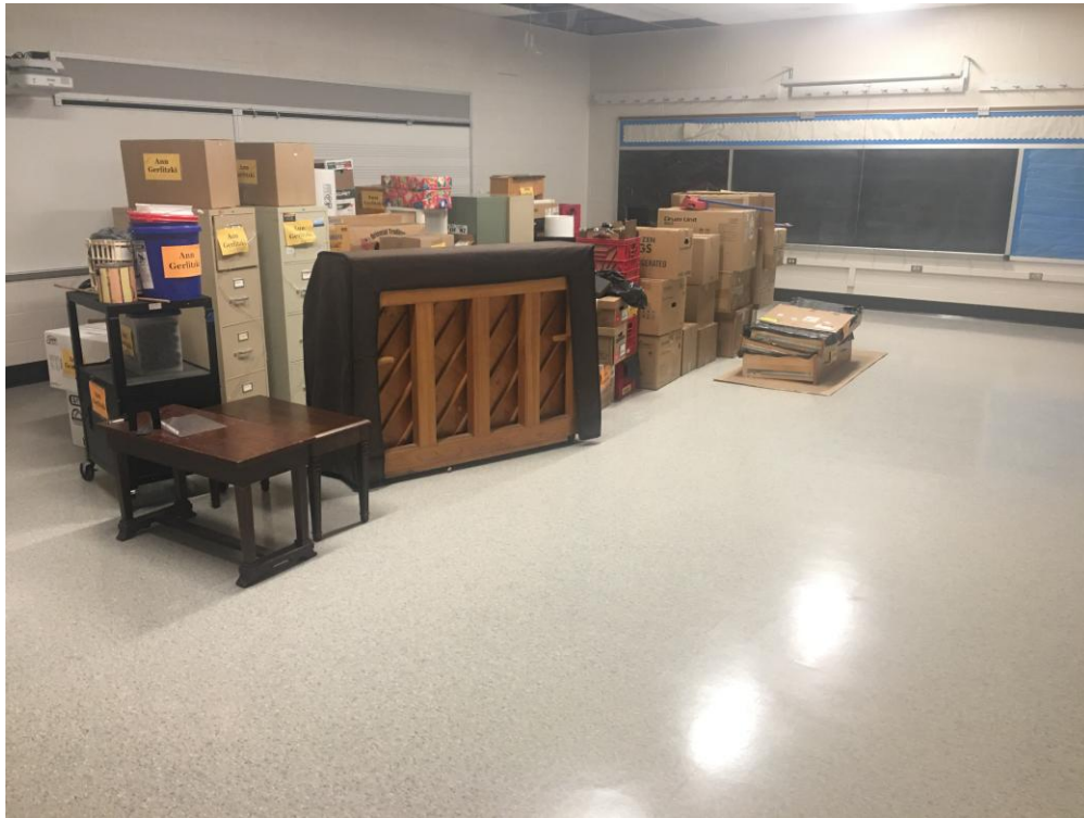
View of renovated Music Classroom.
