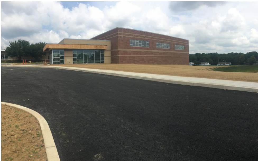
View of South side of new Gym addition.
