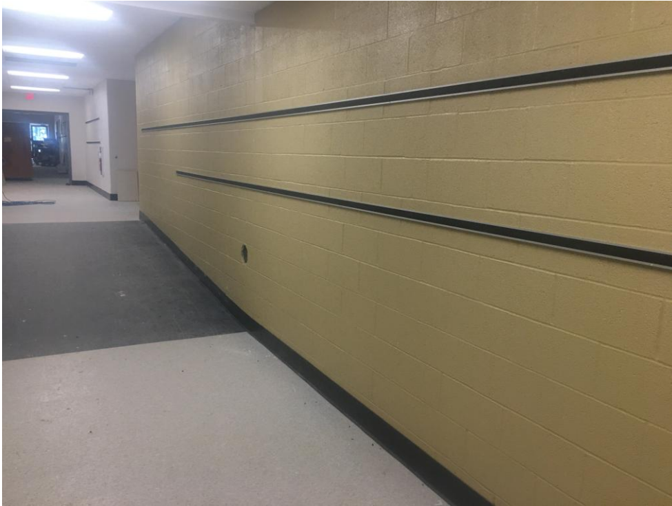
View of new tack strips in N corridor of new Classroom wing.
