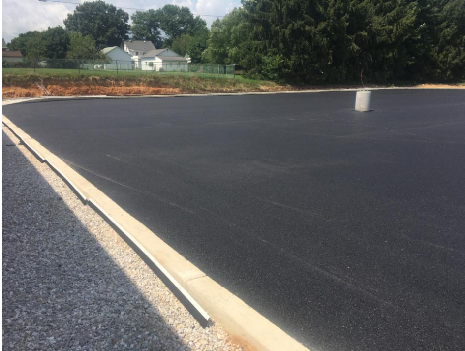
View of rear parking lot. Area where retaining wall goes is at upper left.
