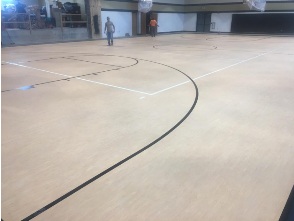
View of painted lines in Gym.
