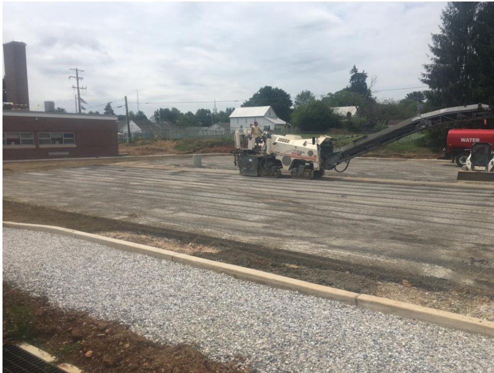
View of Rear Parking Lot being milled in preparation for paving.
