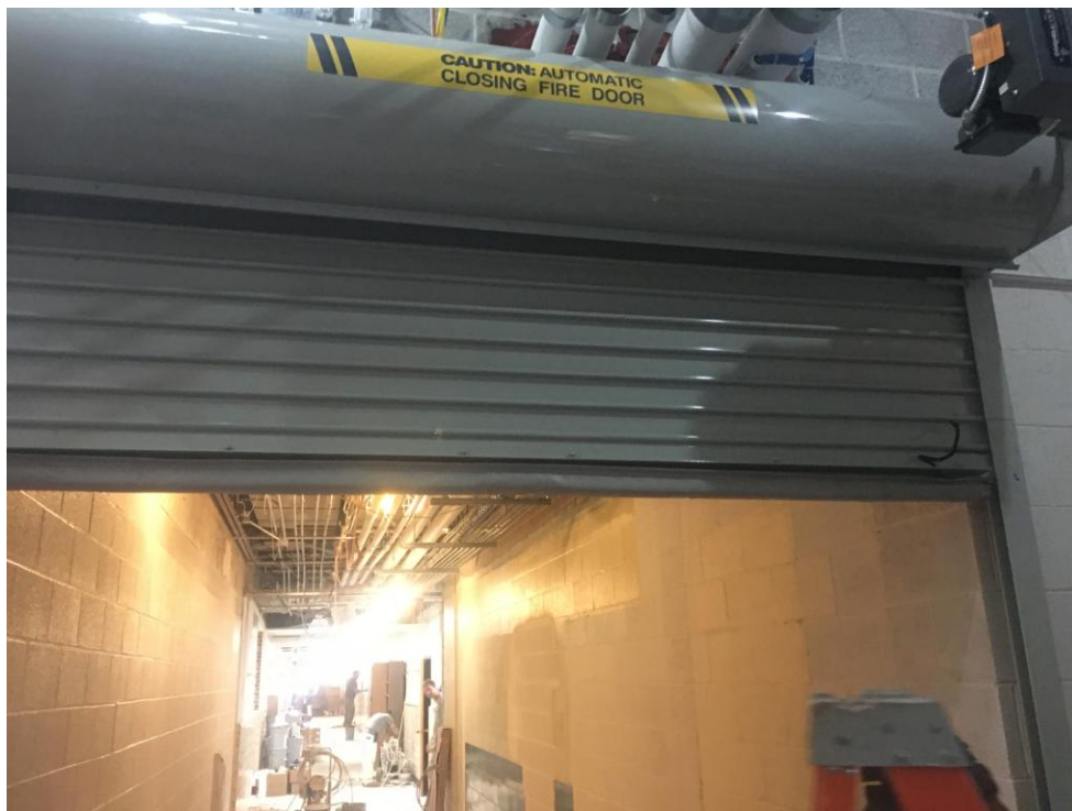
View of one of two fire doors separating the new construction from existing.
