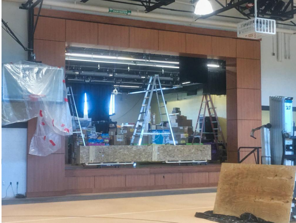
View of new Proscenium Wall.
